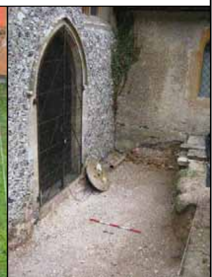
Extension area on completion of excavation
