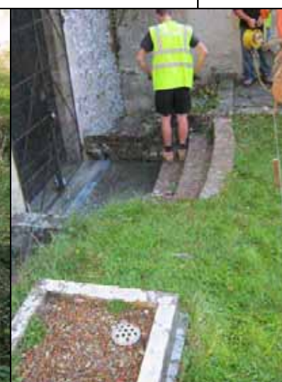
Extension area prior to excavation
