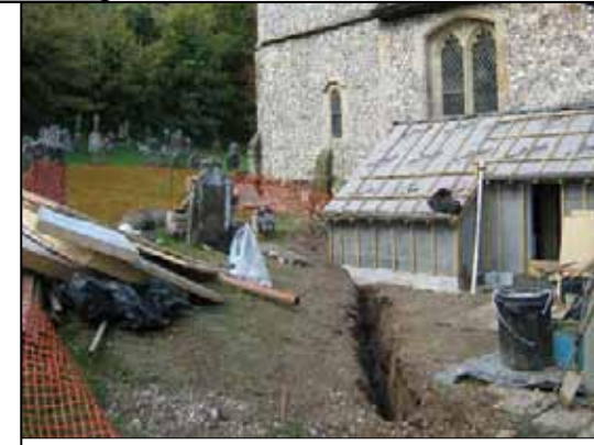
Western service trench and extension
