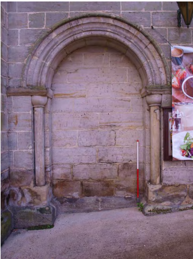
Plate 2: Left-hand blind arch prior to alteration (23)
