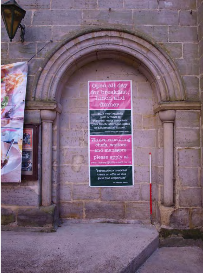
Plate 3: Right-hand blind arch prior to alteration (22)
