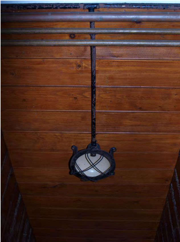
Plate 8: Cell light-fitting (16)
