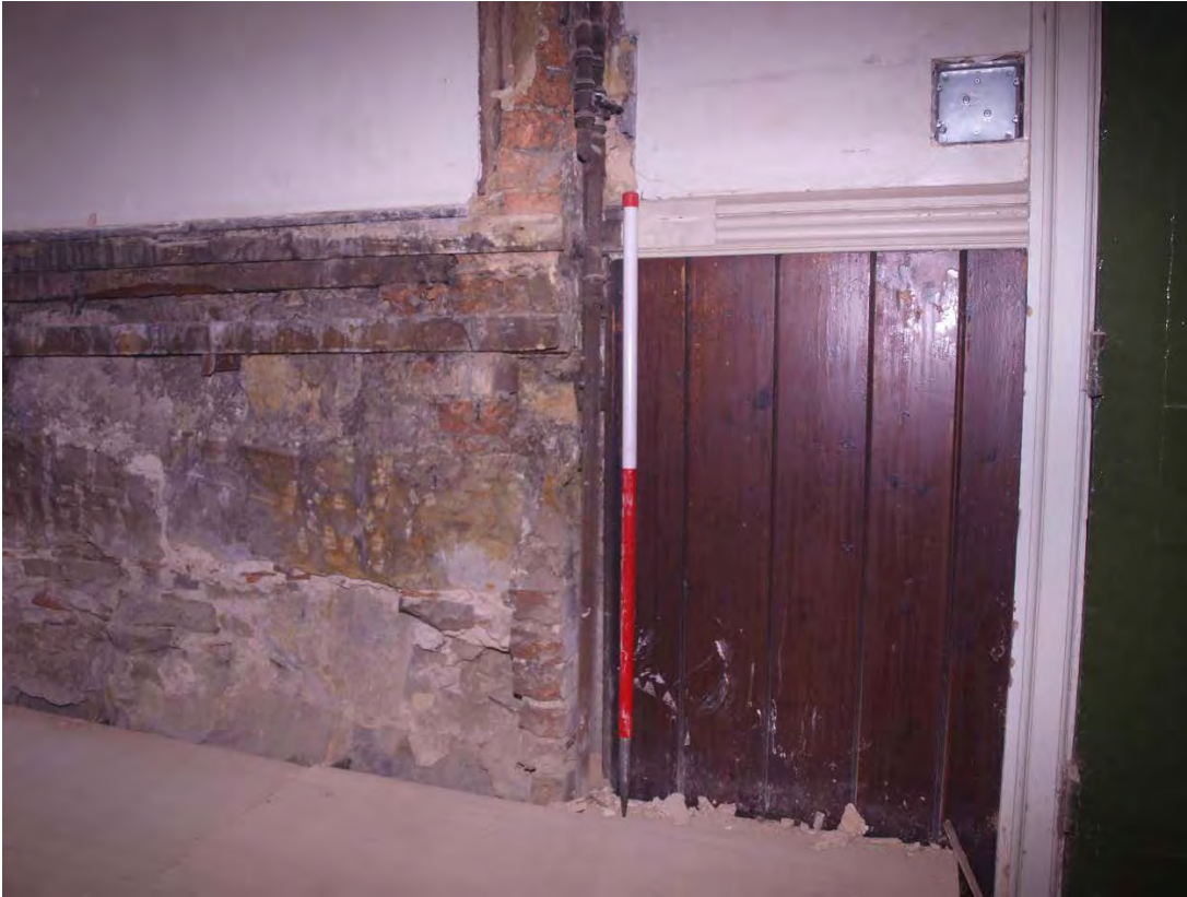
Plate 11: Tongue and groove boarded dado revealed on north wall, looking north (35)
