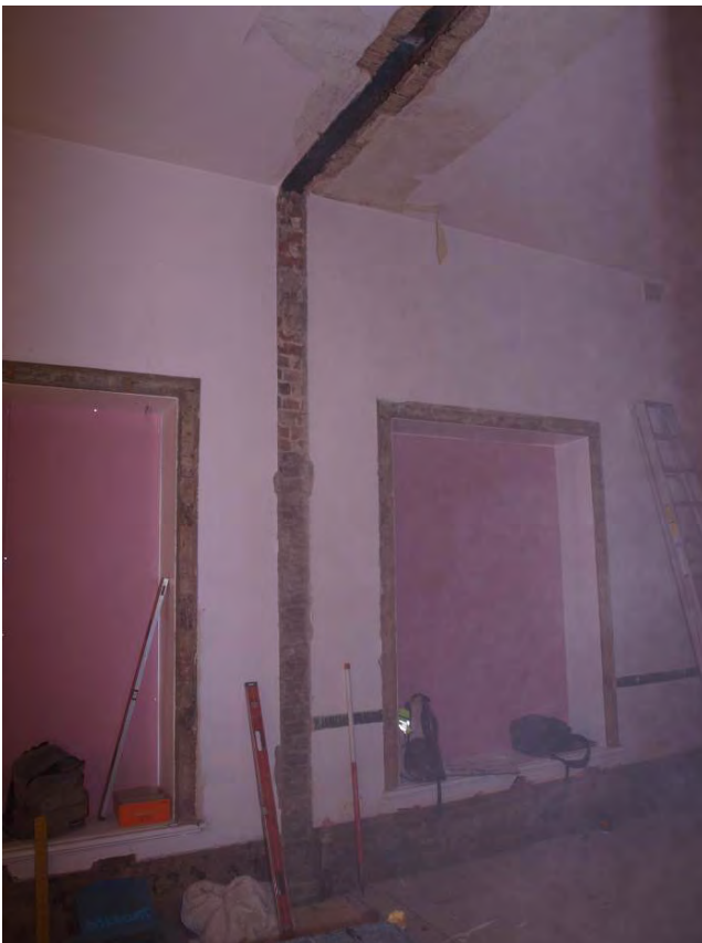
Plate 12: Rear ground floor room following removal of partition wall, looking south (46)
