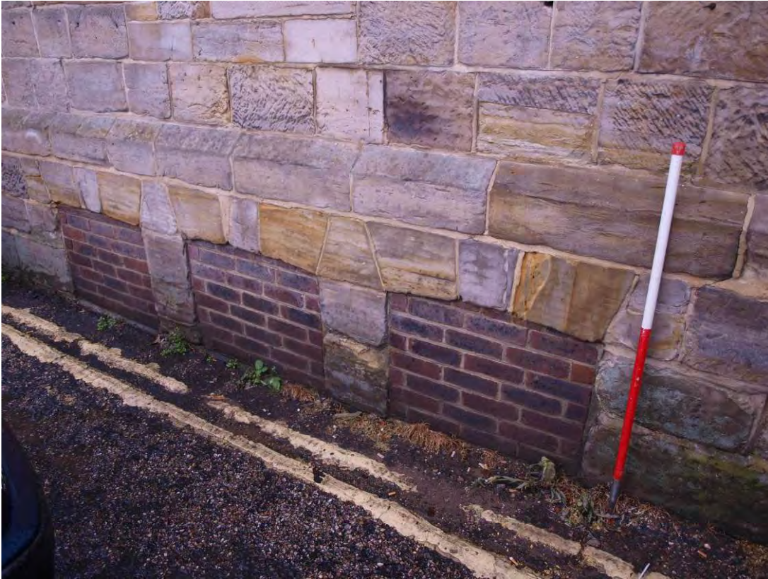
Plate 9: Blocked basement window apertures within south wall, looking north-west (24)
