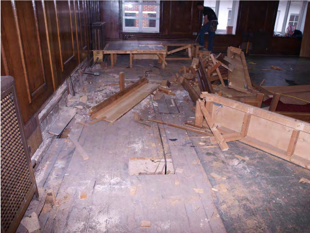
Plate 13: Removal of 1970s dais (first floor), looking east (26)
