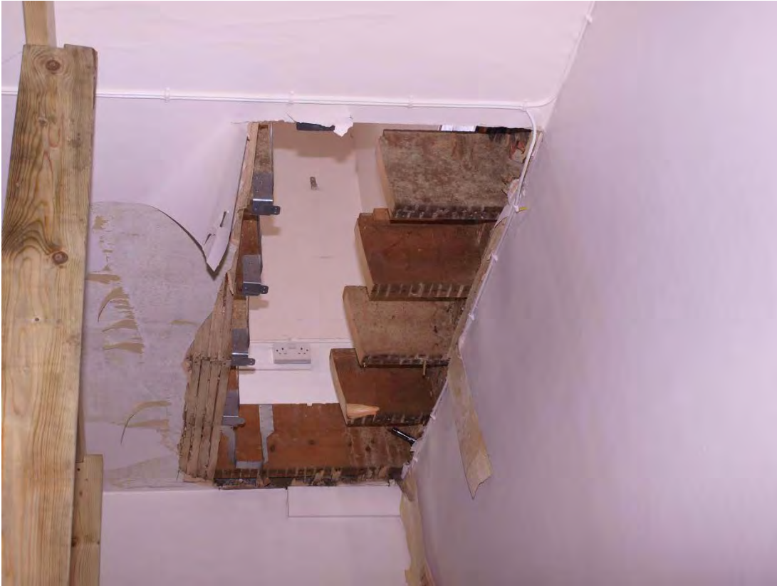
Plate 15: Creation of void in first floor for ducting, looking west (49)
