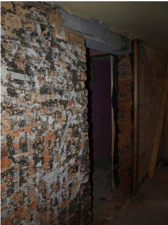
Plate 10: Doorway inserted within basement wall, looking south-east (51)
