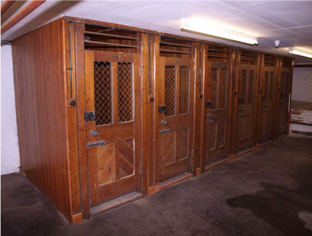
Plate 5: Cells in eastern portion of basement, looking north-west (18)
