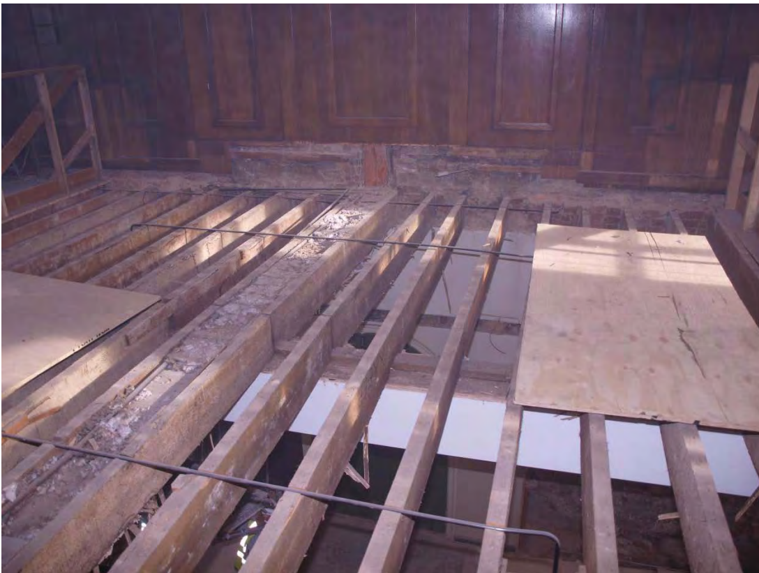
Plate 14: View during creation of first floor void, looking north (43)
