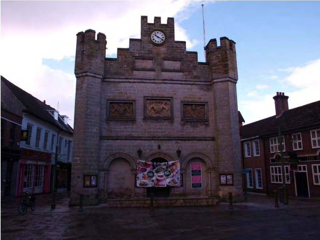
Plate 1: North elevation prior to alteration (21)
