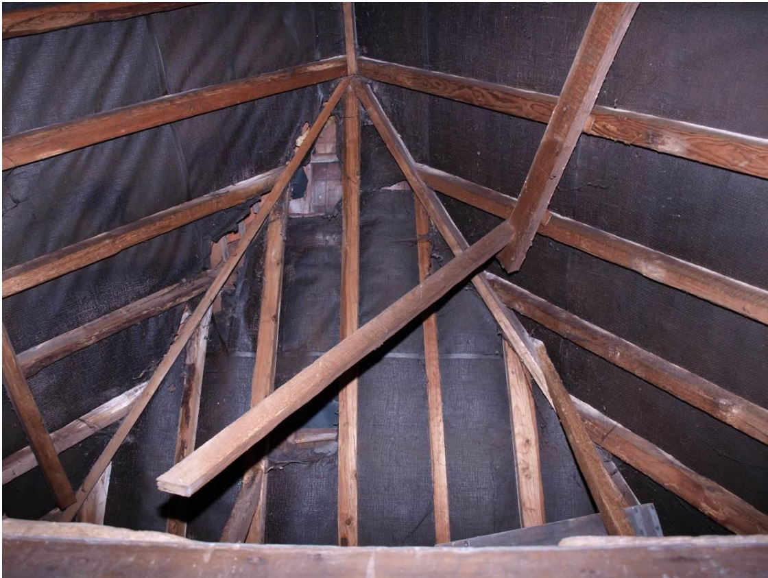
Plate 21: Roof structure visible over Room 8, looking west (37)
