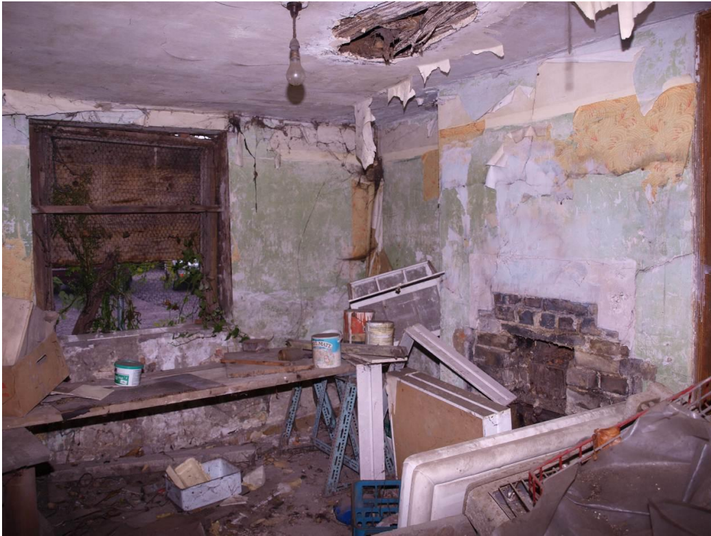
Plate 13: Room 4, looking south-west (28)
