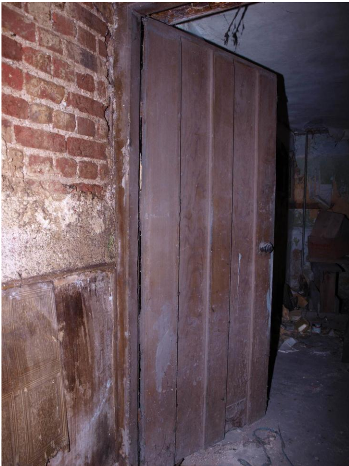
Plate 12: Door to Room 4, looking south-east (29)
