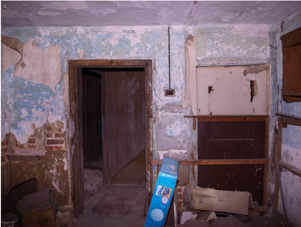
Plate 11: South wall of Room 3, looking south (23)
