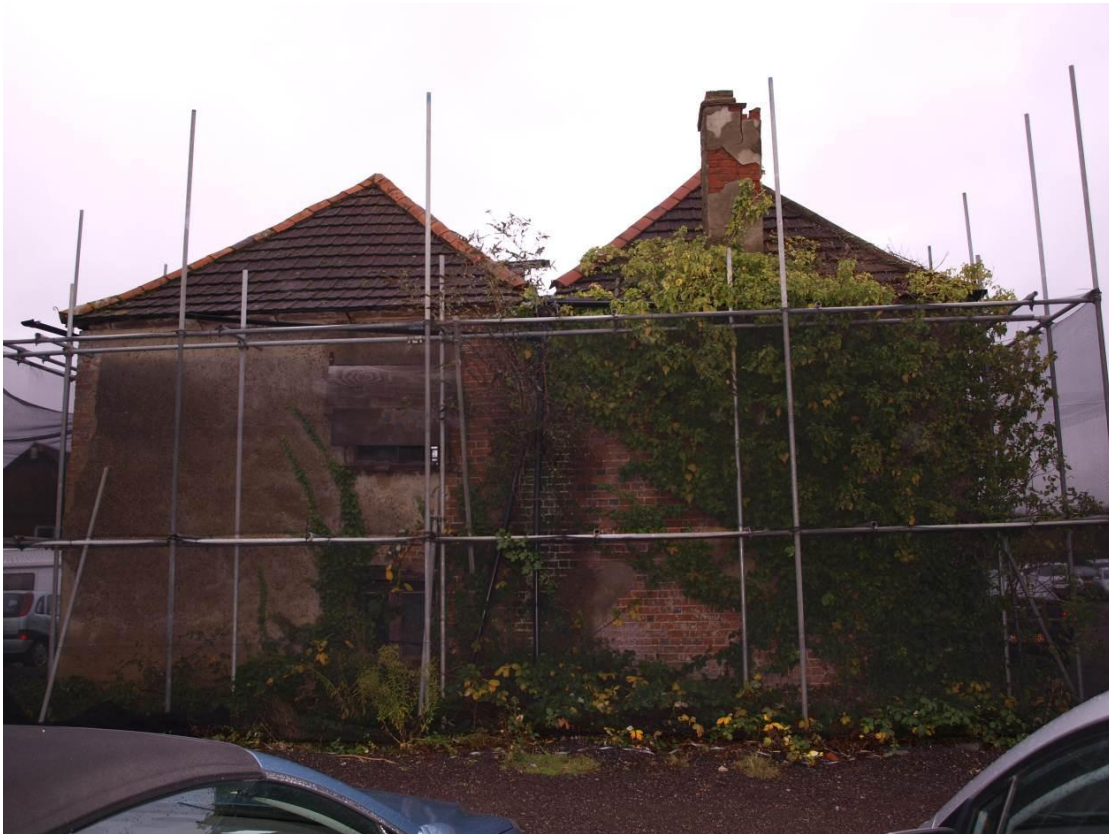
Plate 3: West elevation, looking east (3)
