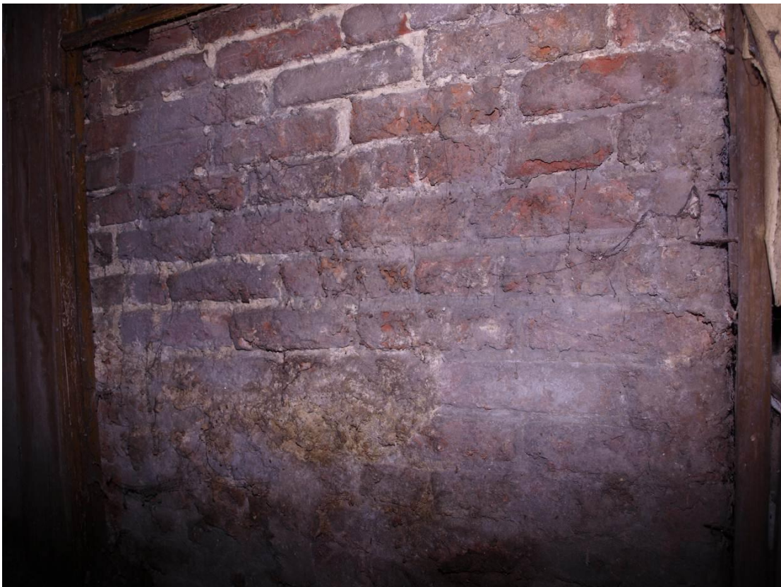
Plate 8: Earlier-looking brickwork on west side of chimney-stack, Room 2, looking east (21)
