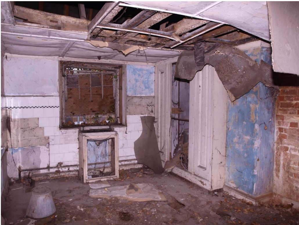
Plate 20: Room 8, looking north-west (36)
