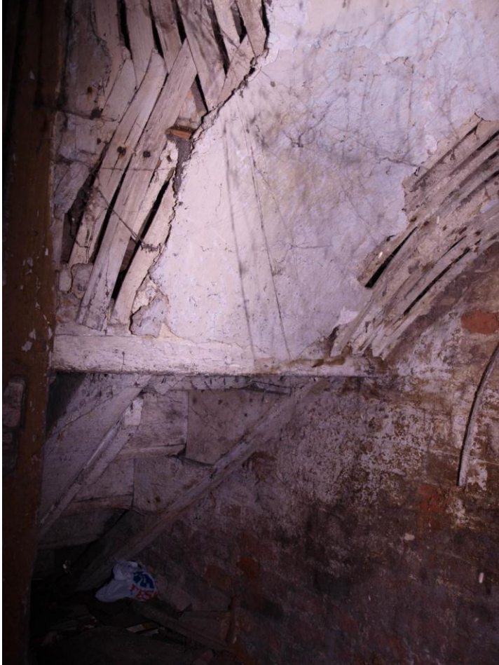
Plate 15: Under-side of staircase, looking east (26)
