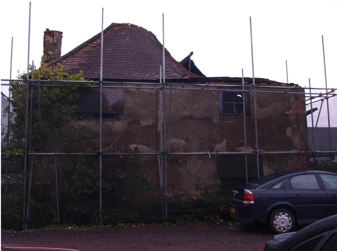
Plate 4: South elevation, looking north (6)
