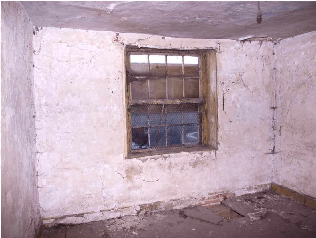
Plate 17: Room 5, looking north (33)
