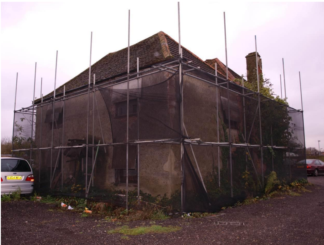
Plate 2: Principal (north) and west elevations, looking south-east (2)
