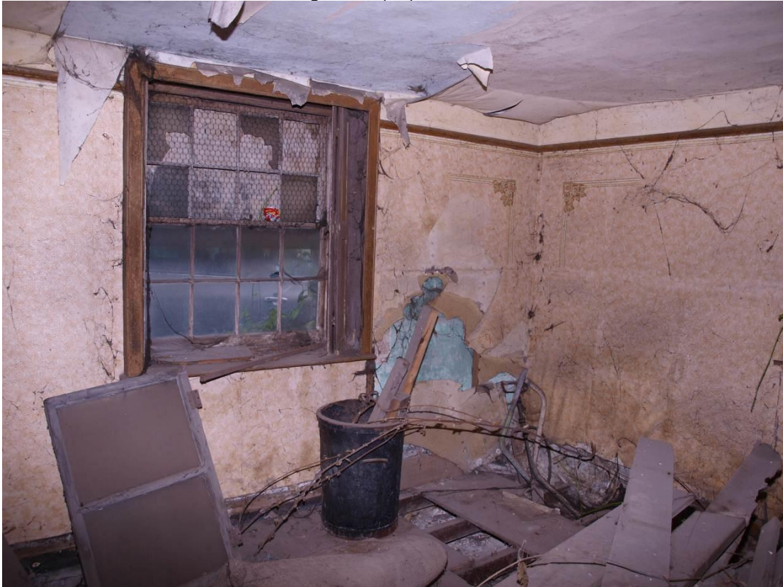
Plate 7: Room 1, looking north-east (15)
