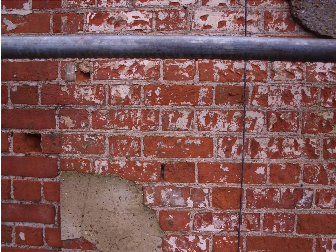
Plate 1: Penny-struck pointing to brickwork of east elevation, looking west (13)
