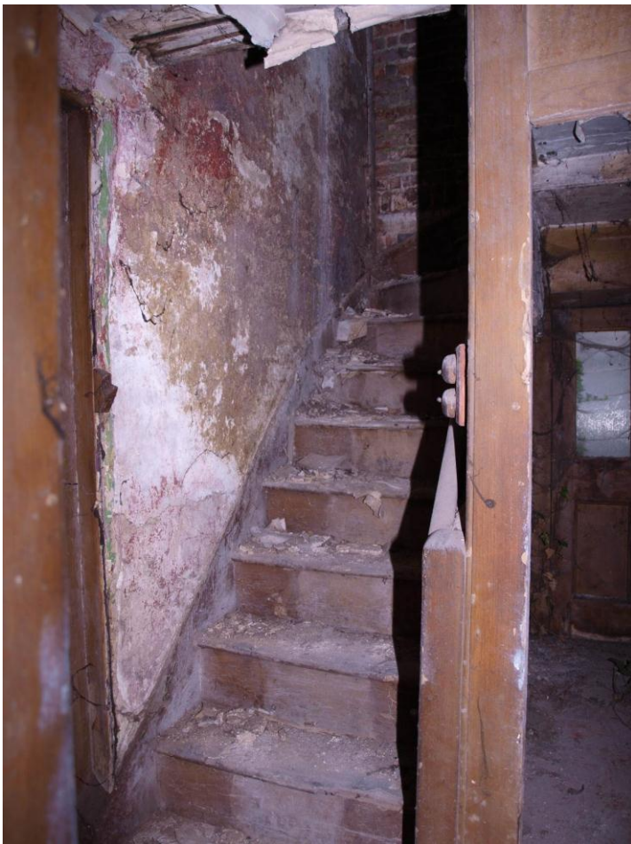
Plate 14: Staircase, looking west (27)
