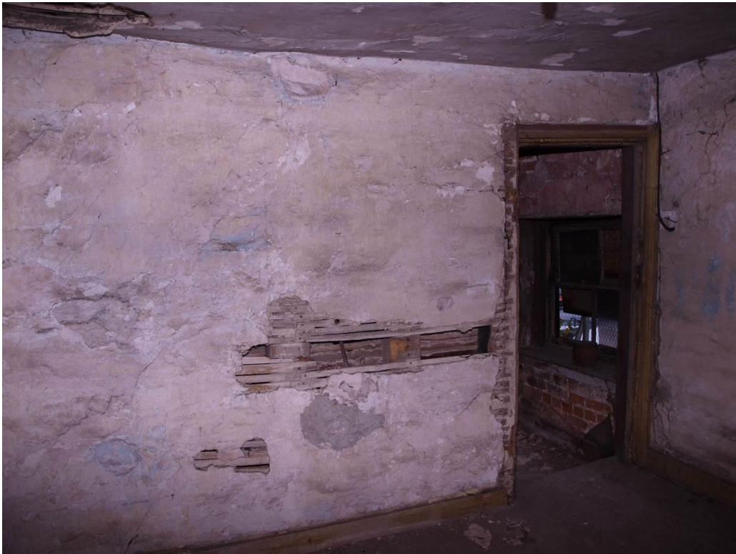
Plate 16: South wall of Room 5, looking south (34)
