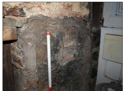
Plate 7: Detail of Elevation 6 showing sooting, filling material and brick-filled opening
