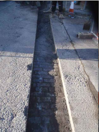
Fig. 3.1 Stone set cobble surface
