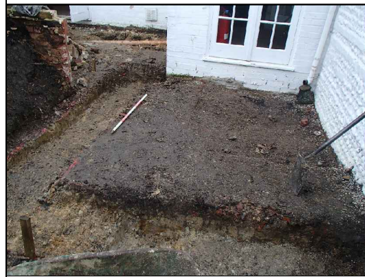
Monitored area, facing north-west
