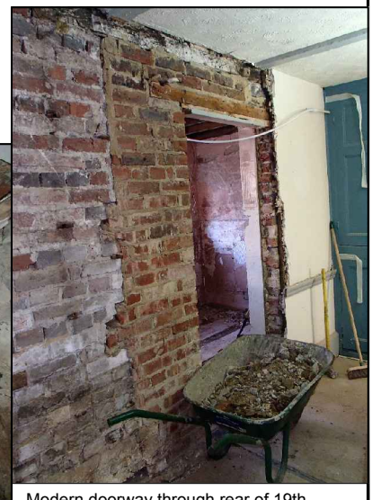
Modern doorway through rear of 19th Century range
