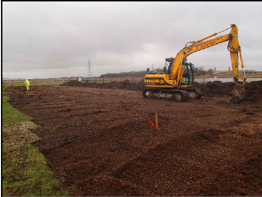
Topsoil strip, looking north-west
