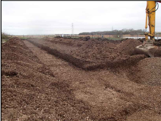
Trenches down to natural, looking north-west
