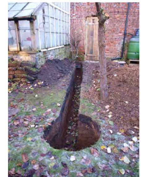
Service trench 1, looking north
