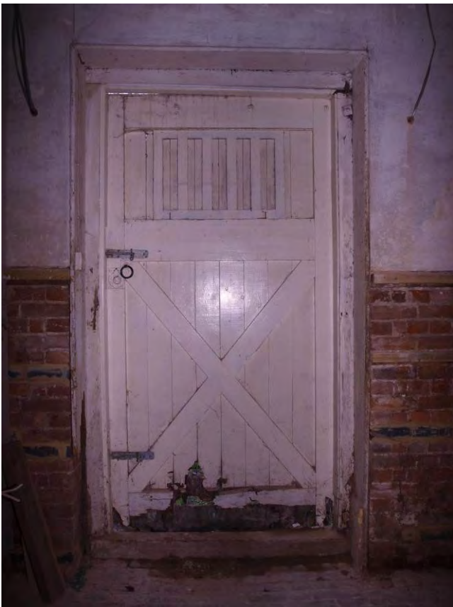
Plate 16: Interior face of entrance door on north elevation, looking north (28)
