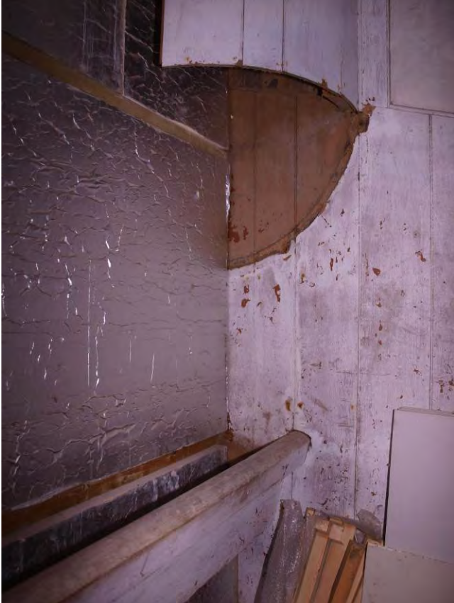
Plate 15: Manger and pitching hole in Room 2, looking south-west (25)
