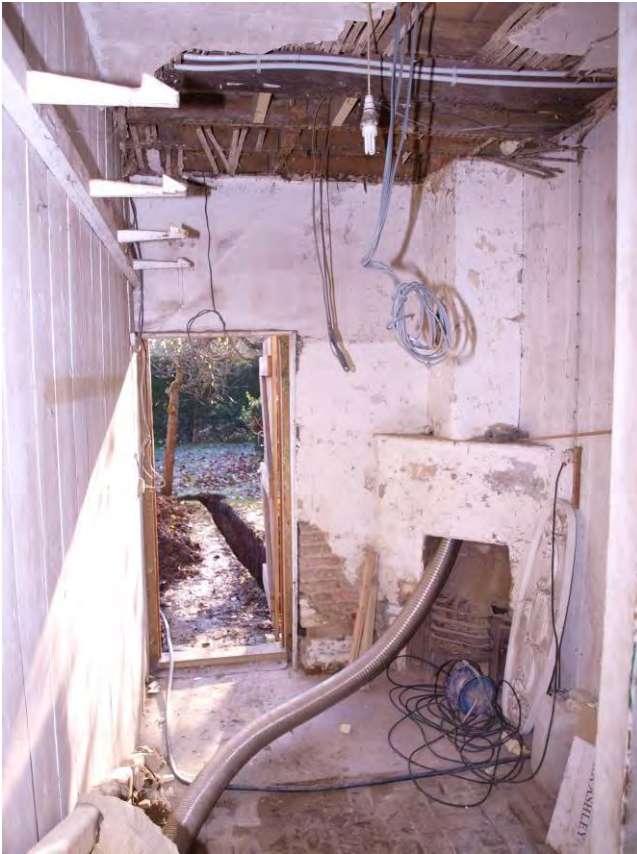
Plate 19: Tack room (Room 3), looking south (33)
