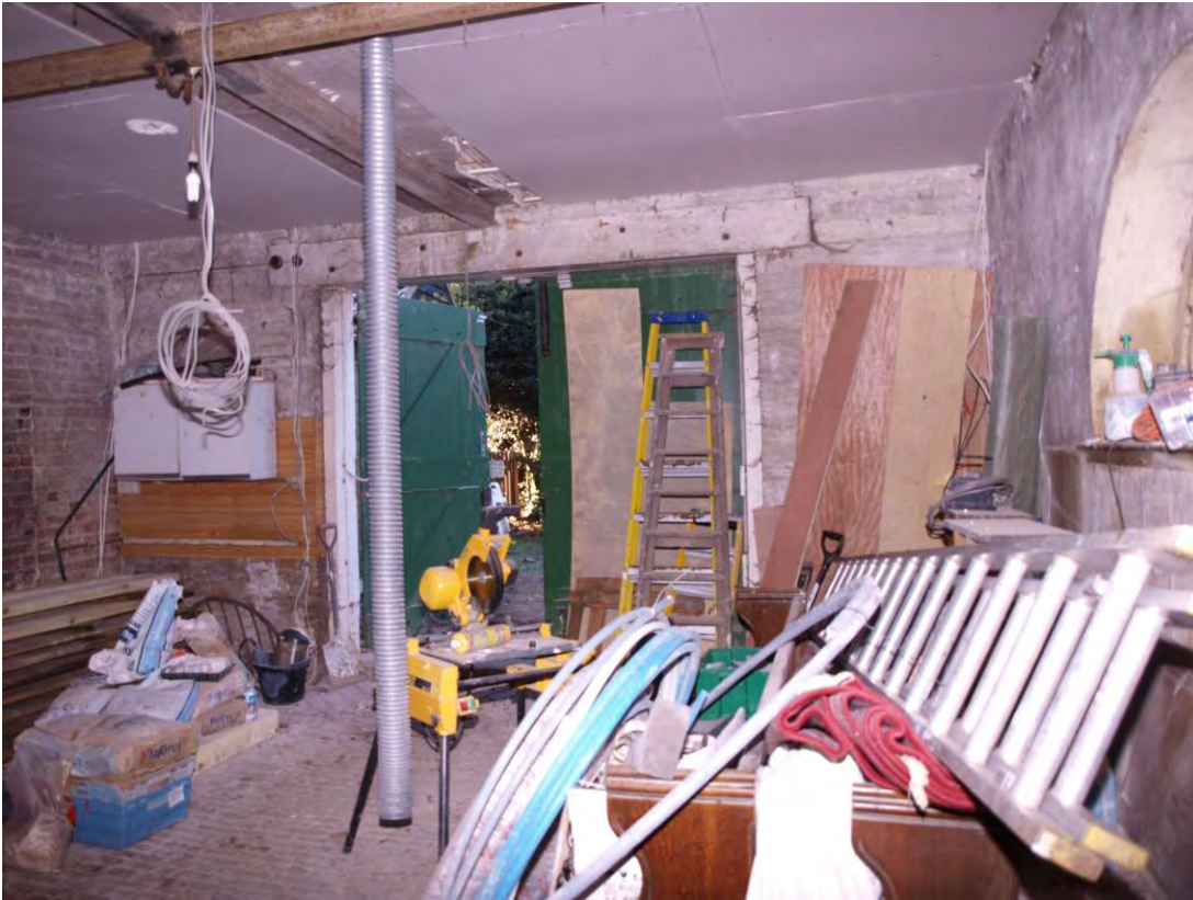
Plate 11: West wall of Room 1, showing wide doorway, looking west (16)
