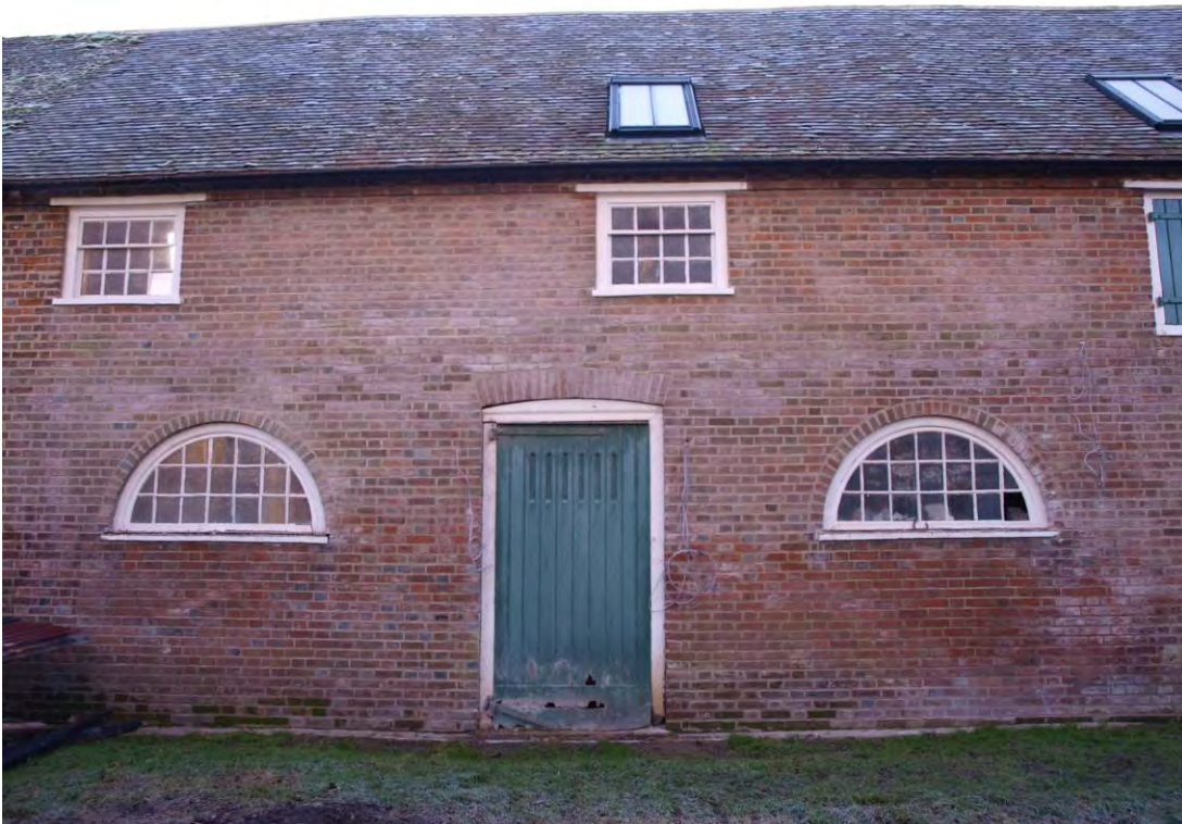
Plate 2: Principal doorway with flanking semi-circular windows on north elevation, looking south (4)
