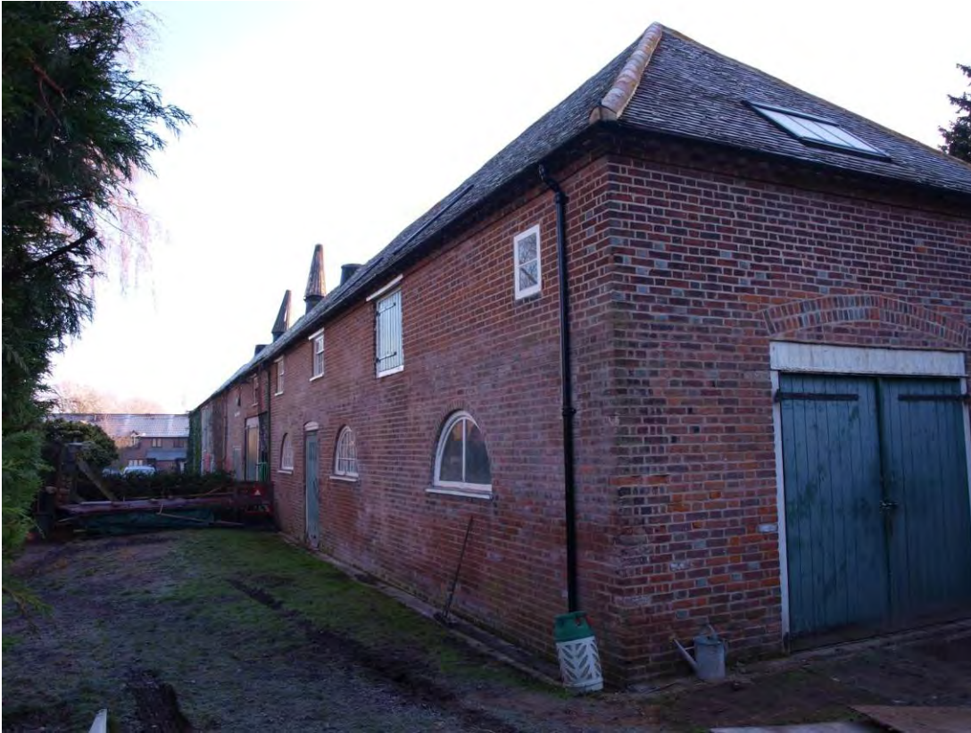
Plate 1: North and west elevations, looking south-west (2)
