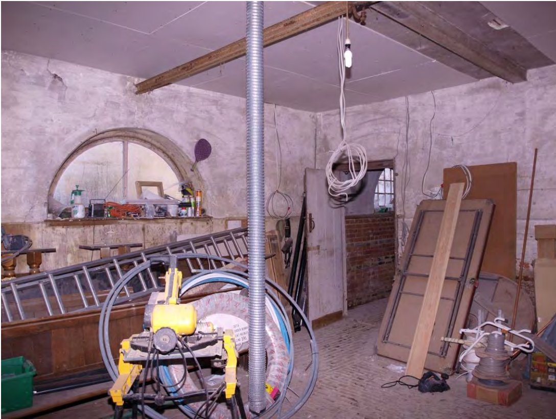
Plate 9: North and east walls of Room 1, showing boarded dado and semi-circular window (N) and boarded door (E), looking north-east (17)
