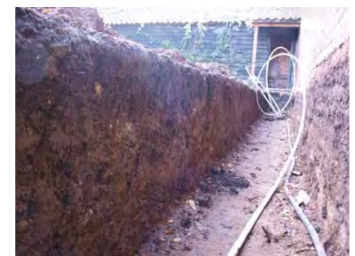
North-facing section of service trench 3, looking west
