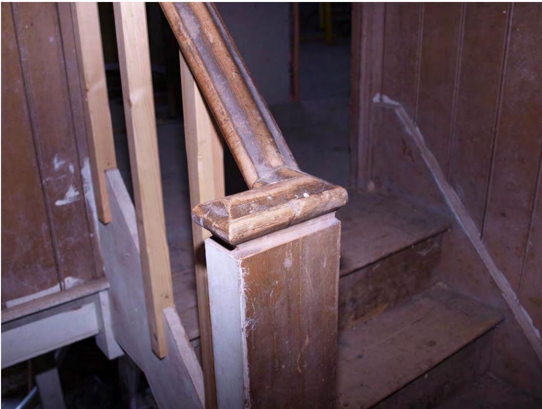
Plate 20: Staircase detail, looking south-west (52)
