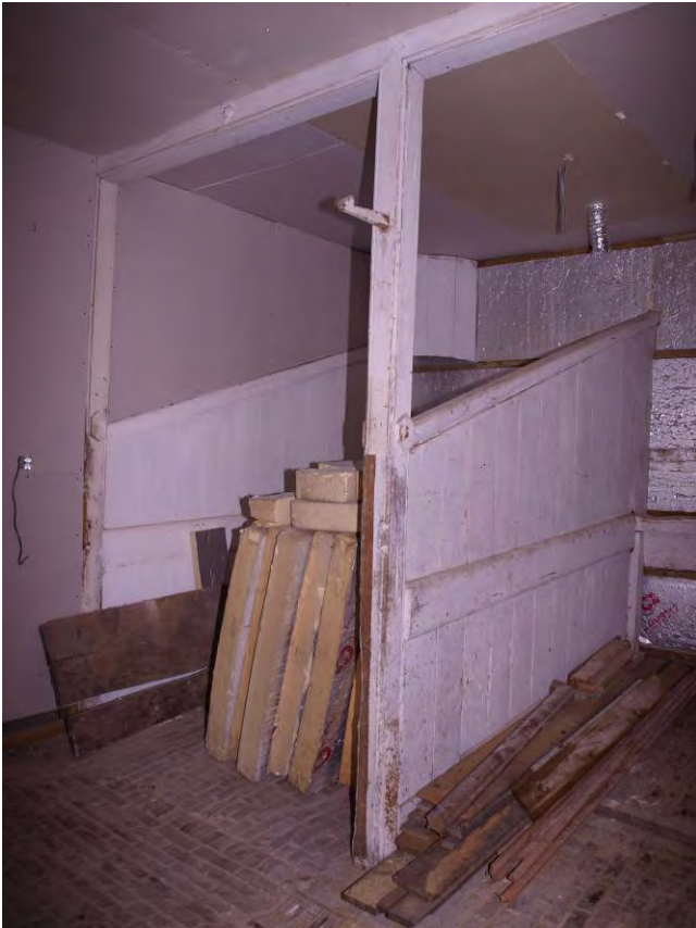
Plate 13: Stall partitions within Room 2, looking south-east (23)
