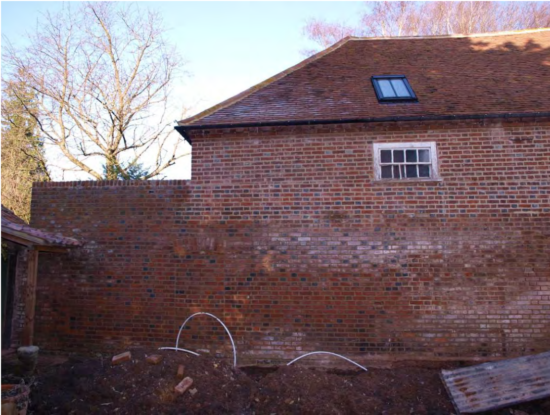
Plate 5: South wall of the building, constructed over pre-existing garden wall, looking north (9)
