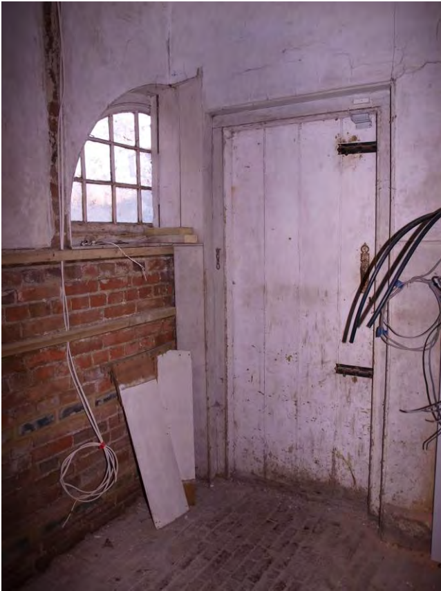
Plate 17: Door between Rooms 2 & 3, looking north-east (29)
