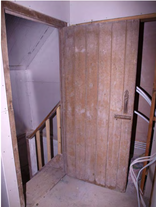
Plate 21: Door to staircase, looking north-east (45)
