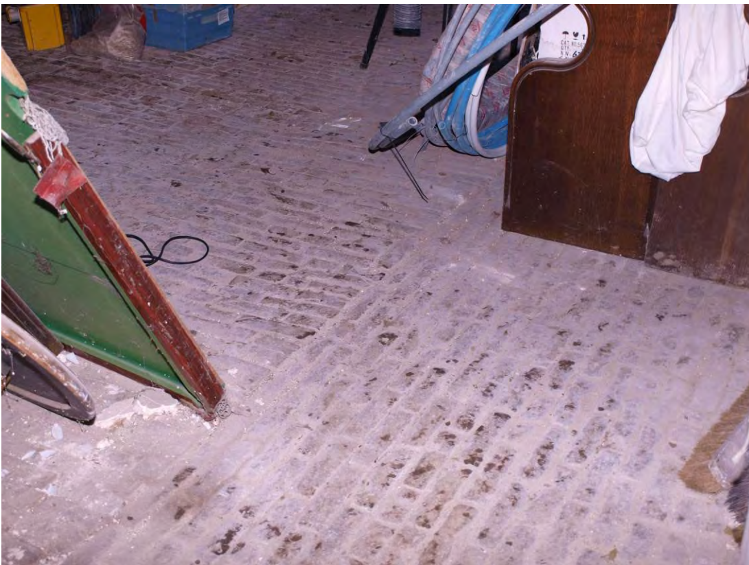
Brick floor within Room 1, looking south-west (22)
