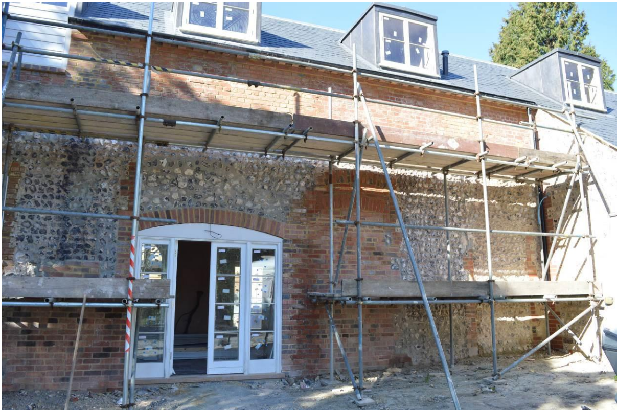
Plate 4.11: Brick quoins indicate former doorway to north-east elevation, blocked with coursed flintwork (right-hand side of photo) (59)
