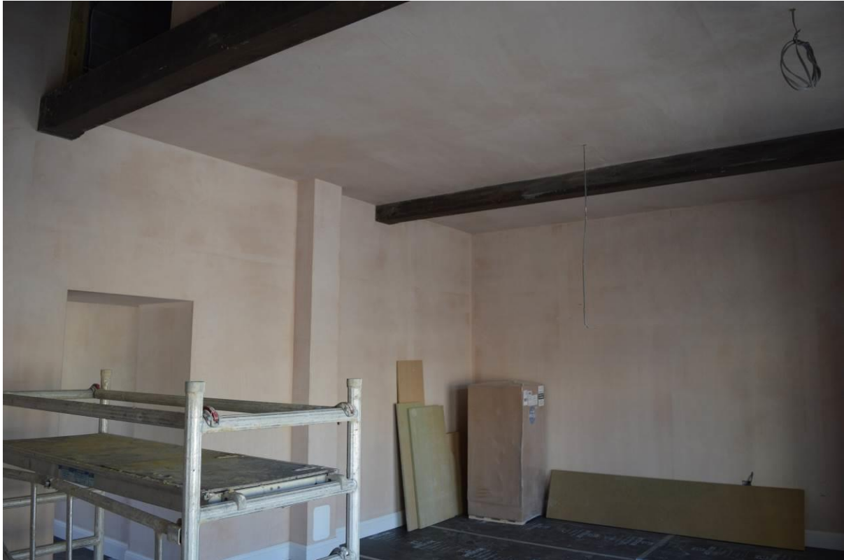
Plate 4.9: Ground floor (Room 17), looking east (60)
