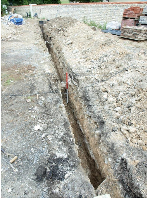
Plate 5.1: Drainage run, southern corner of courtyard, looking east.
