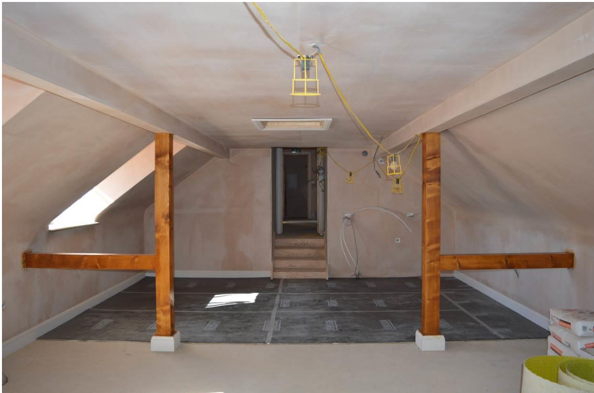
Plate 4.10: First floor of north-eastern half of central range, looking south-west (67)
