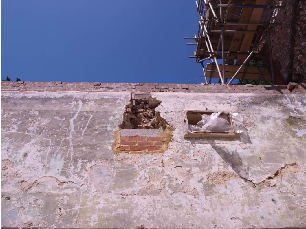
Plate 4.3: Possible vent on north-west wall of Room 1 (36).
