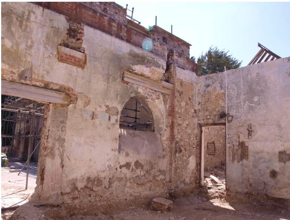
Plate 4.2: Room 1, looking towards south corner (35).
