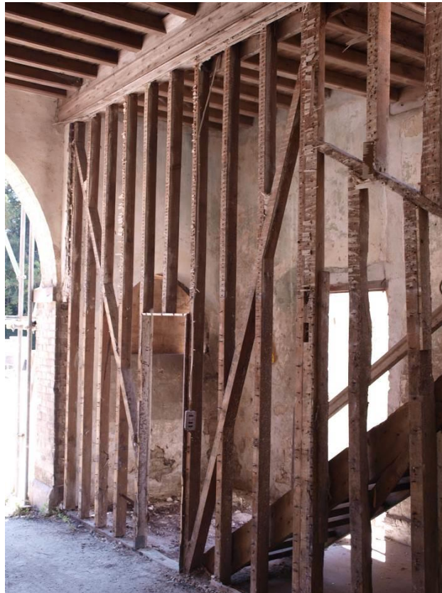
Plate 4.1: Primary braced partition on south-western side of entrance way (43)
