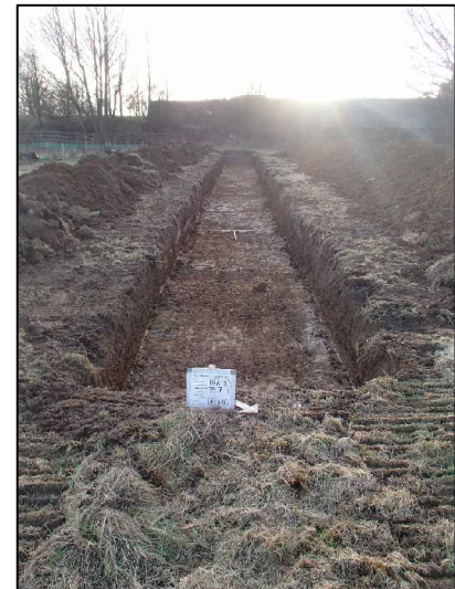
Trench 7, facing South-west
