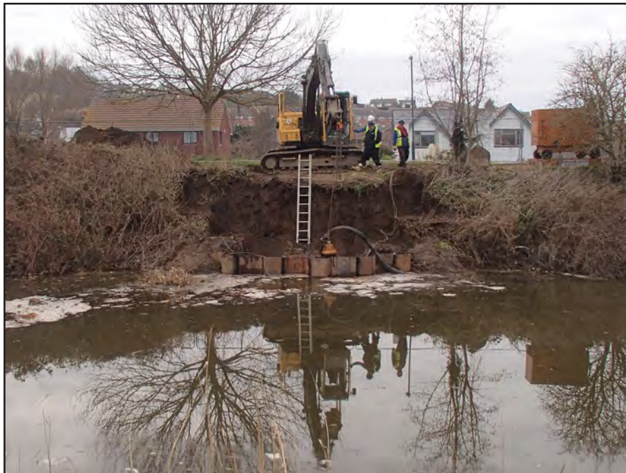
View of monitored groundworks looking north.
