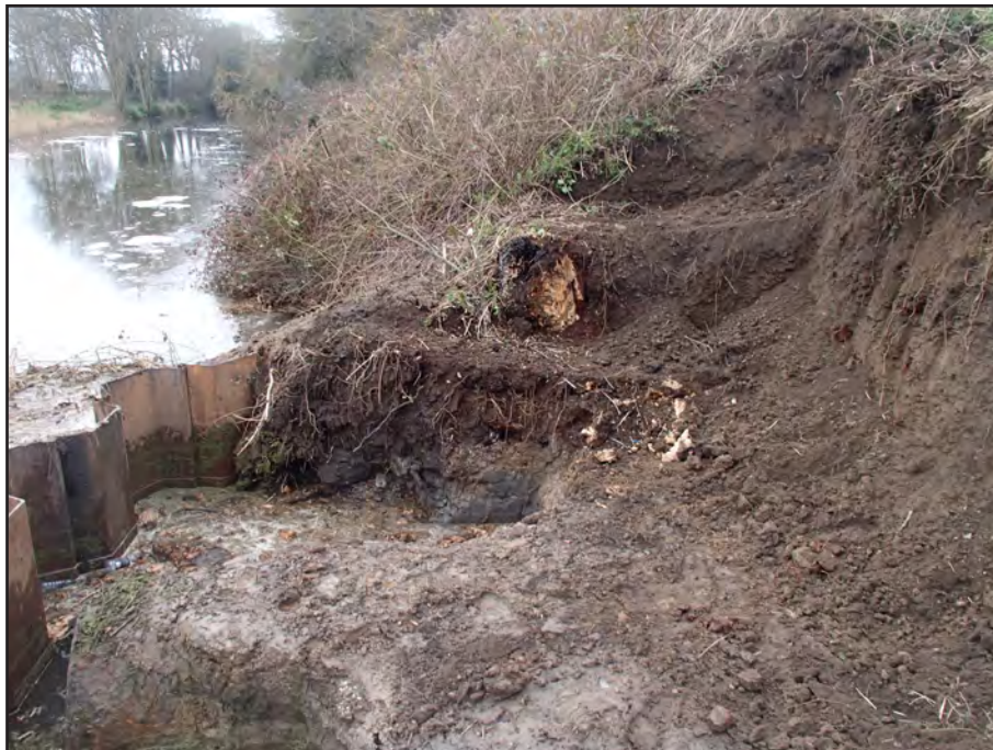
East facing section of monitored area during excavation.
