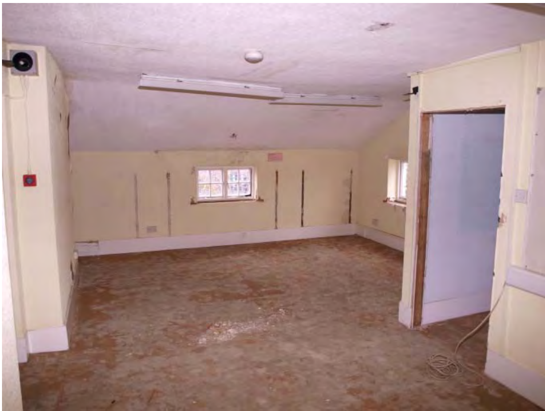
Plate 18 Room 8, looking south-west (27)
