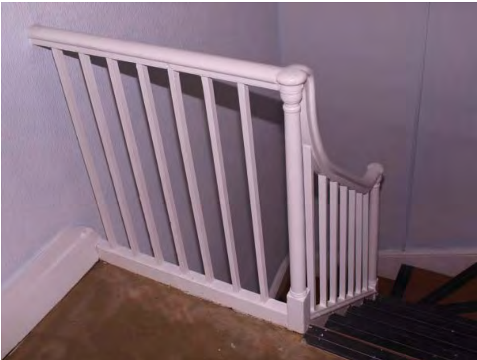
Plate 10 Staircase as seen from second floor landing (Room 7), looking north-west (25)
