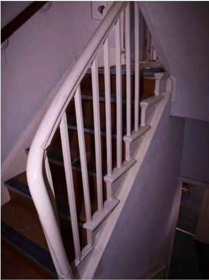
Plate 9 Ground to first floor flight of staircase, looking south-east (16)
