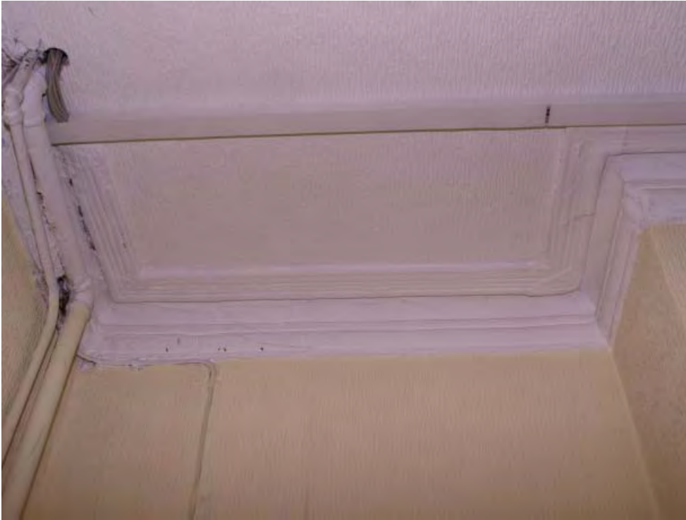
Plate 13 Cornice in Room 3 (14)
