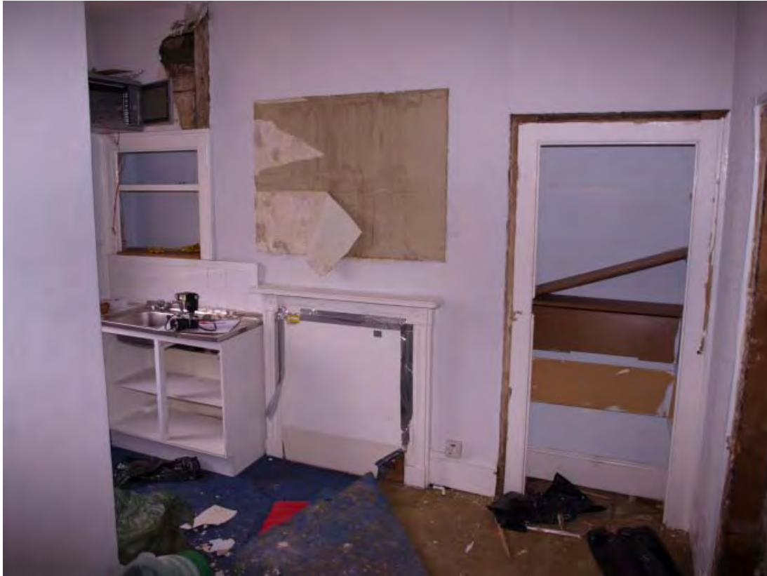
Plate 17 Room 6, looking north-east (24)
