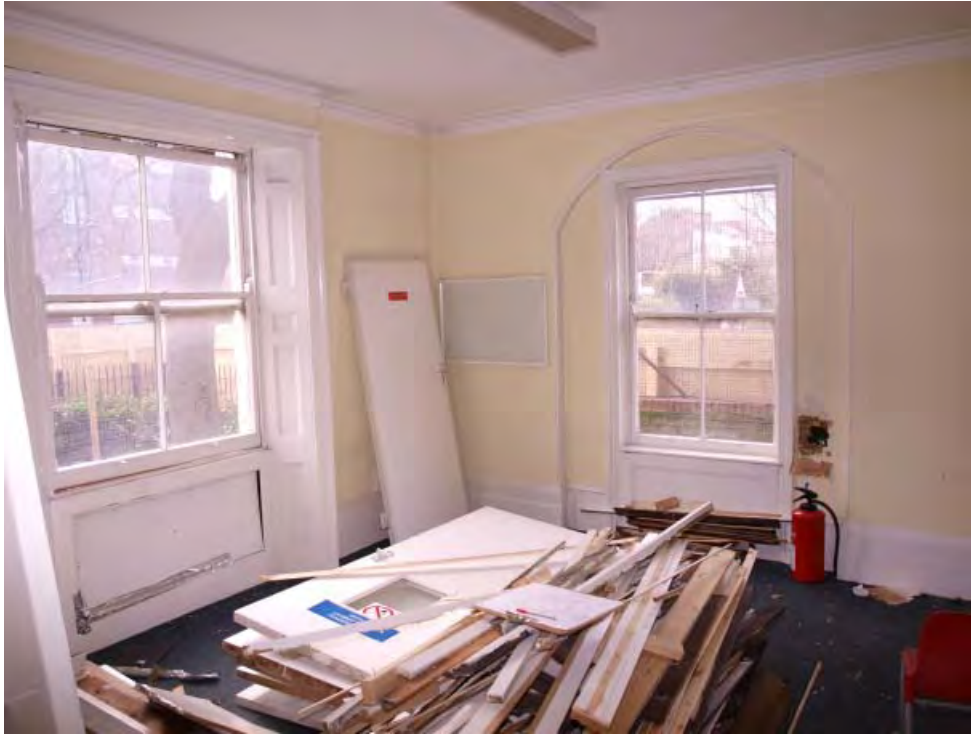
Plate 11 Room 2, looking south-west (8)
