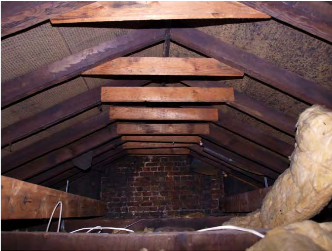
Plate 19 Roof, looking east (28)
