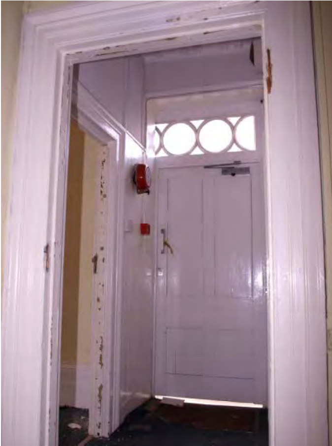
Plate 7 Entrance hall (Room 1) showing partition wall bisecting main entrance, looking west (6)
