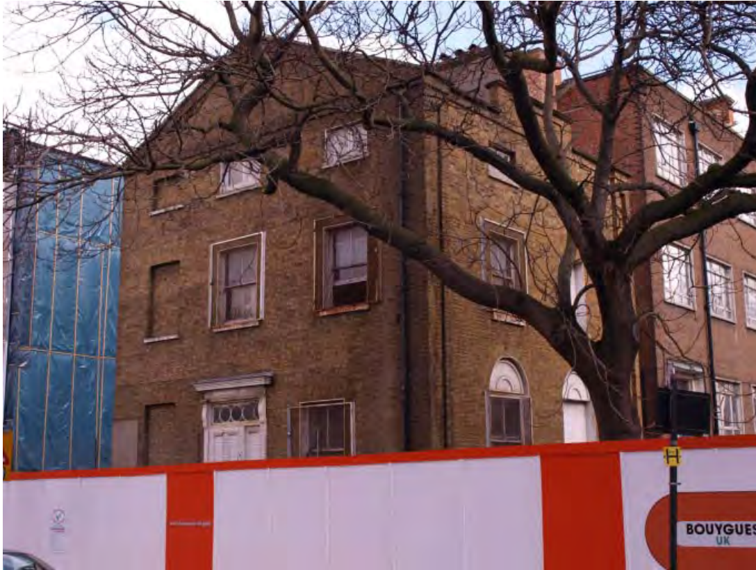
Plate 1 West and south elevations of the building, looking north-east (1)
