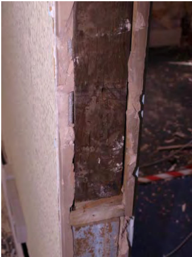
Plate 16 Stud exposed on west side of inserted doorway between Rooms 5 and 6. Shows small section of a Baltic merchant's mark (top) and truncated brace (covered by modern timber) (22)
