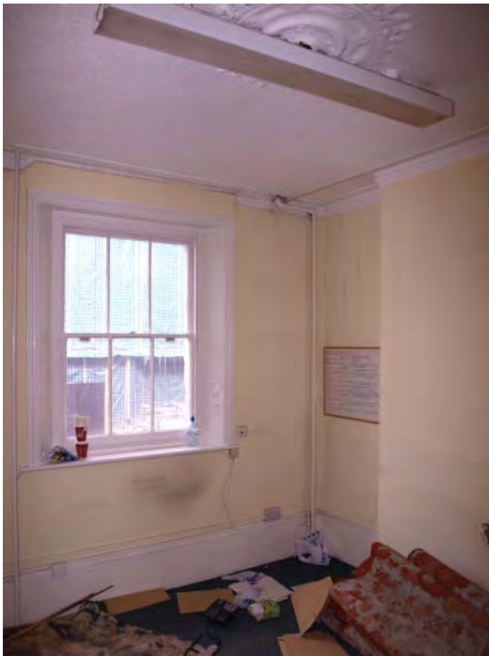
Plate 12 Room 3, looking north-east (12)
