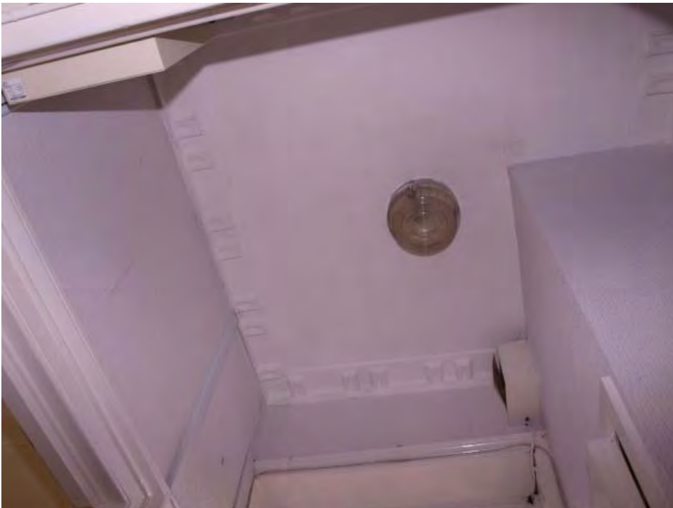
Plate 8 Cornice in Room 1 (7)
