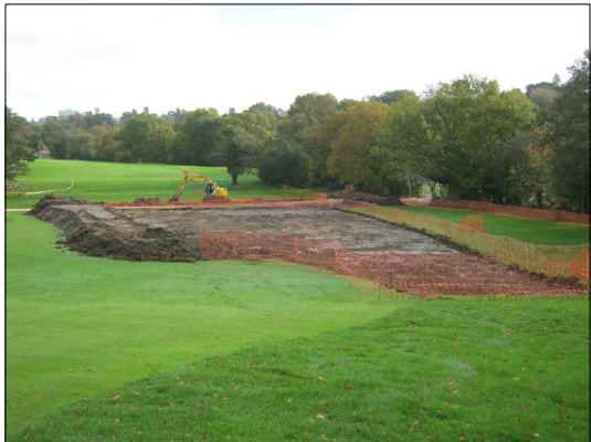
Embankment, facing east
