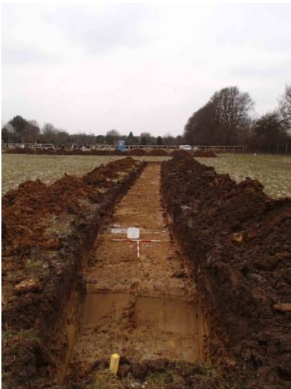
Trench 2 looking west
