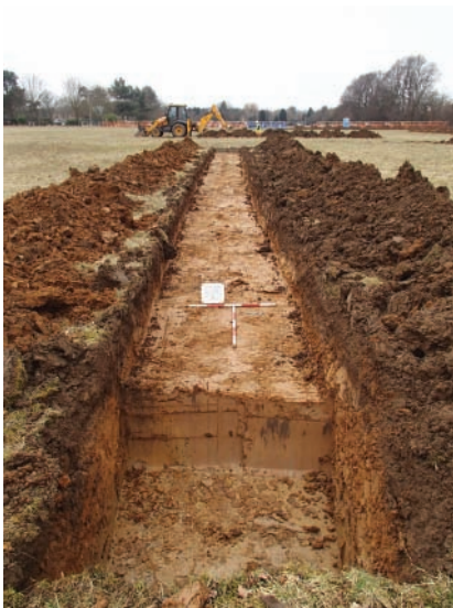
Trench 6 looking west
