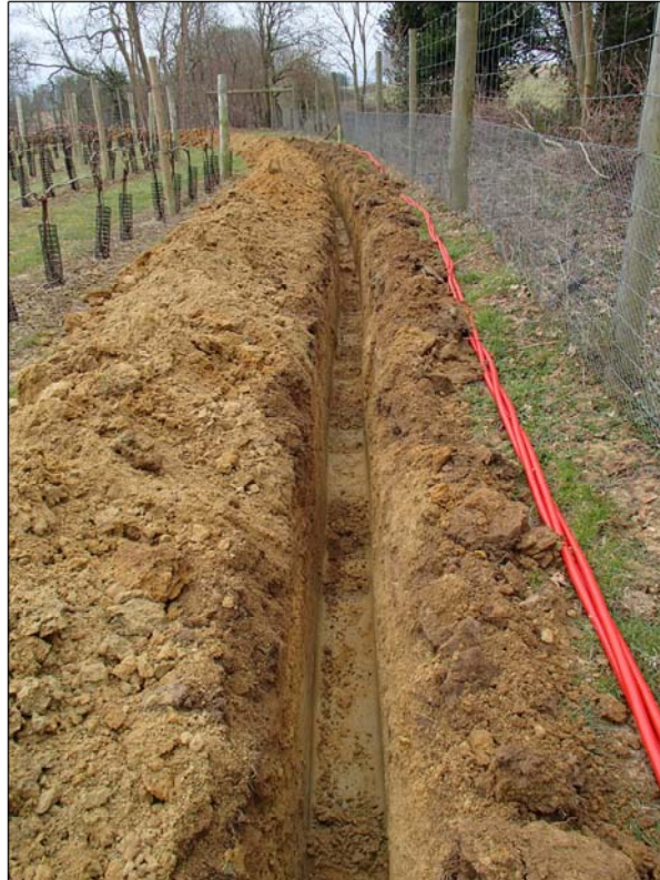
Fig. 3.a Underground HV Route Facing South
