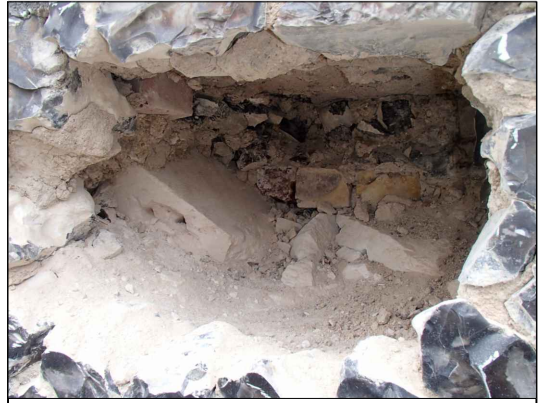
Close-up of test hole in northern transept wall
