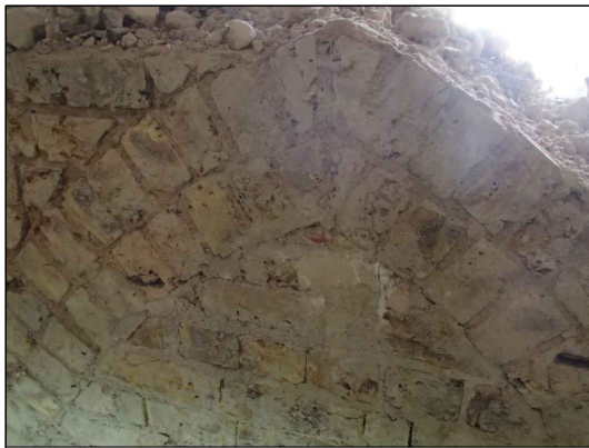
Brick arch door head (from internal wall face looking north)
