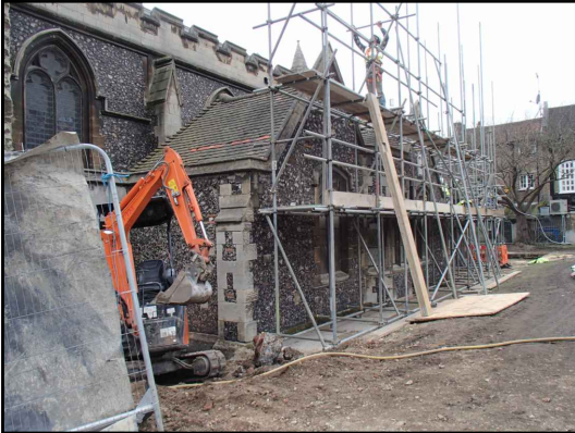
Scaffolding around choir vestry
