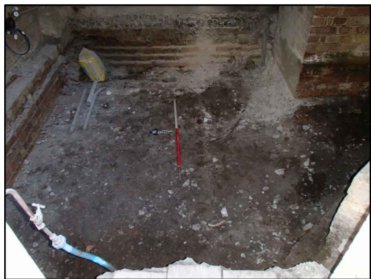
Reduced level in vestry room
