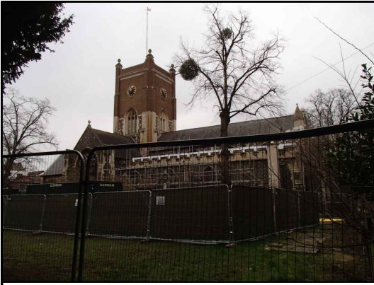
Screened fencing around church
