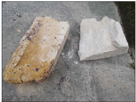
Brick and reused stone in core of northern transept wall
