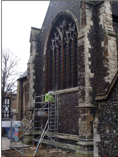
North transept - test hole in wall
