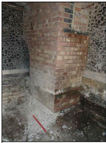
Original buttress in vestry room
