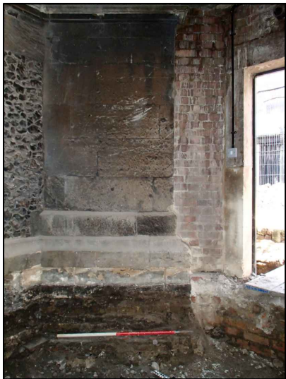
Chimney in vestry room
