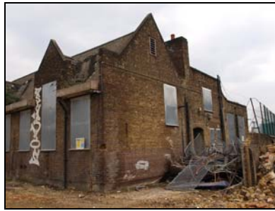
5852-017 (1/17) South elevation, oblique view. Facing east-northeast
