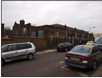
5852-026 (1/26) East and south elevations, oblique view. Facing northwest
