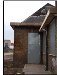
5852-030 (1/30) East elevation, south face of central block. Facing north
