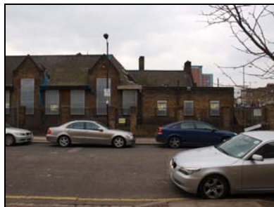
5852-023 (1/23) East elevation (northern section). Facing west
