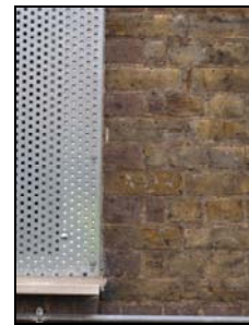
5852-021 (1/21) East elevation, detail of brickwork. Facing west
