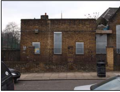
5852-025 (1/25) East elevation (southern section). Facing west
