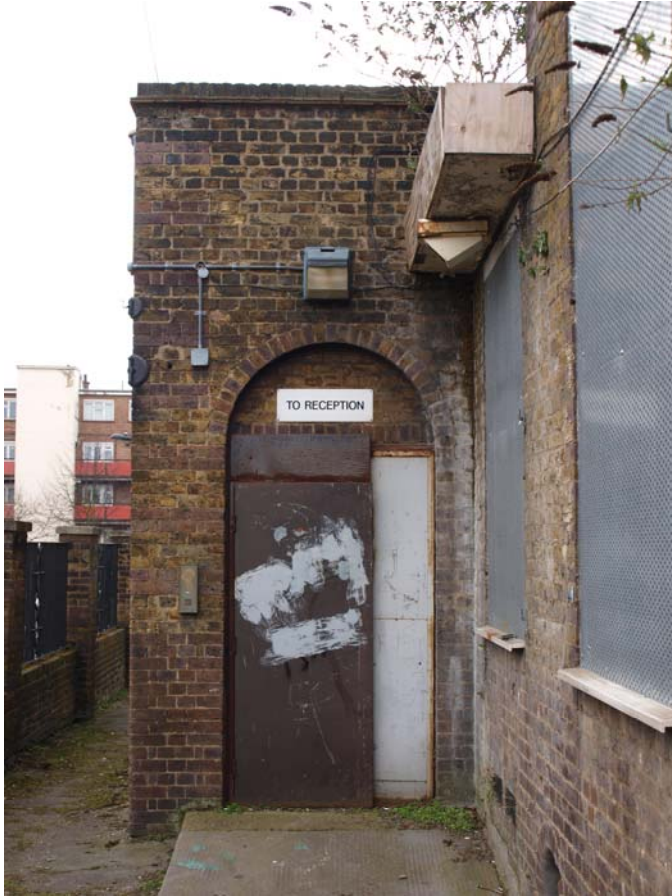
Plate 11. East elevation, north face of southern block. Facing south.
