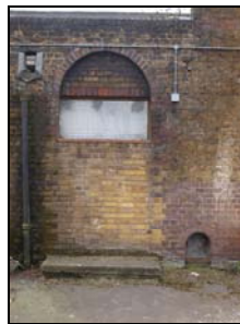
5852-011 (1/11) North elevation, blocked door and boot scraper. Facing south
