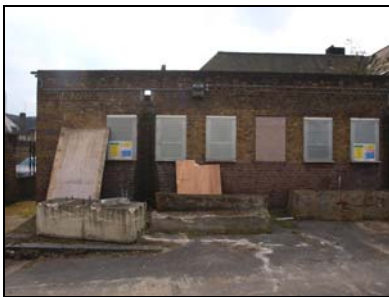
5852-010 (1/10) North elevation (eastern section). Facing south
