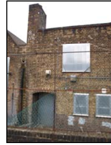
5852-015 (1/15) South elevation (central section). Facing north
