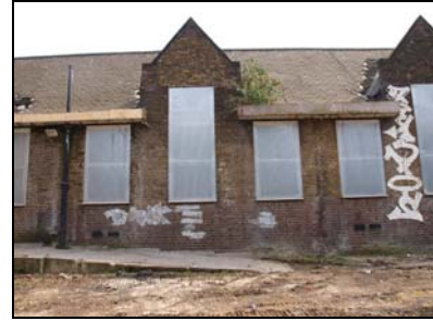
5852-003 (1/3) West elevation (northern wing). Facing east
