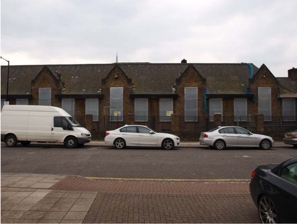
Plate 13. East elevation (central section). Facing west.
