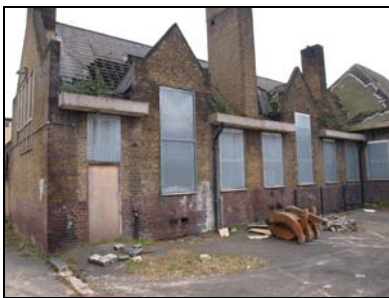
5852-004 (1/4) West elevation, oblique view. Facing southeast
