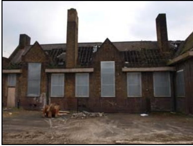
5852-001 (1/1) West elevation (southern wing). Facing east
