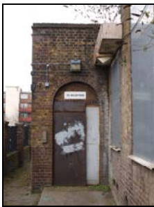
5852-019 (1/19) East elevation, north face of southern block. Facing south
