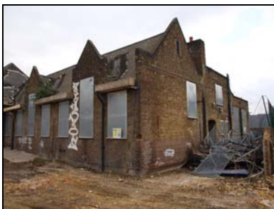
5852-007 (1/7) West and south elevations, oblique view. Facing northeast
