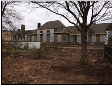
5852-029 (1/29) East elevation, oblique view from road. Facing northeast
