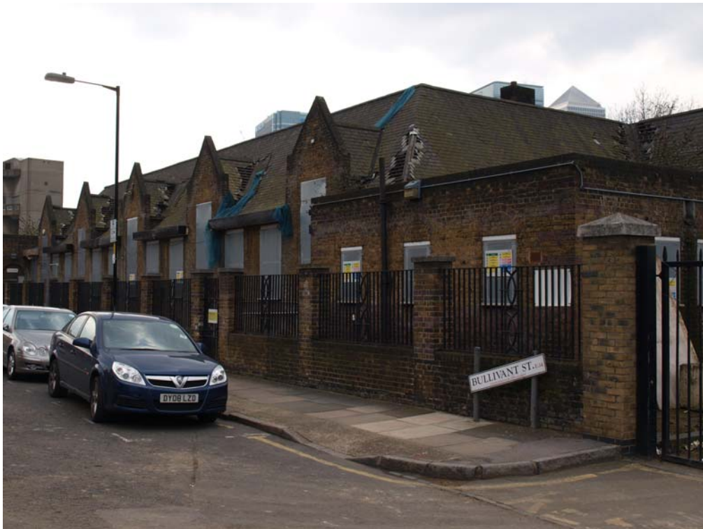
Plate 10. East elevation, oblique view. Facing southwest.
