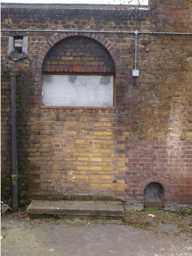
Plate 7. North elevation, blocked door and boot scraper. Facing south.
