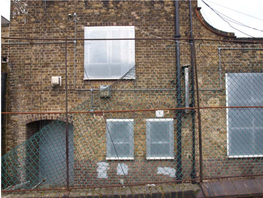
Plate 9. South elevation (central section). Facing north.
