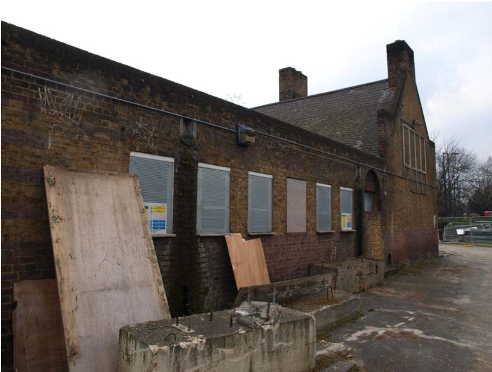
Plate 6. North elevation, oblique view, showing gable end of north wing and parapeted wall to flat roof behind. Facing west-southwest.
