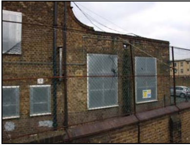
5852-013 (1/13) South elevation (eastern section). Facing northeast
