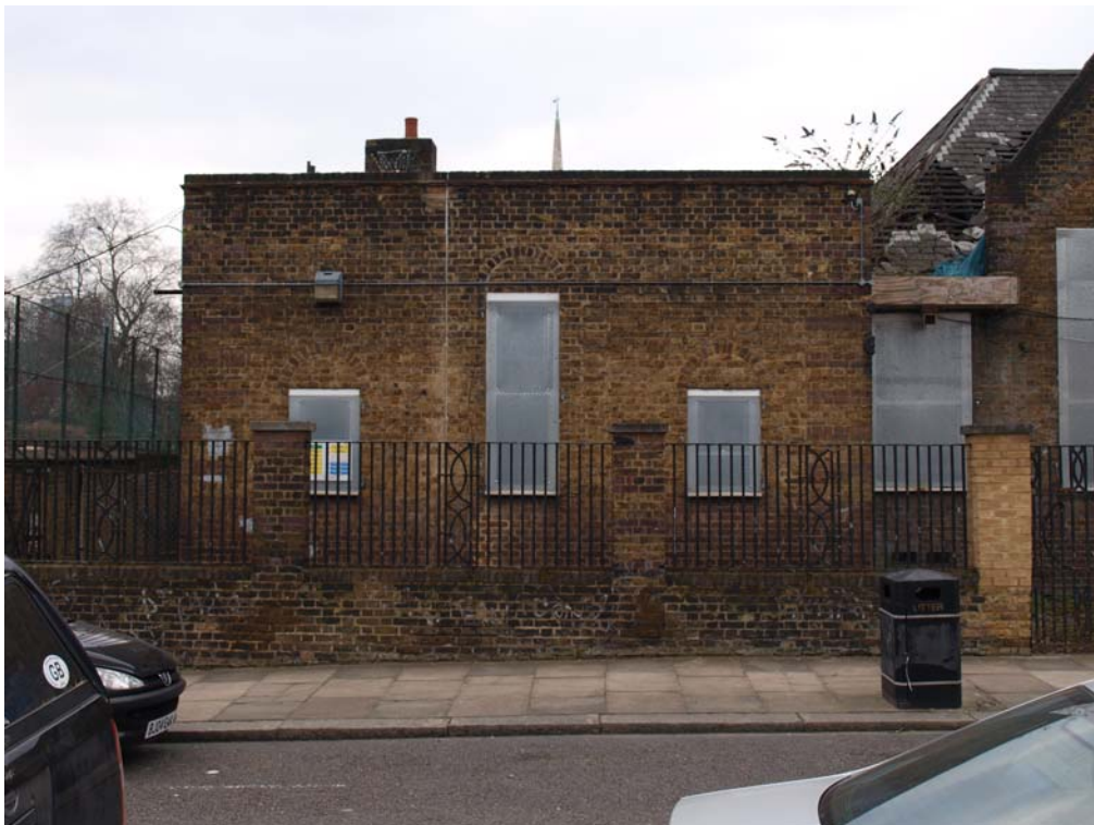
Plate 12. East elevation (southern section). Facing west.
