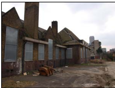
5852-005 (1/5) West elevation, oblique view. Facing south-southeast
