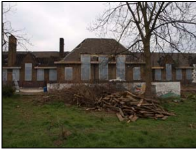
5852-028 (1/28) East elevation (central section) from road. Facing east
