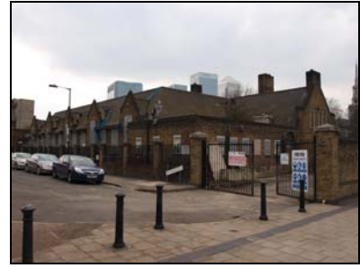
5852-027 (1/27) East and north elevations, oblique view. Facing southwest
