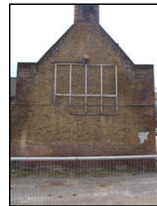
5852-012 (1/12) North elevation (western section). Facing south
