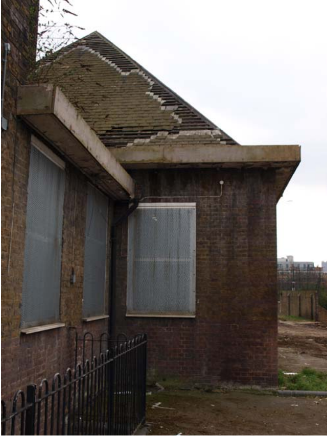
Plate 5. North elevation, north face of central block. Facing south.
