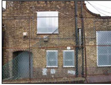
5852-014 (1/14) South elevation (central section). Facing north-northeast
