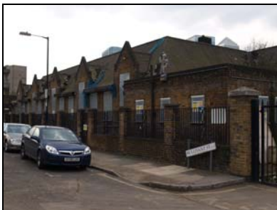
5852-022 (1/22) East elevation, oblique view. Facing southwest
