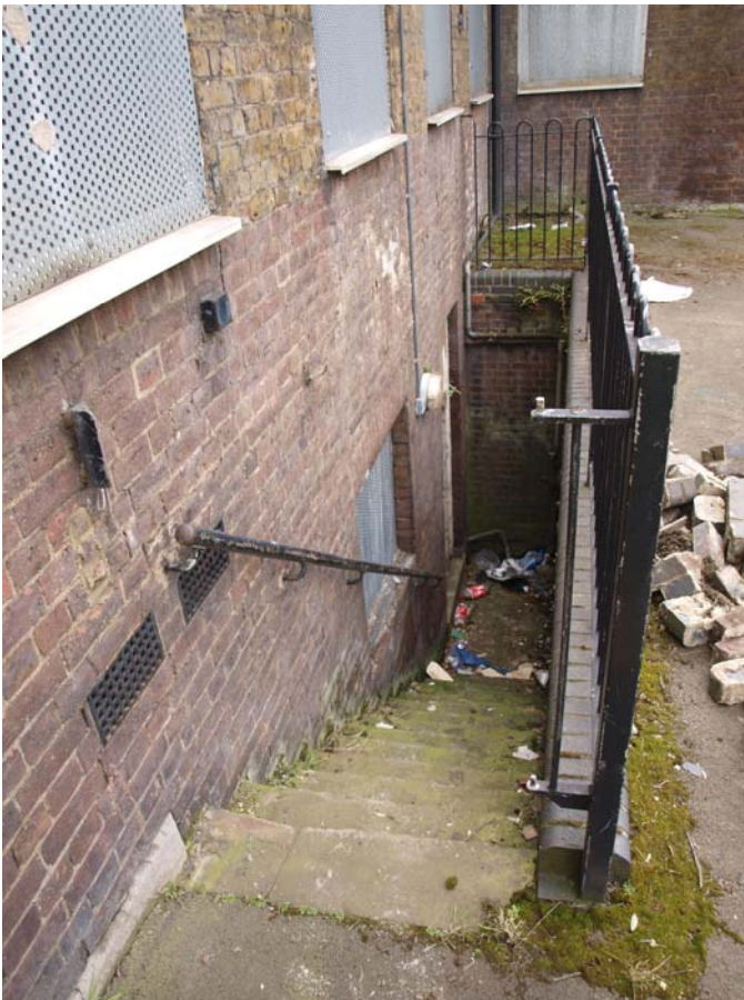
Plate 4. West elevation, view down basement steps. Facing south.
