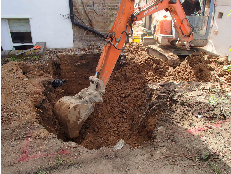
Working shot facing south-west
