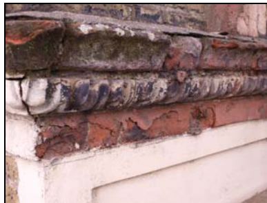
6119-05 (1/5) South elevation, detail of moulded decoration below main arch. Facing north-northeast
