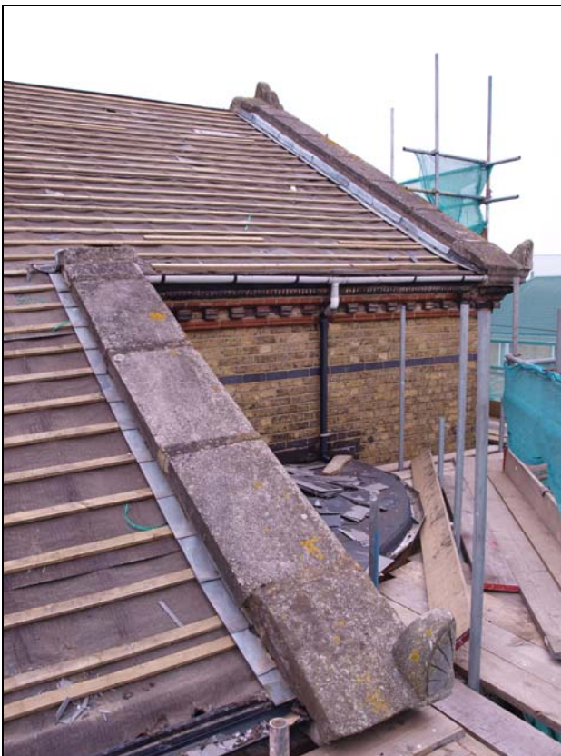
Plate 16. Coping to gable end of roof, south elevation (16)
