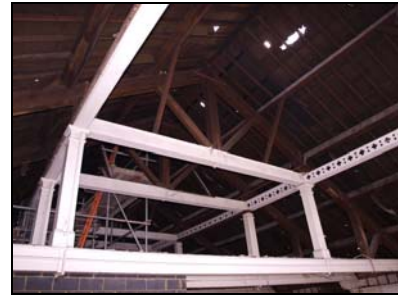
6119-42 (2/7) Roof, view of trusses. Facing southwest
