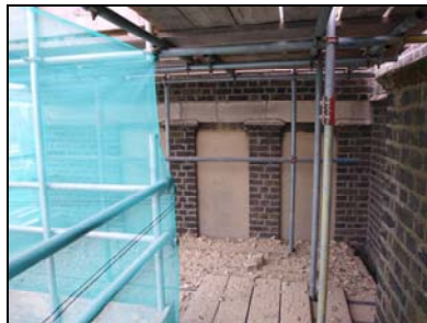
6119-17 (1/17) West elevation, blocked windows at upper level. Facing east
