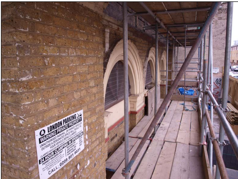
Plate 4. Arches to arcade in south elevation (20)
