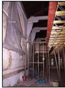
6119-38 (2/3) Interior, general view showing jowled posts supporting roof trusses. Facing north
