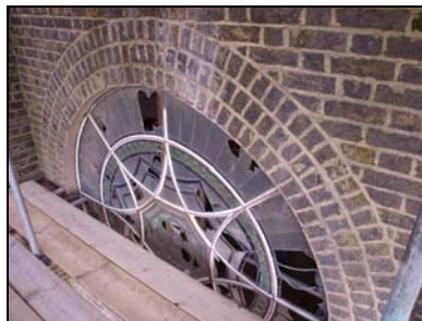
6119-08 (1/8) West elevation, large window. Facing northeast
