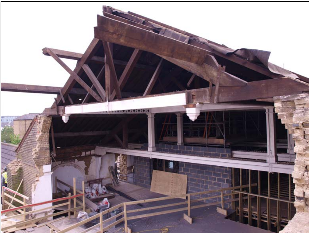
Plate 20. Roof structure showing purlins notched into principle rafter (15)
