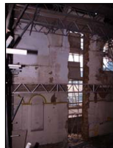
6119-33 (1/33) Interior, east elevation showing blocked windows. Facing east-southeast
