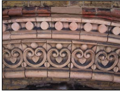
6119-11 (1/11) South elevation, detail of decorative arch over arcade. Facing north
