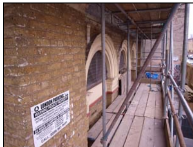
6119-20 (1/20) South elevation, arcade. Facing east-northeast
