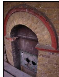
6119-21 (1/21) South elevation, window in stair turret, lower level. Facing north-northeast
