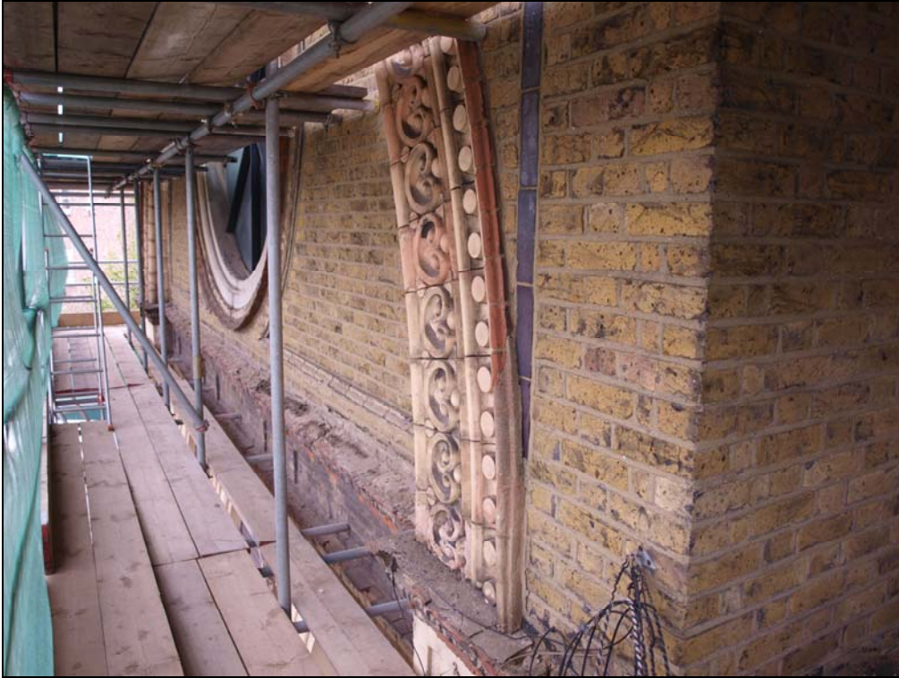
Plate 5. Arch over arcade in south elevation (4)
