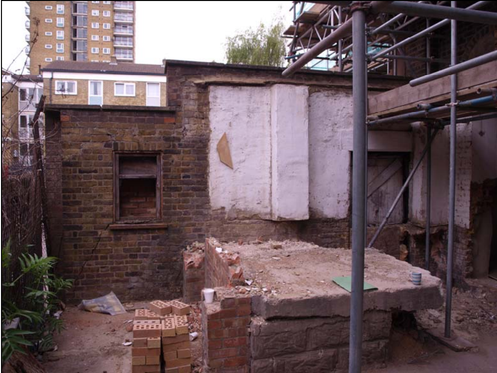
Plate 23. Adjoining wall, north end of west elevation (24)
