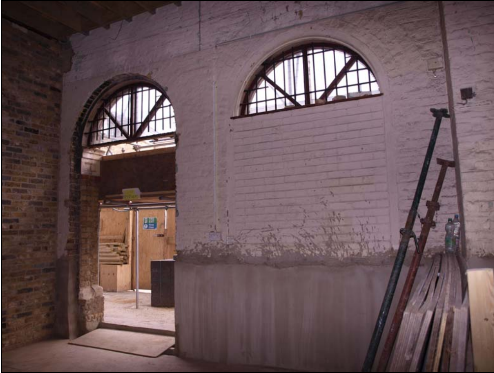
Plate 21. Interior wall of south elevation (48)
