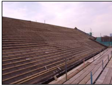
6119-14 (1/14) Roof, general view. Facing southeast
