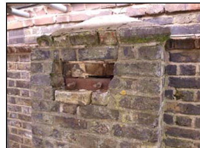
6119-09 (1/9) West elevation, truss tie set within buttress. Facing east-northeast
