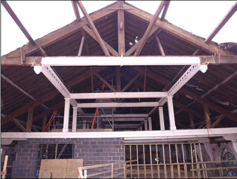
Plate 19. Roof trusses (41)
