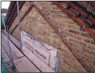
6119-49 (2/14) South elevation, detail of gable showing inscribed plaque. Facing northwest
