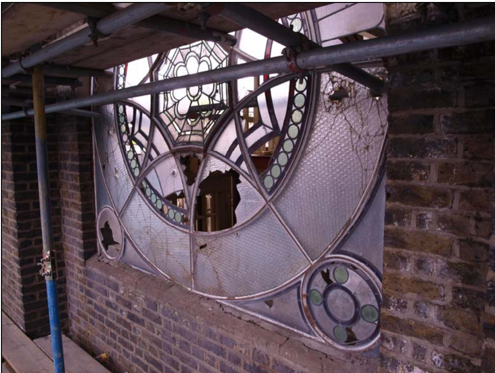
Plate 12. Lower part of window, upper level of west elevation (19)
