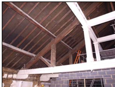
6119-44 (2/9) Roof, view of trusses. Facing south-southeast
