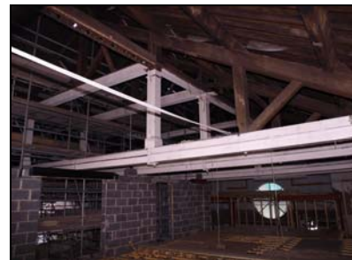
6119-45 (2/10) Roof, view of trusses. Facing south-southeast
