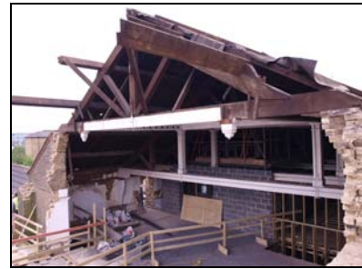
6119-15 (1/15) Roof, structure visible where east elevation has been removed. Facing southeast
