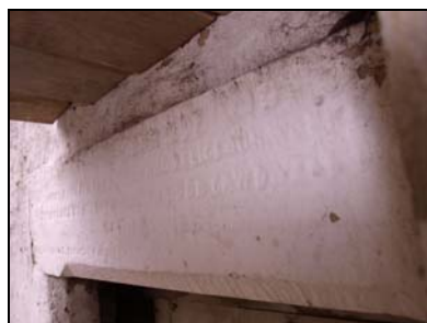
6119-27 (1/27) Wall at north end of building, inscription. Facing northwest
