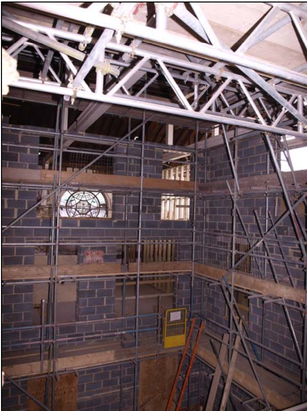
Plate 2. General view of interior (2)
