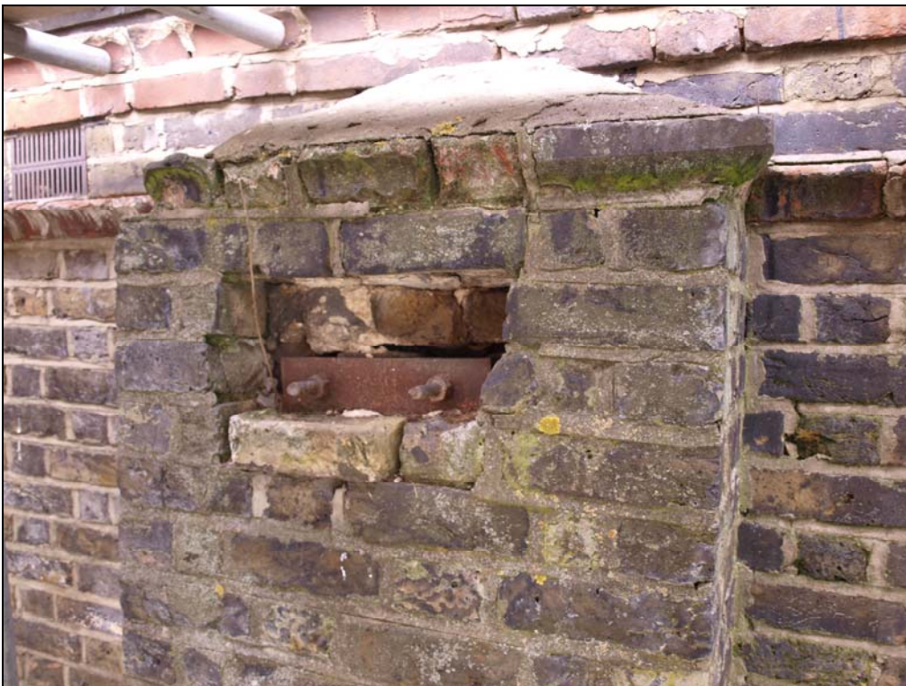
Plate 18. Tie plate and rods securing roof truss to buttress (9)
