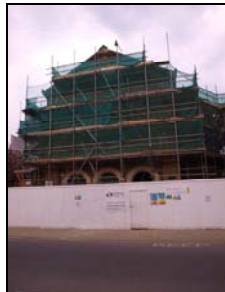
6119-28 (1/28) South elevation, general view. Facing north
