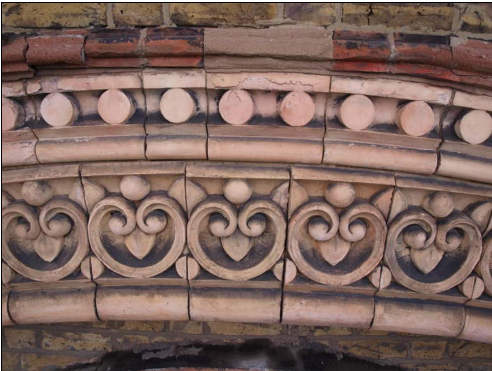
Plate 6. Detail of decoration to arch in south elevation (11)
