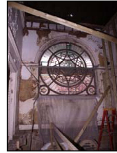
6119-36 (2/1) Interior, large window in west elevation. Facing west
