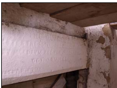
6119-26 (1/26) Wall at north end of building, inscription. Facing northeast
