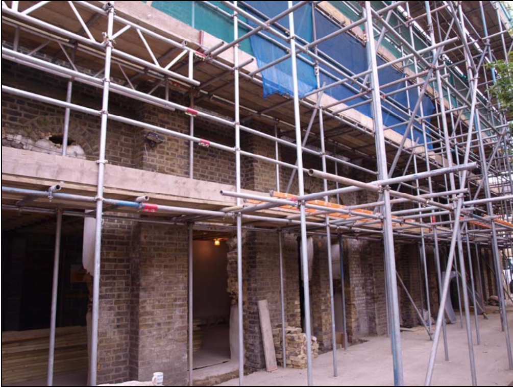
Plate 11. Buttresses in west elevation dividing it into alternating wide and narrow panels (23)
