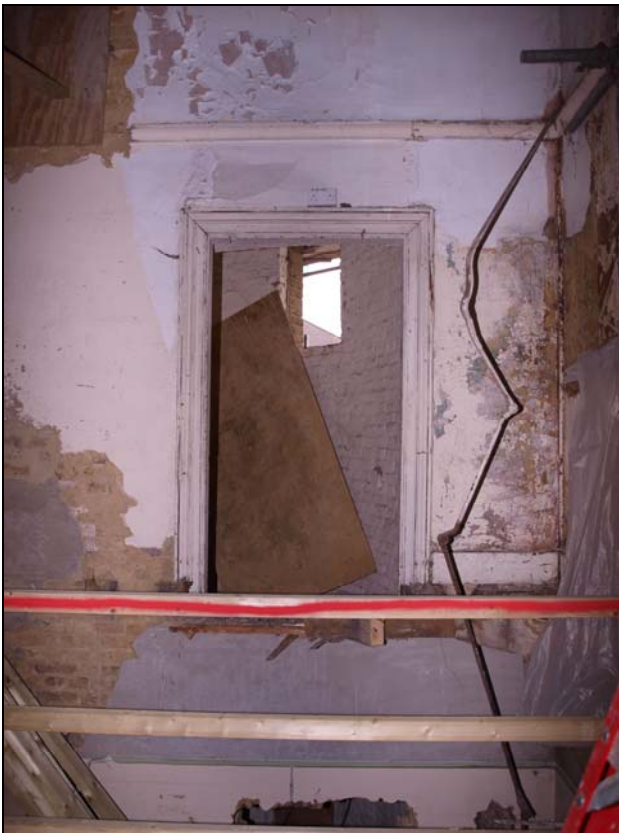
Plate 22. Doorway between main body of the building and southwest turret (37)
