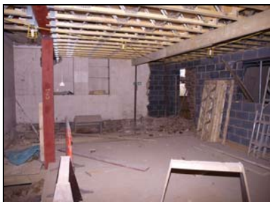
6119-32 (1/32) Interior, general view. Facing east-southeast
