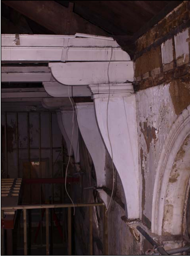
Plate 17. Timber corbels supporting roof trusses (46)
