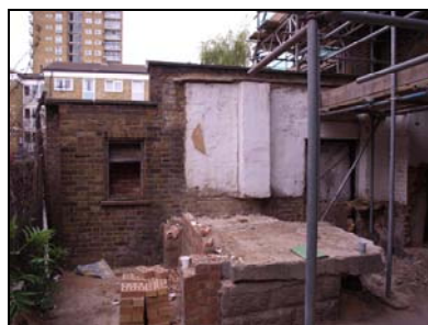
6119-24 (1/24) Wall at north end of building. Facing north
