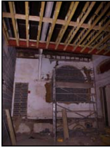
6119-34 (1/34) Interior, east elevation showing blocked windows. Facing east
