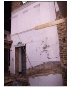
6119-39 (2/4) Interior, blocked windows in west elevation. Facing west-southwest
