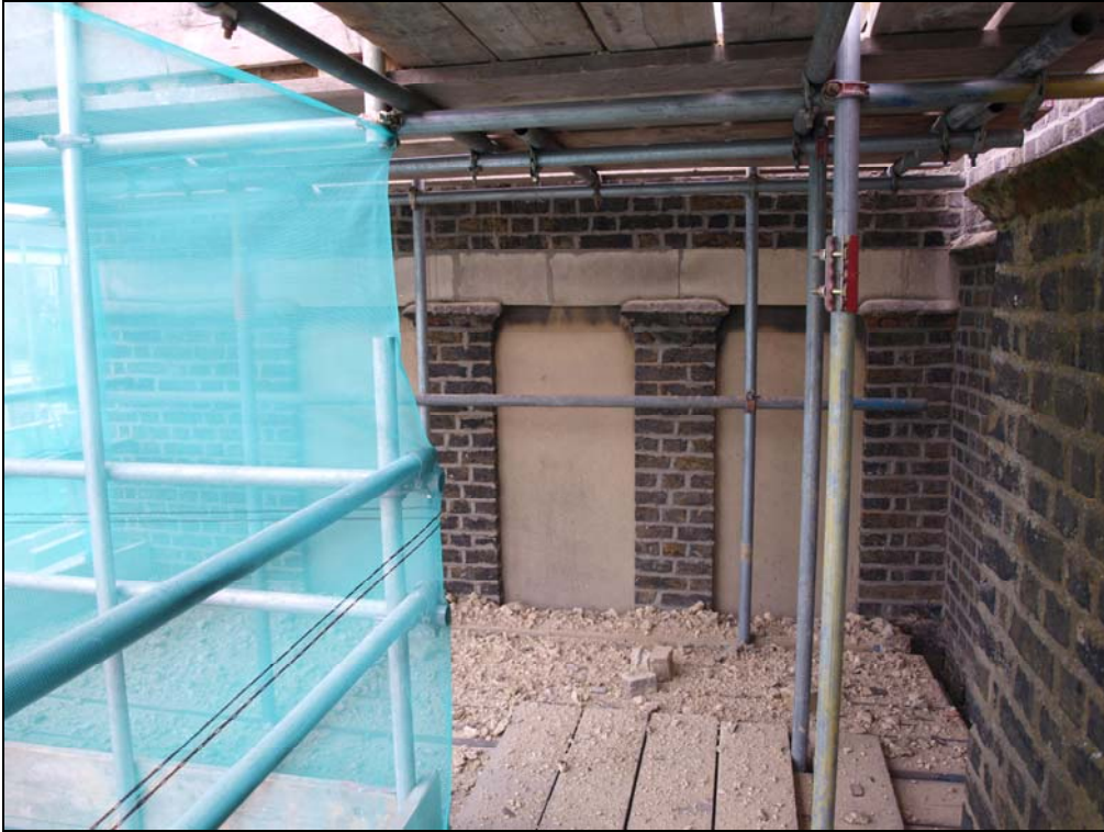
Plate 13. Blocked windows in west elevation, upper level (17)
