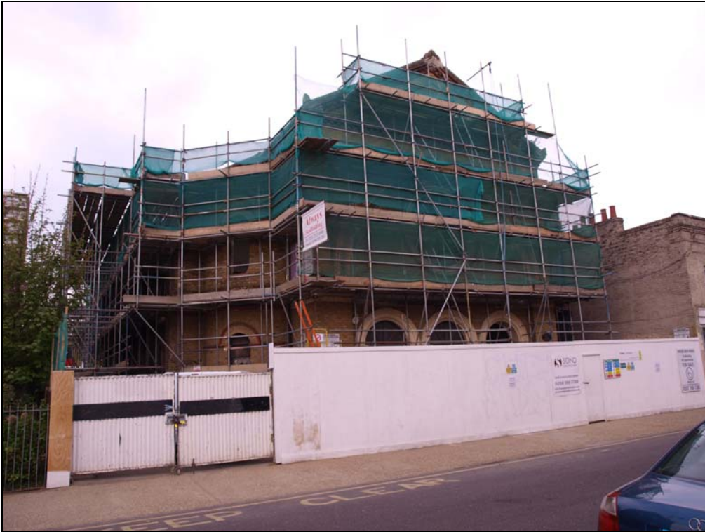
Plate 1. General view of south elevation at the time of survey (29)
