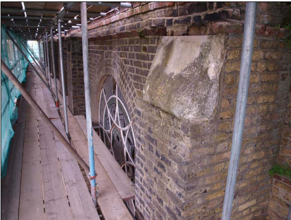
Plate 10. Buttress at west of south elevation capped with limestone, and window of west elevation (7)
