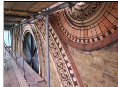
6119-06 (1/6) South elevation, decorated arch above arcade and roundel. Facing northwest
