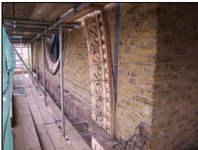
6119-04 (1/4) South elevation, decorated arch above arcade. Facing west-northwest
