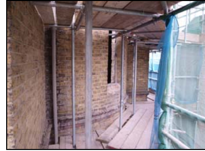
6119-03 (1/3) South elevation, stair turret at upper level. Facing north
