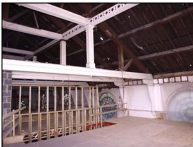
6119-43 (2/8) Roof, view of trusses. Facing south-southwest
