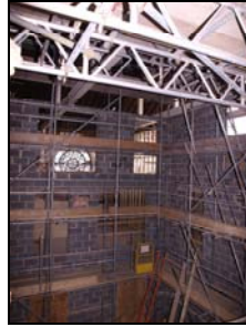
6119-02 (1/2) Interior, general view. Facing northwest
