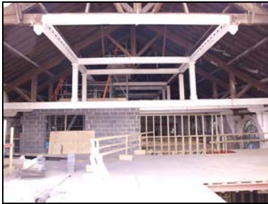
6119-40 (2/5) Roof, view of trusses. Facing south
