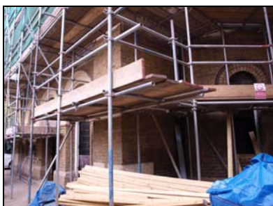
6119-22 (1/22) South elevation, general view. Facing northwest
