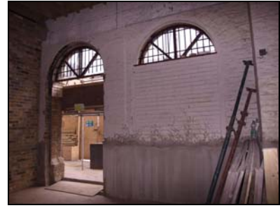
6119-48 (2/13) Interior, doorway in south elevation. Facing south-southeast
