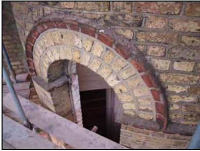
6119-10 (1/10) South elevation, window, upper level of stair turret. Facing north-northeast
