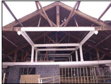
6119-41 (2/6) Roof, view of trusses. Facing south
