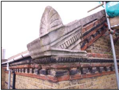
6119-13 (1/13) South elevation, detail of gable end. Facing northeast
