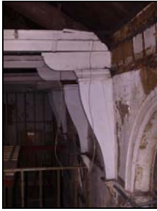
6119-46 (2/11) Roof, jowled posts and 'corbels' supporting trusses. Facing south
