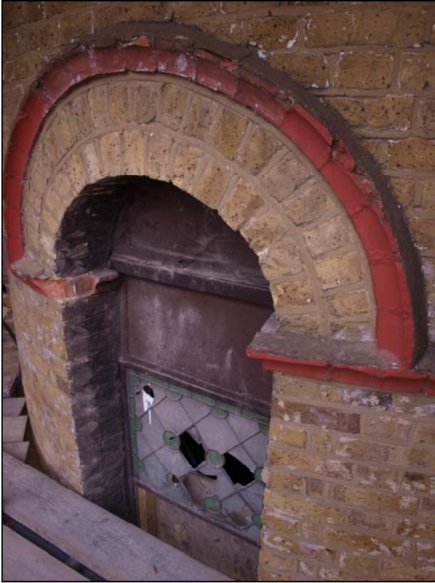
Plate 9. Window in western turret, lower level (21)
