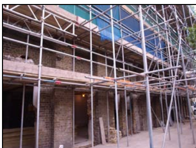
6119-23 (1/23) West elevation, general view. Facing south-southeast
