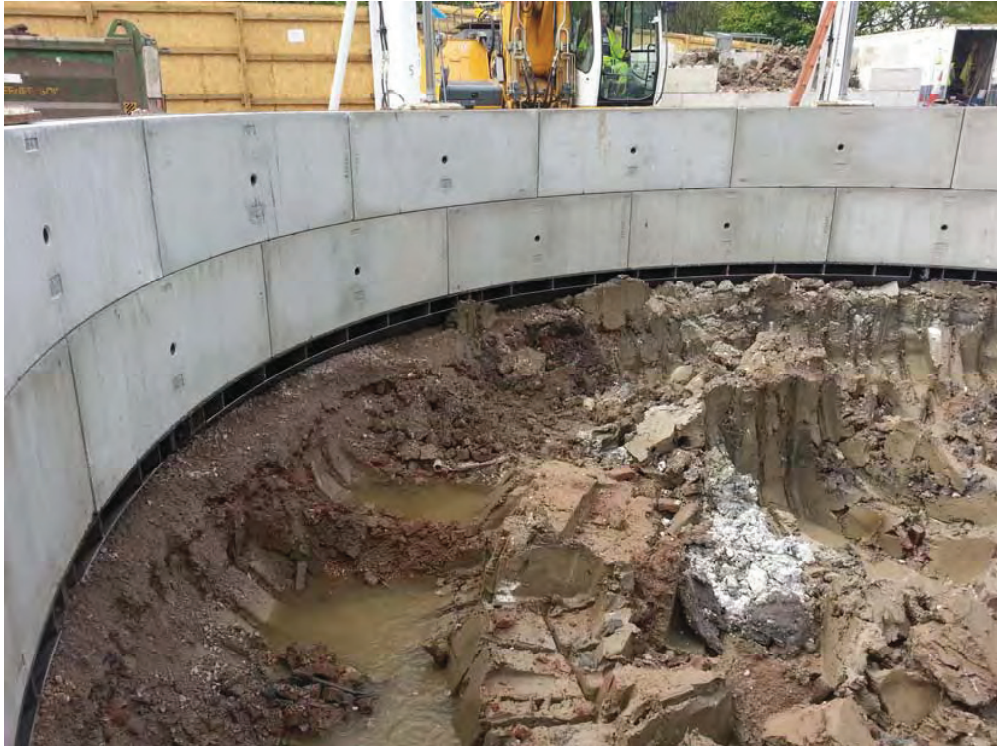
Made ground [001], alluvium [002] and chalky material [003]
