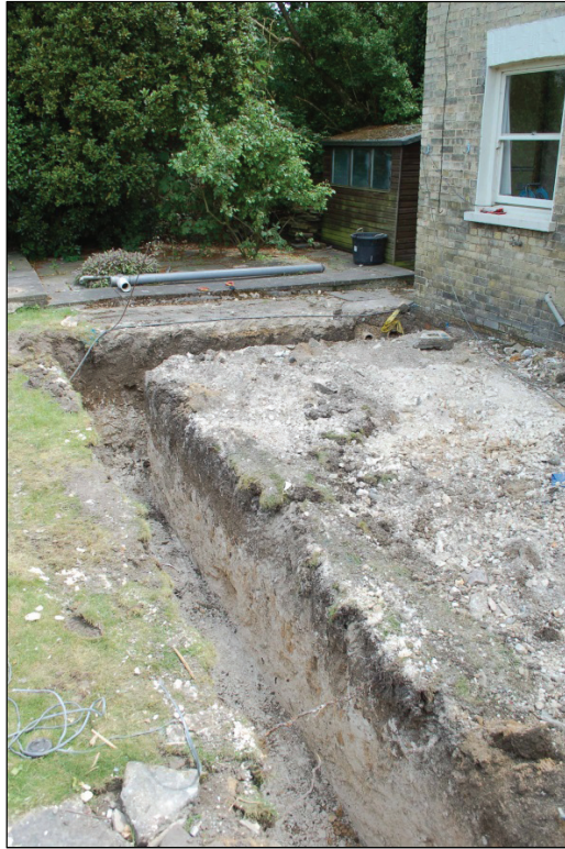
Fig. 3. Rear extension, looking east
