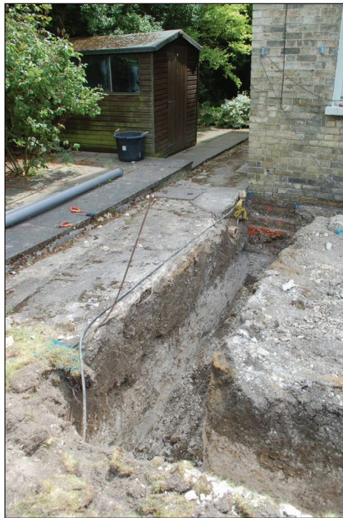
Fig. 4. Rear extension, looking south-east
