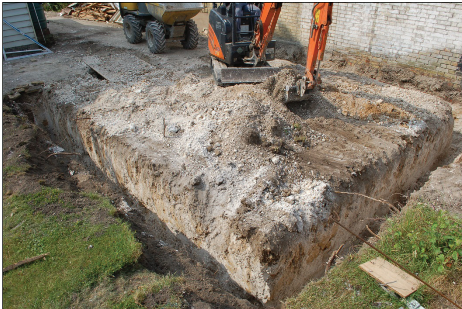
Fig. 6. Garage, looking south
