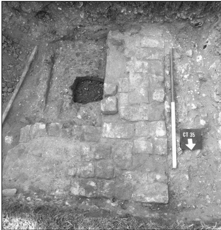
Figure 4: Wall 05, looking south (1m scale)
