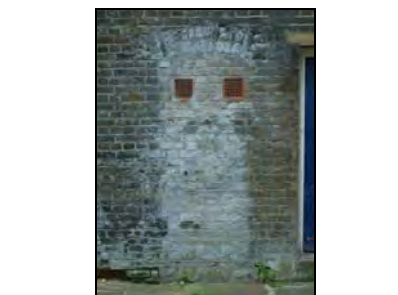
e2668-12 Northeast elevation, blocked door. Facing southwest
