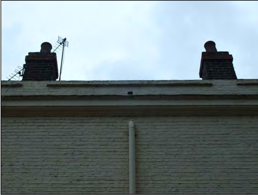
Plate 9. Northeast elevation, cornice, parapet & chimney stacks. Facing southwest (59)
