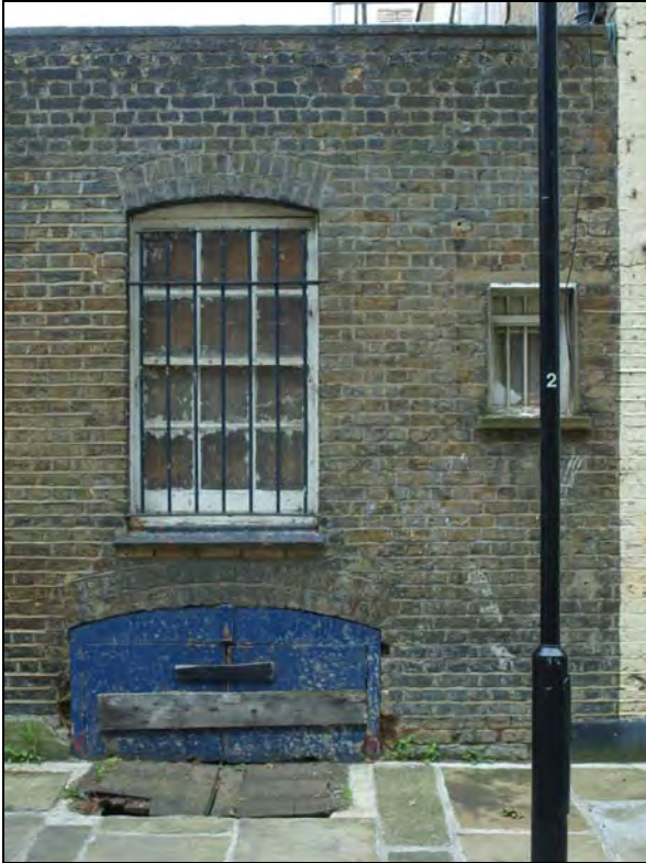
Plate 11. Northeast elevation, windows and cellar access. Facing southwest (10)
