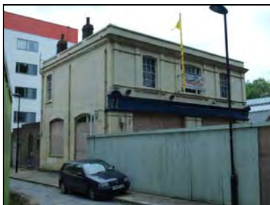
e2668-07 Northwest and northeast elevations. Facing south
