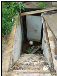
e2668-31 Cellar steps. Facing northwest
