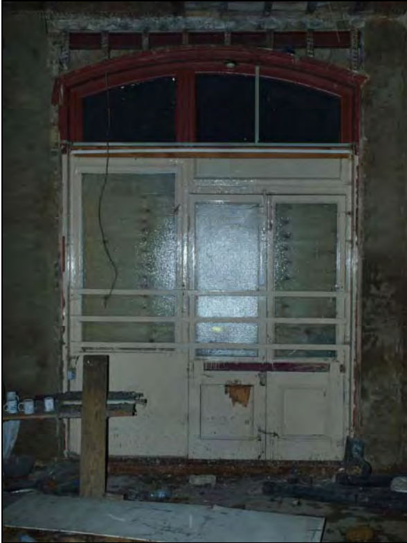
Plate 31. Interior, ground floor, door in side wall. Facing northeast (42)
