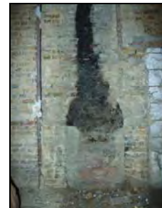
e2668-45 Interior, former fireplace. Facing southwest
