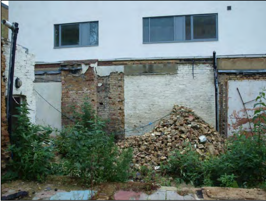
Plate 17. Rear boundary wall, showing capped flue at left. Facing southeast (25)
