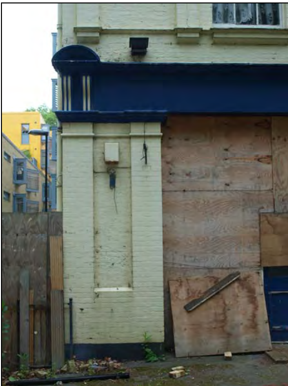
Plate 2. Northwest elevation, pilaster. Facing southeast (16)
