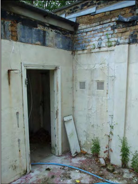
Plate 21. Doorway between demolished store and extant outbuilding. Facing north (27)
