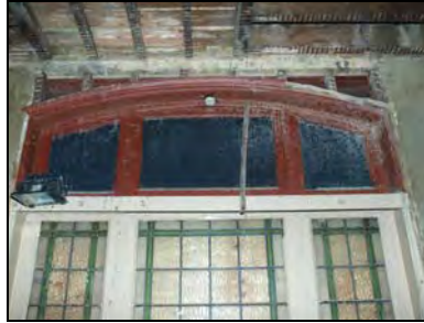
e2668-50 Interior, window in northeast elevation. Facing northeast
