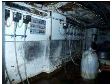
e2668-32 Cellar, interior. Facing northeast
