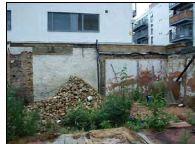
e2668-24 Internal face of southeast boundary wall. Facing southeast
