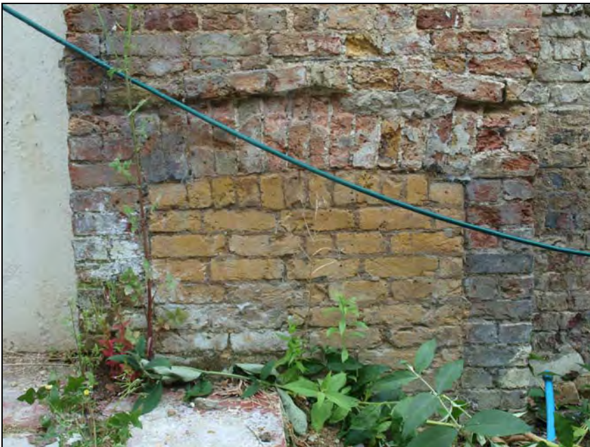
Plate 18. Rear boundary wall, blocked fireplace. Facing southeast (29)
