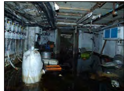
e2668-33 Cellar, interior. Facing east-northeast
