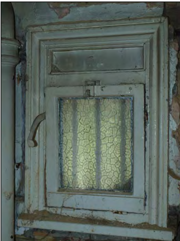
Plate 22. Window in outbuilding. Facing northeast (21)
