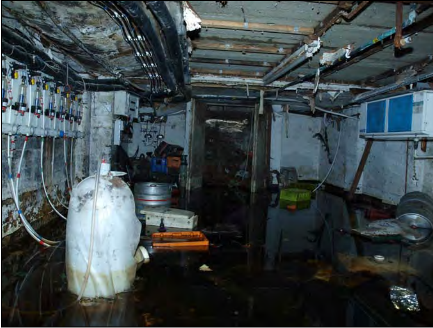
Plate 25. Cellar, general view. Facing east-northeast (33)
