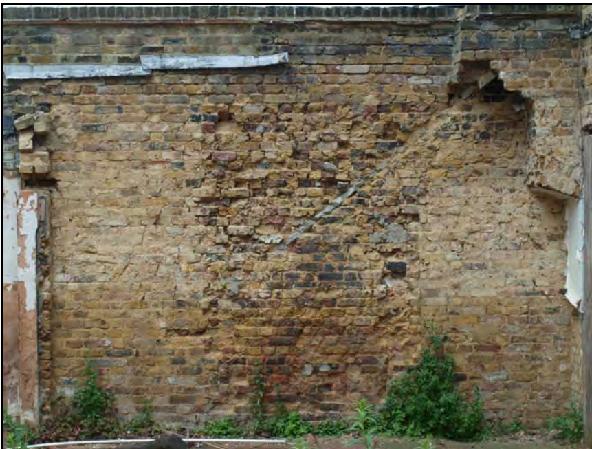
Plate 16. Southwest boundary wall. Facing southwest (20)
