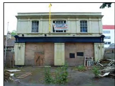
e2668-06 Northwest elevation. Facing southeast
