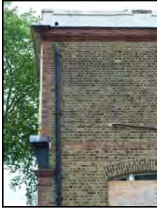
e2668-61 Southwest elevation, detail to corner, first floor. Facing northeast
