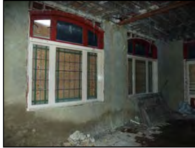
e2668-38 Interior, ground floor windows in southwest elevation. Facing west
