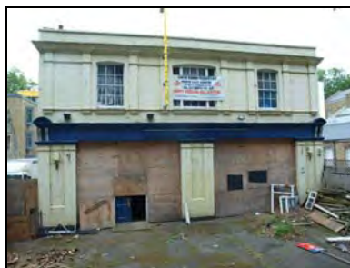
e2668-71 Northwest elevation. Facing southeast
