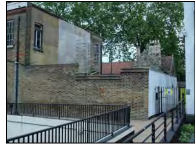
e2668-03 Southwest and southeast elevations. Facing north
