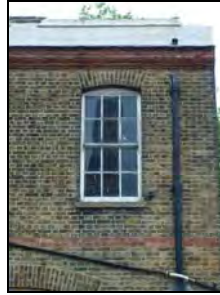
e2668-62 Southwest elevation, first floor window. Facing northeast
