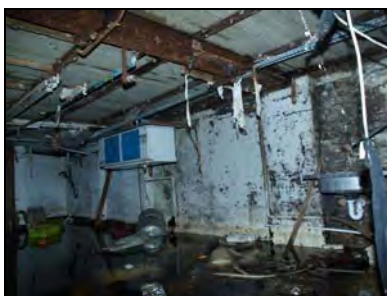
e2668-34 Cellar, interior. Facing east
