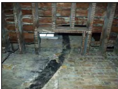
e2668-46 Interior, flue opening in ground floor ceiling. Facing southwest
