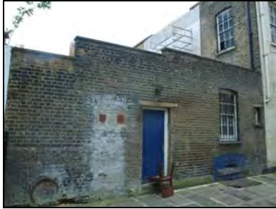
e2668-13 Northeast elevation, rear extension. Facing west-southwest
