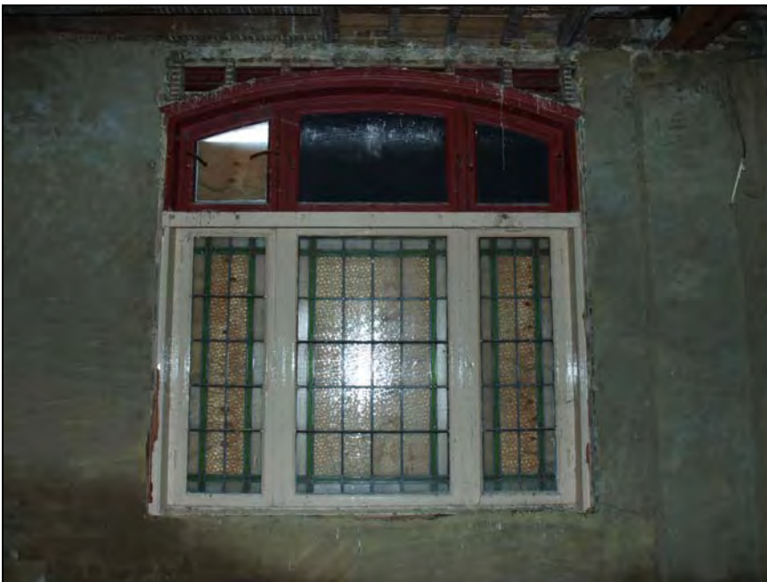
Plate 30. Interior, ground floor, window in side wall. Facing southwest (37)
