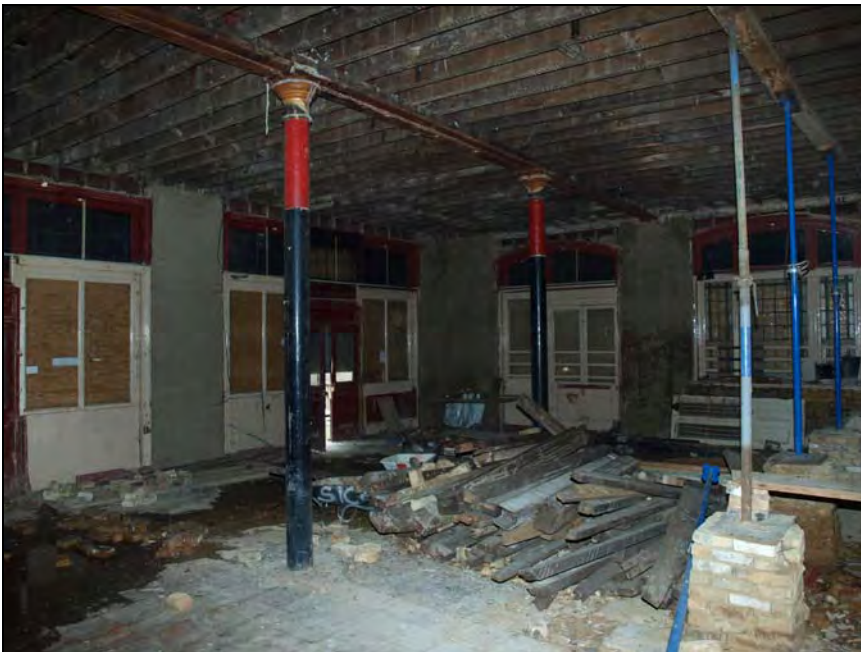
Plate 26. Interior, ground floor, general view. Facing north (40)
