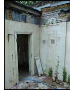
e2668-27 Doorway and blocked doorway, rear of building. Facing north
