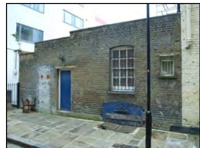
e2668-09 Northeast elevation, rear extension. Facing south
