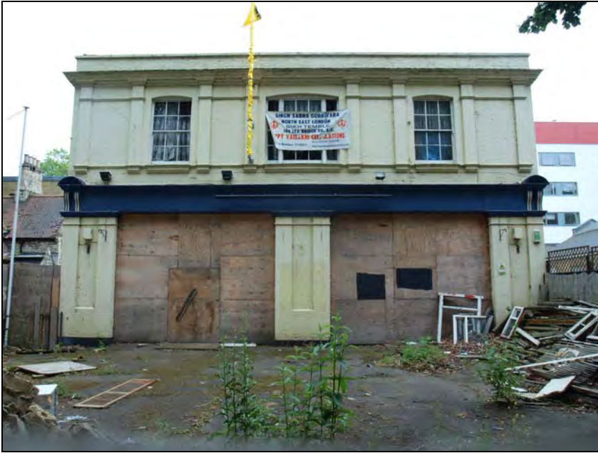
Plate 1. Northwest elevation. Facing southeast (06)
