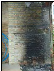
e2668-22 Blocked fireplace in outbuilding. Facing southeast
