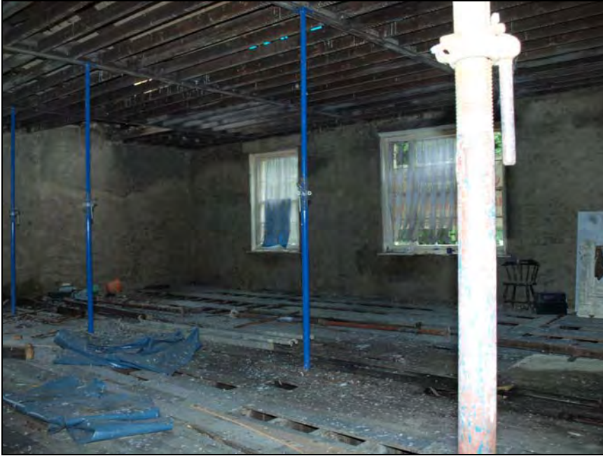
Plate 33. Interior, first floor, general view. Facing west (65)
