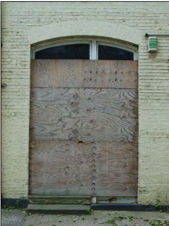
Plate 8. Northeast elevation, door. Facing southwest (55)
