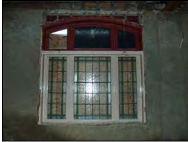
e2668-37 Interior, ground floor window in southwest elevation. Facing southwest
