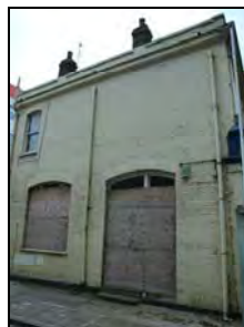
e2668-08 Northeast elevation, openings. Facing south
