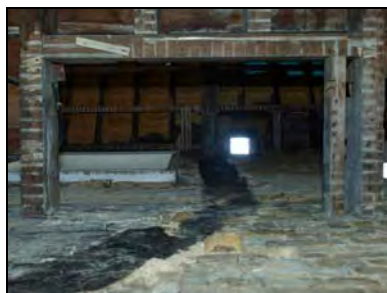
e2668-47 Interior, flue opening in roof. Facing southwest
