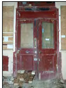
e2668-68 Interior, door in northwest elevation. Facing northwest
