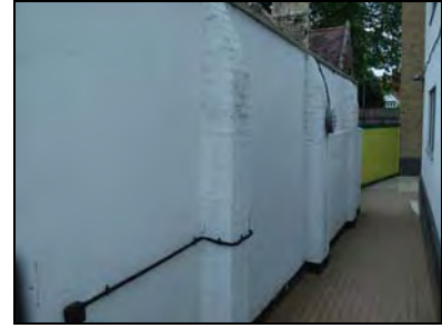
e2668-63 Rear of southeast boundary wall. Facing north
