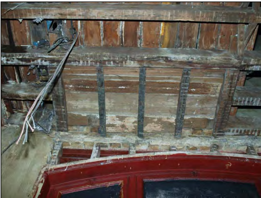
Plate 32. Interior, ground floor, hearth in floor above. Facing southwest (66)
