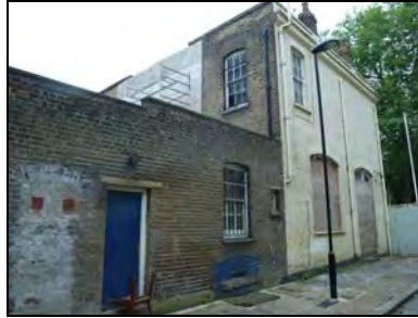
e2668-14 Northeast elevation. Facing west
