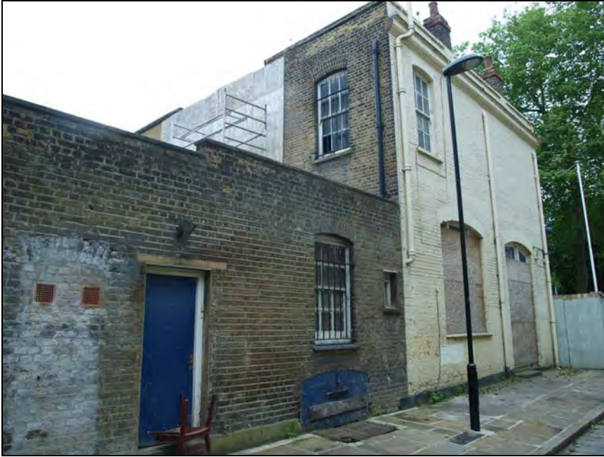
Plate 7. Northeast elevation, general view. Facing west (14)
