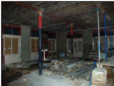
e2668-40 Interior, general view. Facing north
