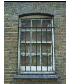
e2668-57 Northeast elevation, window. Facing southwest
