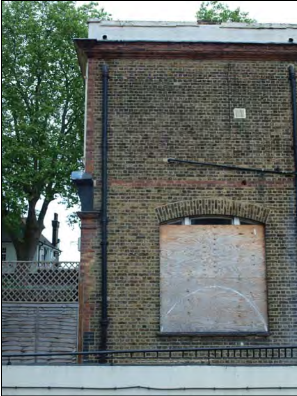
Plate 5. Southwest elevation, window & decorative string course. Facing northeast (04)
