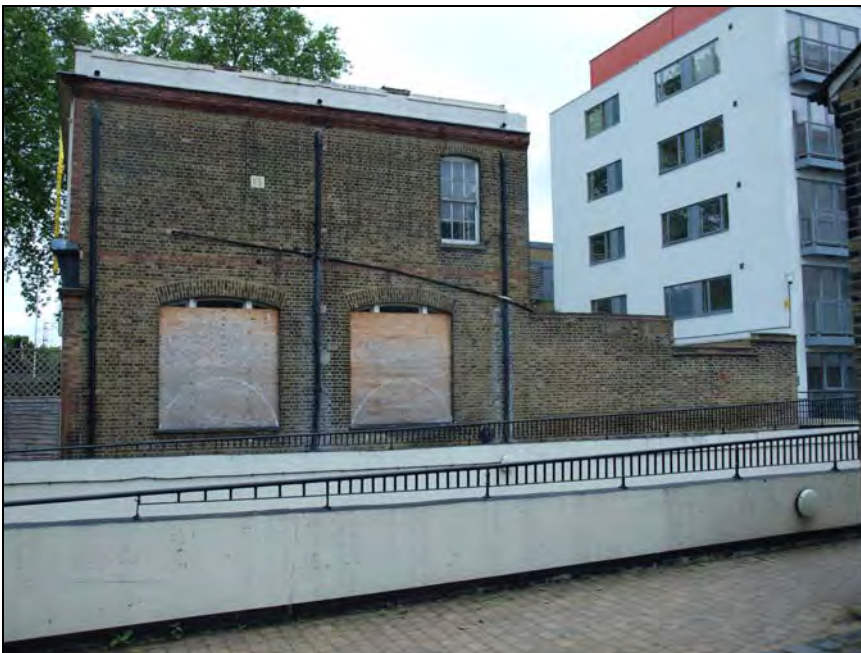
Plate 4. Southwest elevation, general view. Facing northeast (01)
