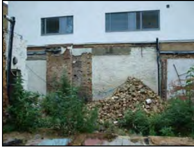
e2668-25 Internal face of southeast boundary wall. Facing southeast
