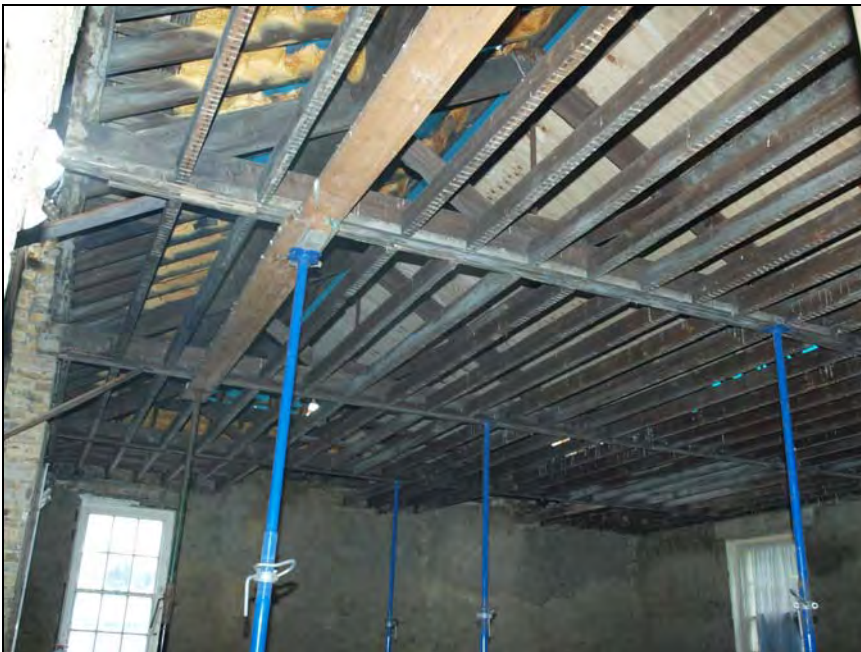
Plate 34. Roof, view of internal structure. Facing west (64)
