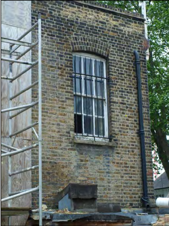
Plate 15. Southeast elevation, first floor window. Facing north (30)
