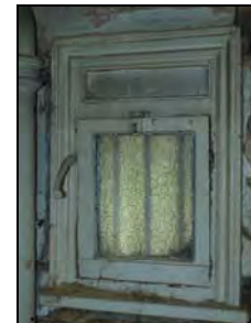
e2668-21 Internal view, window in northeast wall. Facing northeast
