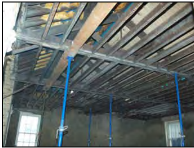
e2668-64 Roof, truss formation. Facing west
