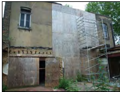
e2668-17 Southeast elevation. Facing north-northwest
