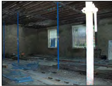
e2668-65 Interior, general view of first floor. Facing west
