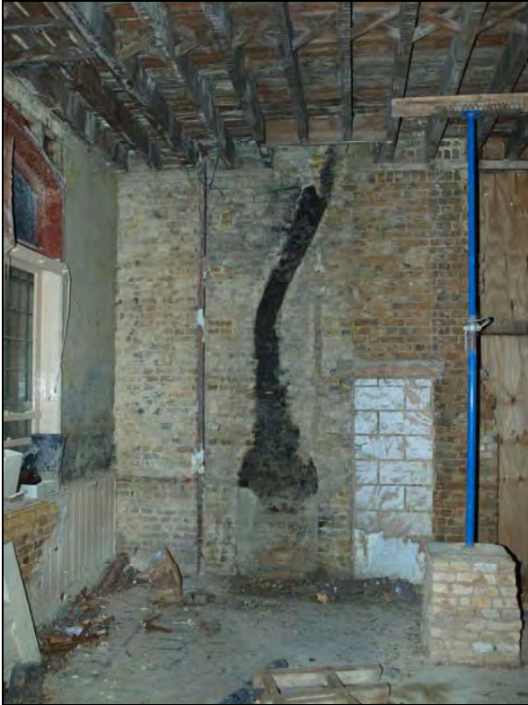
Plate 27. Interior, ground floor, eastern part of rear wall. Facing southwest (44)
