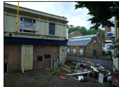
e2668-69 General shot showing relationship to carbolic acid works. Facing south
