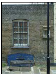
e2668-10 Northeast elevation, windows and cellar access. Facing southwest
