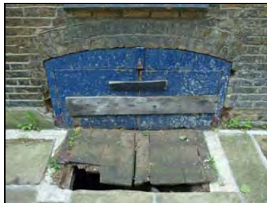
e2668-56 Northeast elevation, detail of cellar access. Facing southwest
