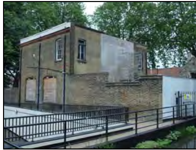
e2668-02 Southwest elevation. Facing north
