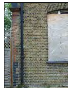
e2668-60 Southwest elevation, detail to corner, ground floor. Facing northeast
