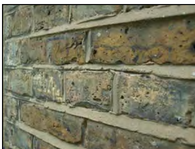
e2668-58 Northeast elevation, pointing. Facing south
