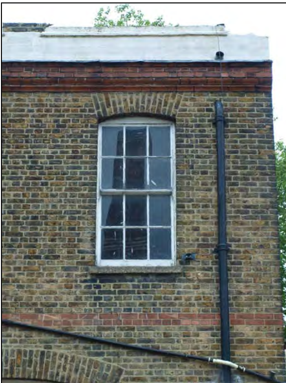
Plate 6. Southwest elevation, first floor window. Facing northeast (62)
