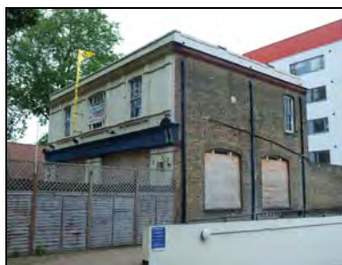
e2668-05 Northwest and southwest elevations. Facing west
