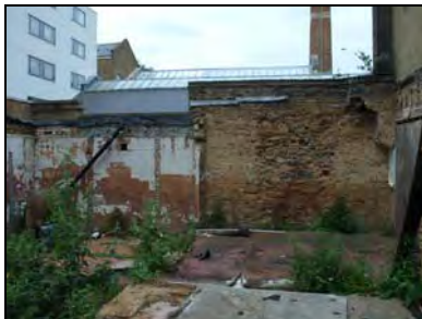
e2668-19 Internal face of southwest boundary wall. Facing southwest
