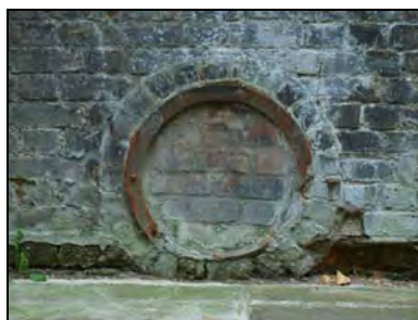
e2668-11 Northeast elevation, circular opening. Facing southwest
