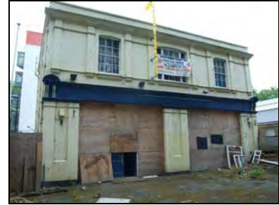
e2668-15 Northwest elevation. Facing south-southeast
