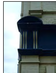
e2668-54 Northwest elevation, pilaster decoration. Facing southeast
