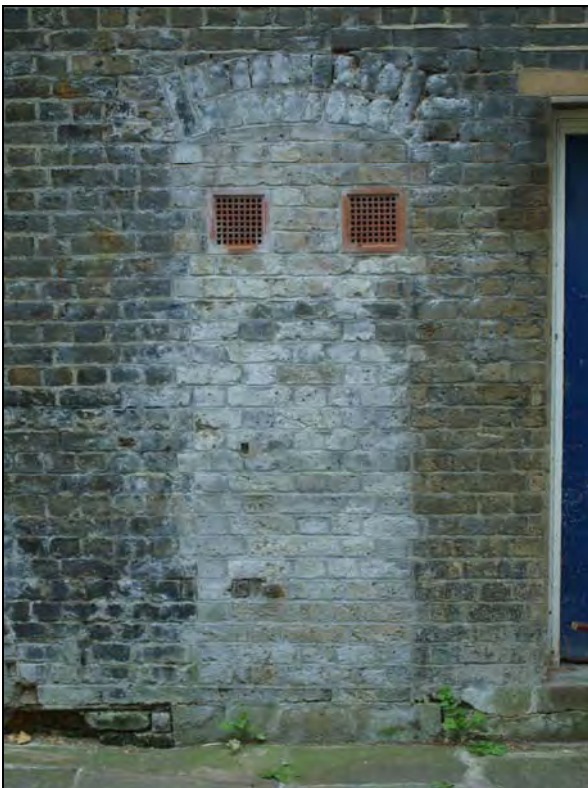
Plate 12. Northeast elevation, blocked doorway. Facing southwest (12)
