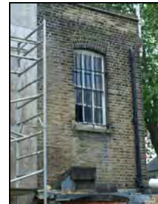
e2668-30 Southeast elevation, first floor window. Facing north
