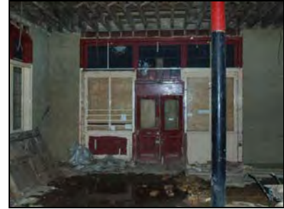
e2668-39 Interior, doorway in northwest elevation. Facing northwest
