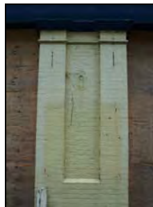
e2668-53 Northwest elevation, central pilaster. Facing southeast
