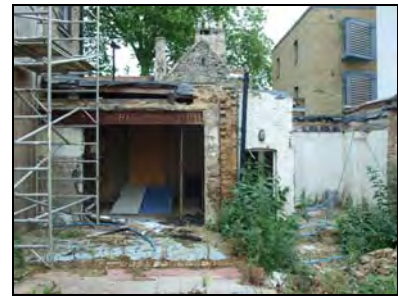
e2668-18 Remaining structure, rear of building. Facing northwest
