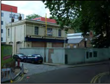
e2668-73 General location. Facing south
