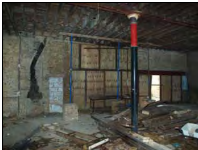
e2668-43 Interior, general view. Facing south
