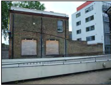
e2668-01 Southwest elevation. Facing northeast
