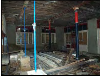
e2668-49 Interior, general view. Facing west
