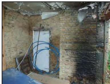
e2668-23 Interior of remaining structure, rear of building. Facing east
