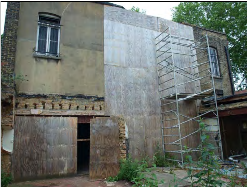
Plate 14. Southeast elevation, general view. Facing north-northwest (17)
