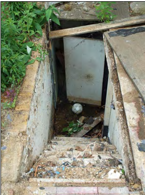
Plate 24. Cellar access at rear of building. Facing northwest (31)
