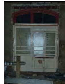
e2668-42 Interior, doorway in northeast elevation. Facing northeast
