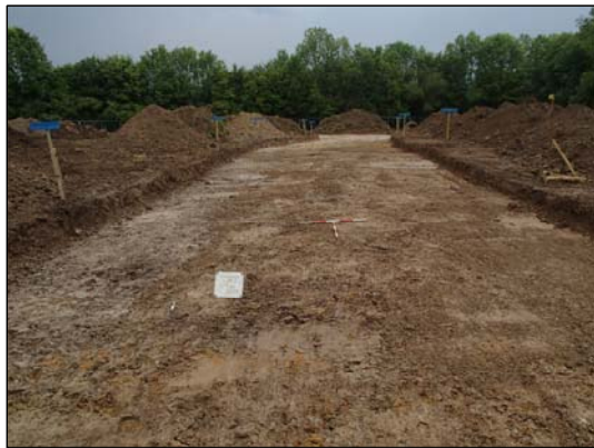
Fig. 3.1 Haul road looking North
