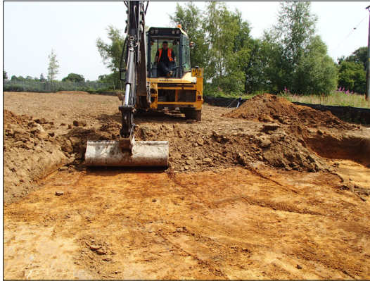
Fig. 3.1 Excavation area B looking south
