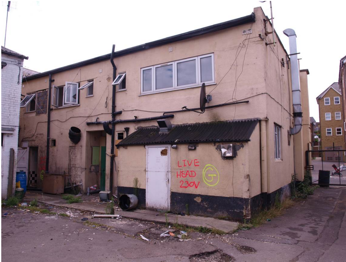
Plate 29: 75a and 75b South Street, east elevation (108)
