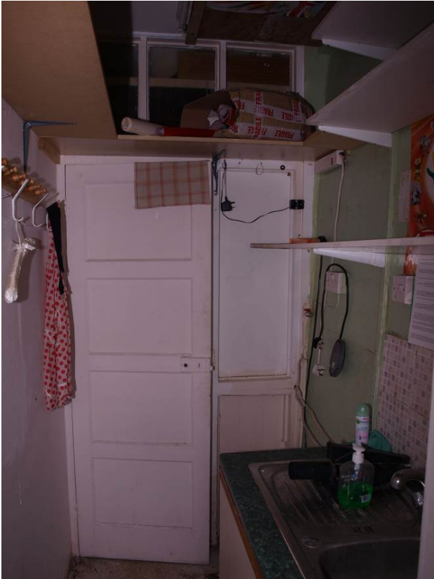
Plate 9: Room 3, looking north (17)
