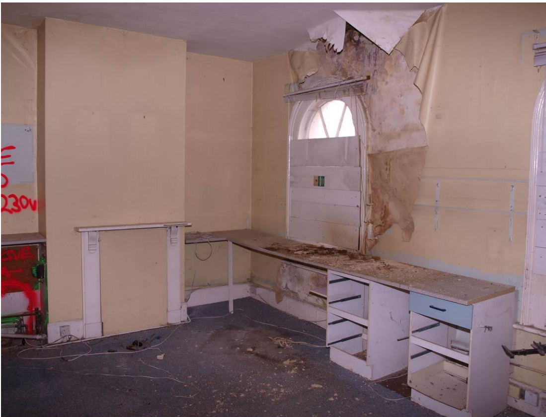
Plate 22: Room 12, looking south-west (51)
