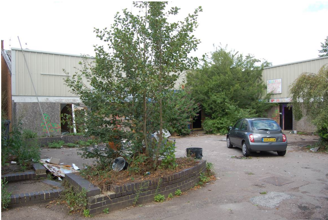
Plate 32: South Street Commercial Centre, Units 3-12, looking north-east (80)
