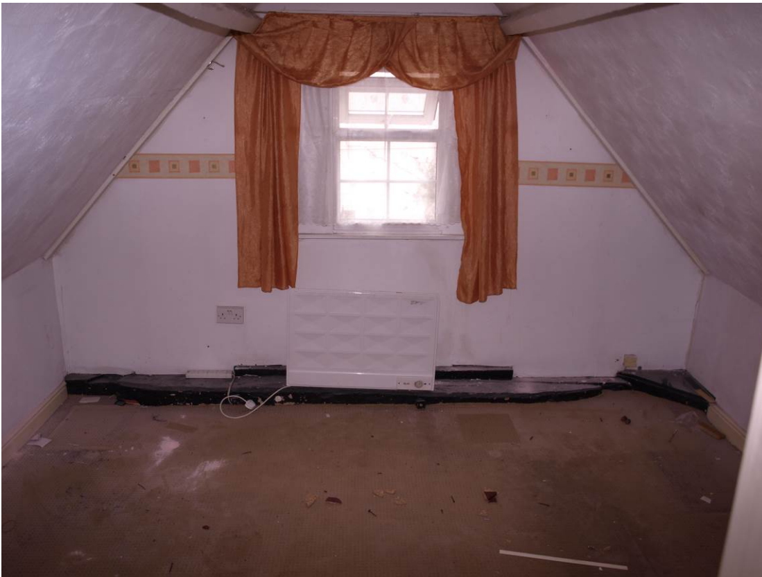
Plate 12: Timber kerb bolted to wall-plate, Room 9 (9)
