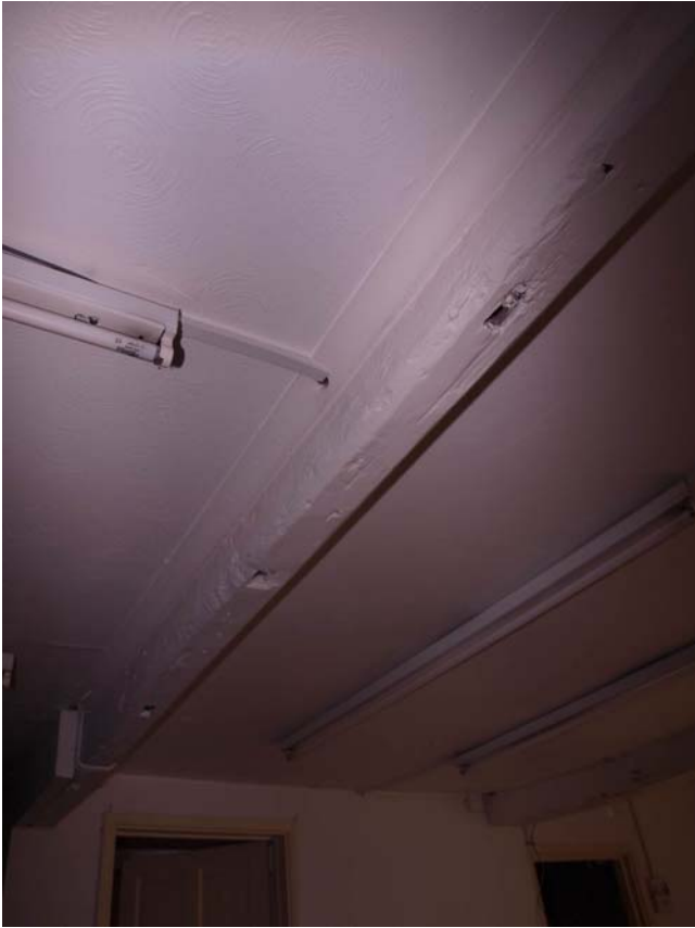
Plate 7: Mortices for former partition (16)
