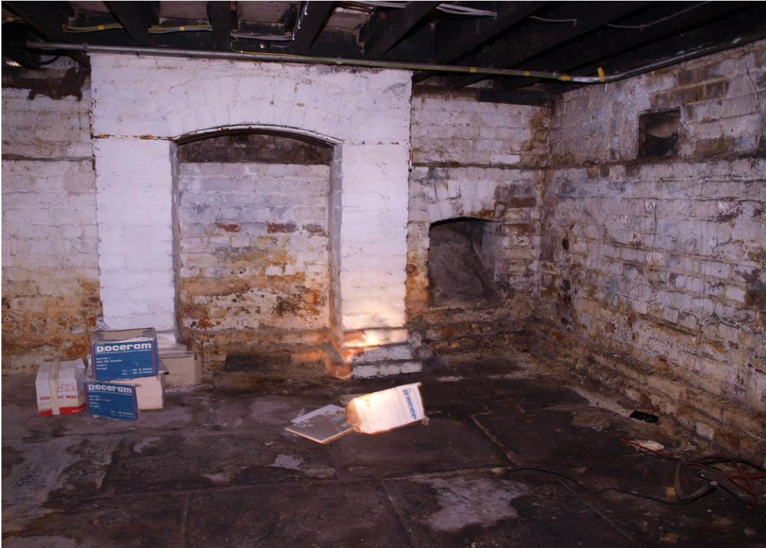
Plate 23: Cellar, looking south (54)
