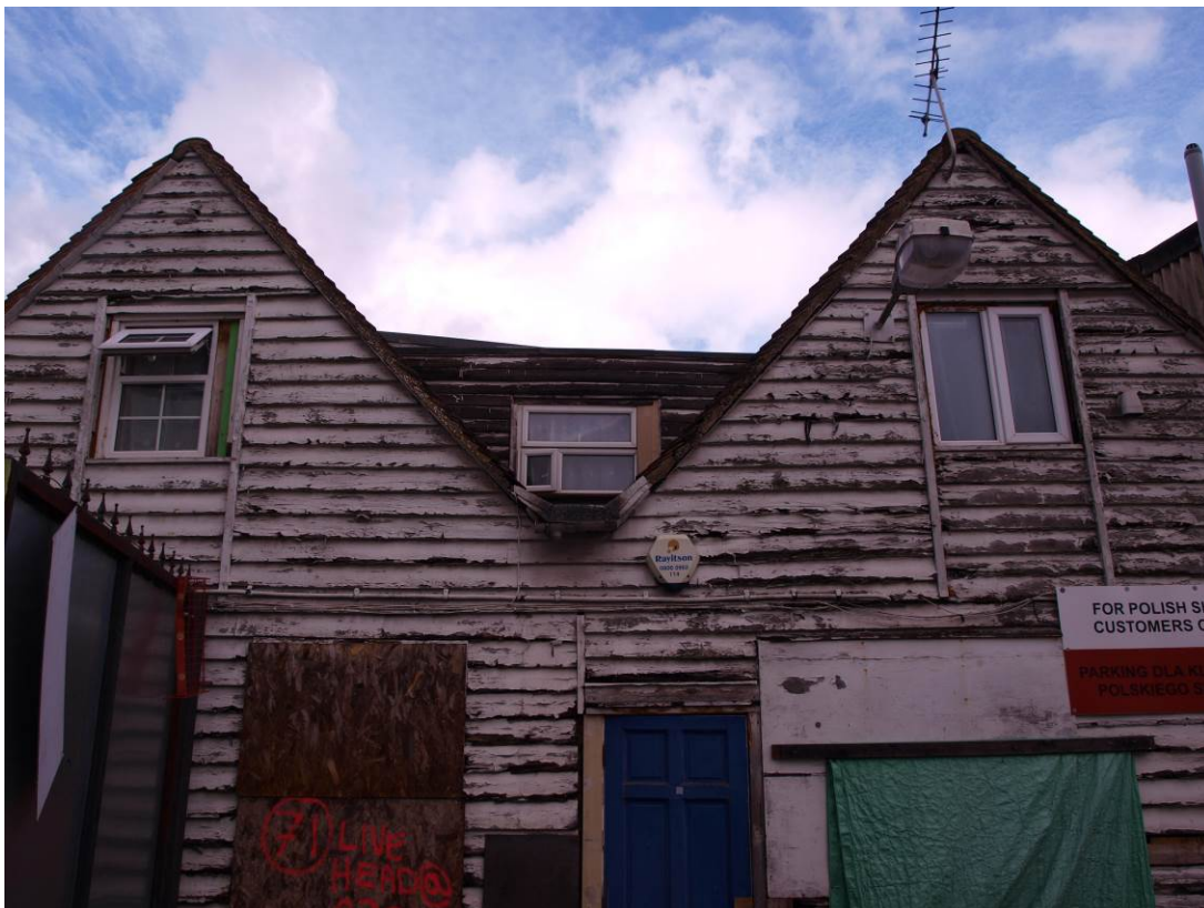
Plate 2: Flat-roofed dormer linking the central and eastern roofs (37)
