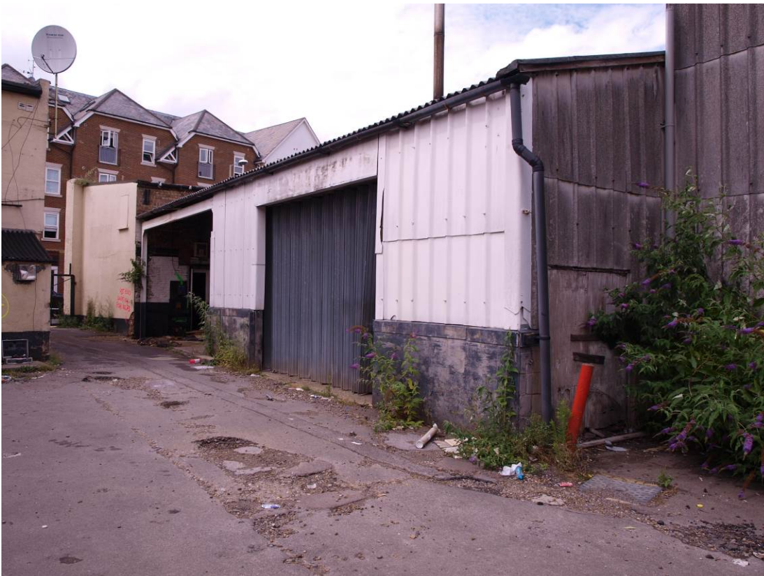
Plate 26: Rear additions to 73 South Street, looking west (26)
