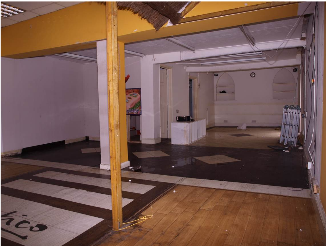
Plate 6: Room 1, looking east (3)
