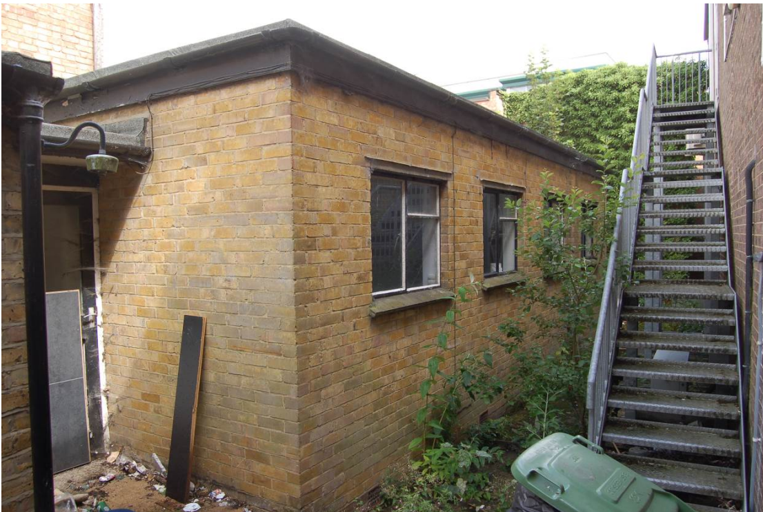
Plate 14: Modern extension to the west (57)
