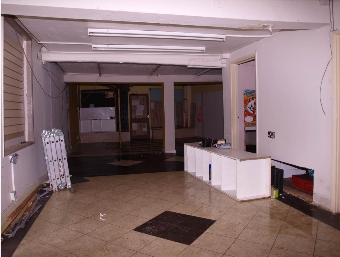
Plate 5: Room 1, looking west (1)
