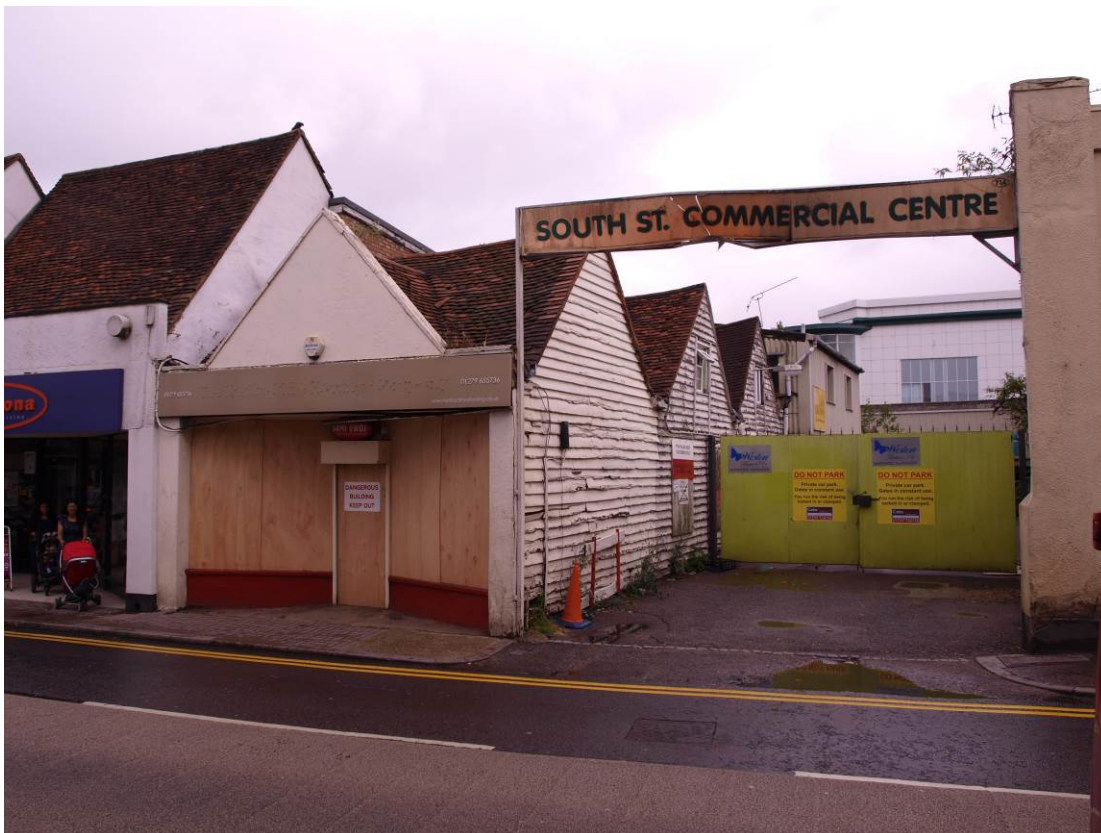
Plate 4: West elevation, looking north-east (27)
