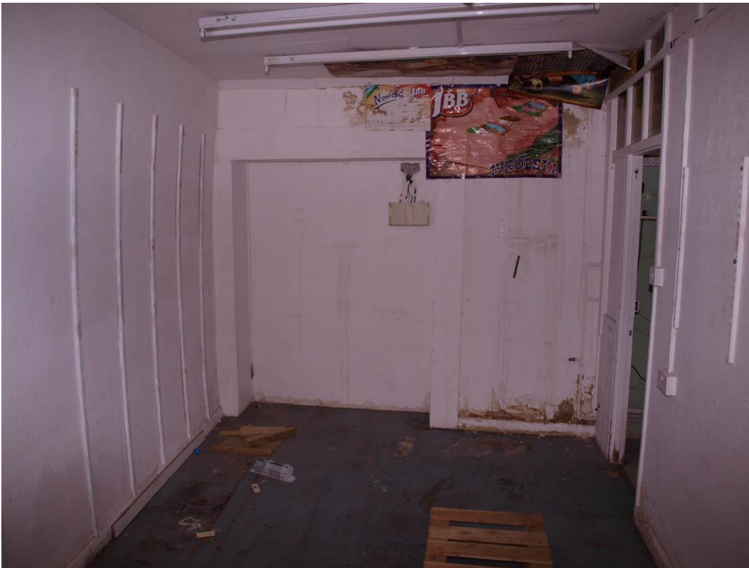
Plate 8: Room 2, looking west (4)
