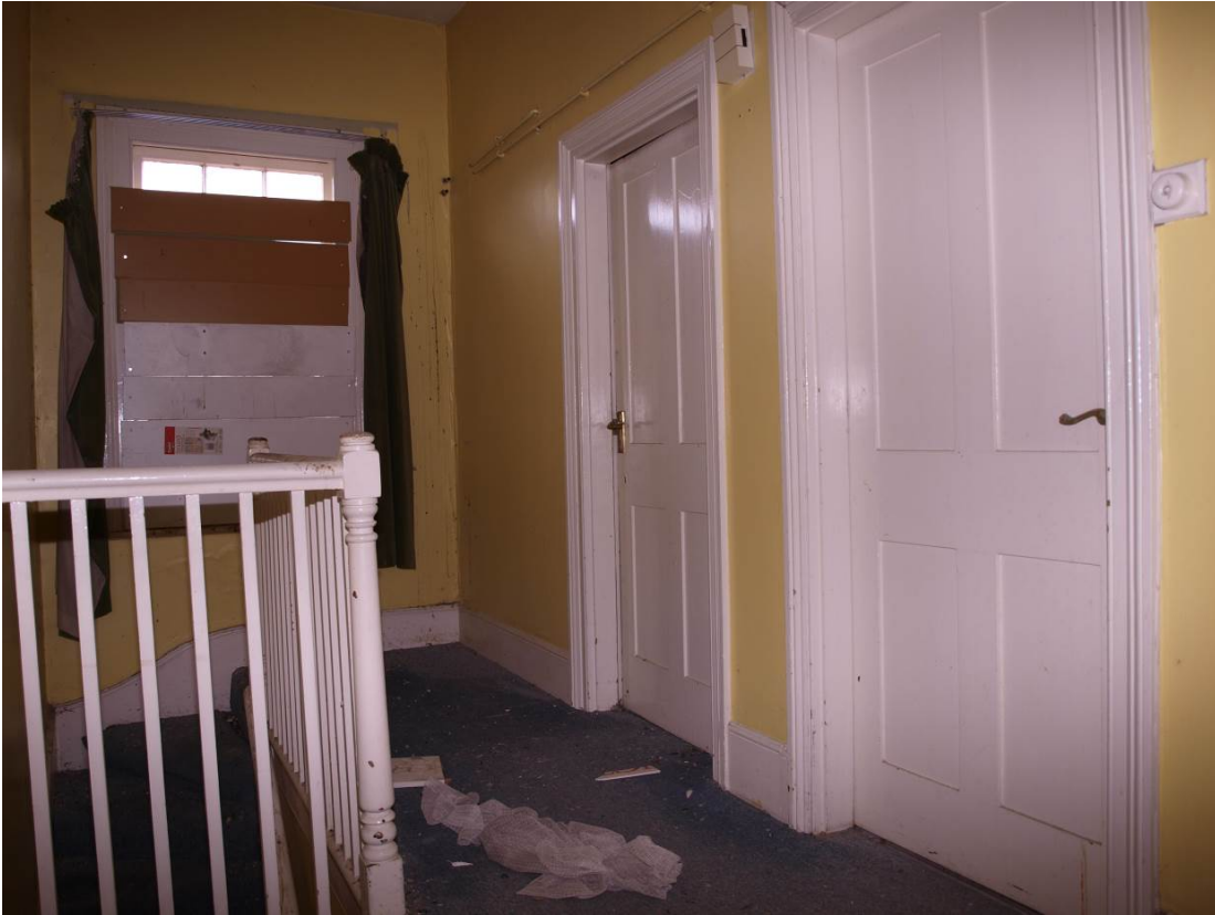
Plate 21: Stair landing, looking west (50)
