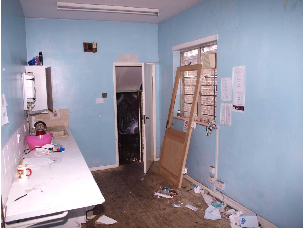
Plate 19: Room 8, looking west (39)
