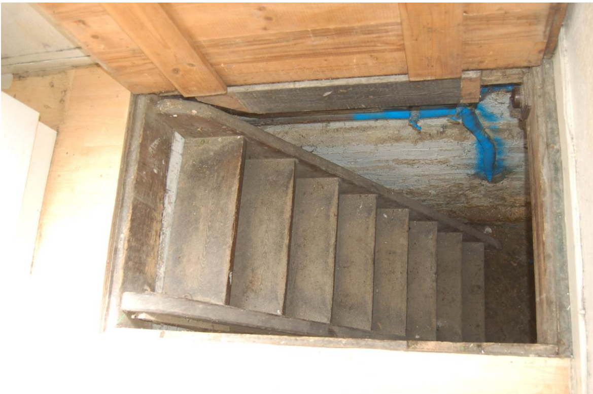
Plate 18: Trap door and steps leading to cellar (56)
