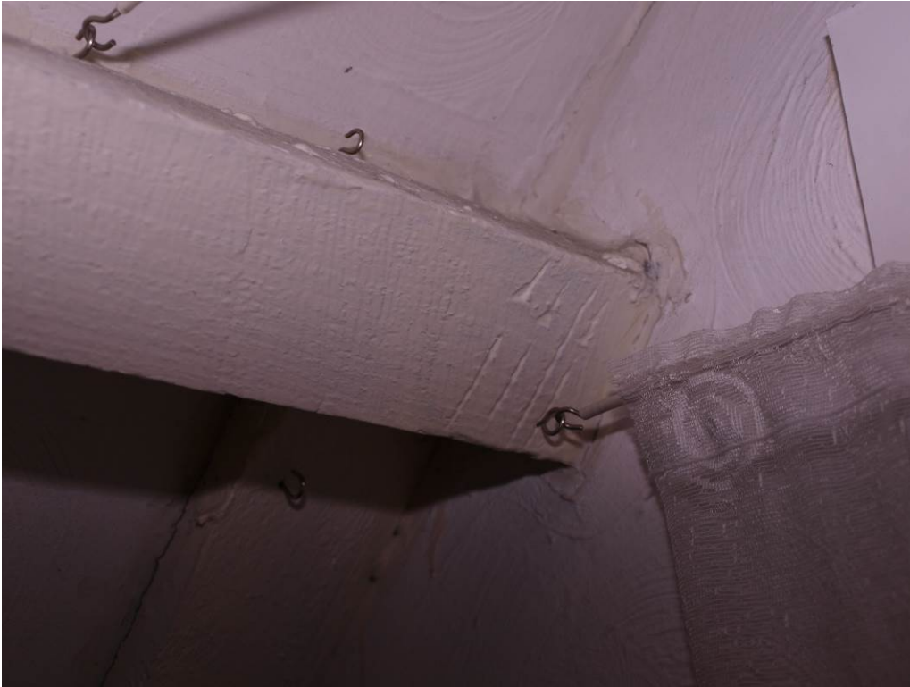
Plate 11: Carpenter's marks to purlin (18)
