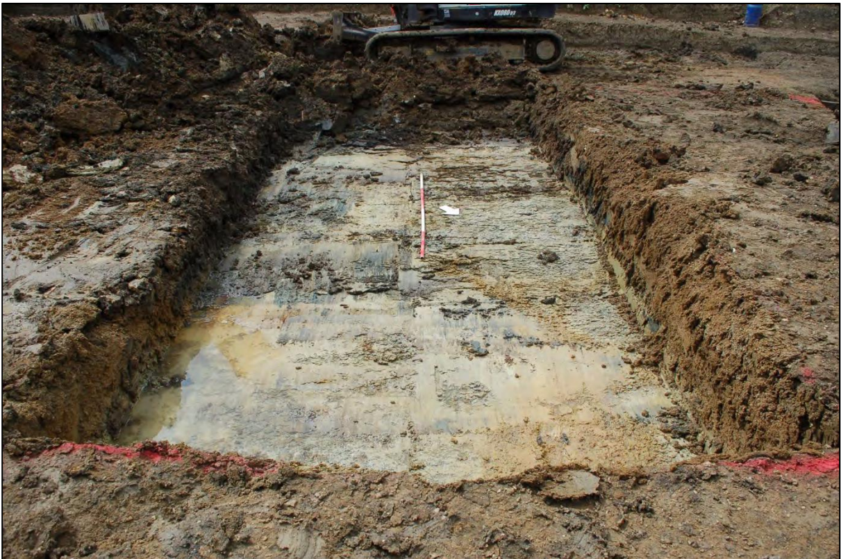
Figure 18. Attenuation Tank pit 2
