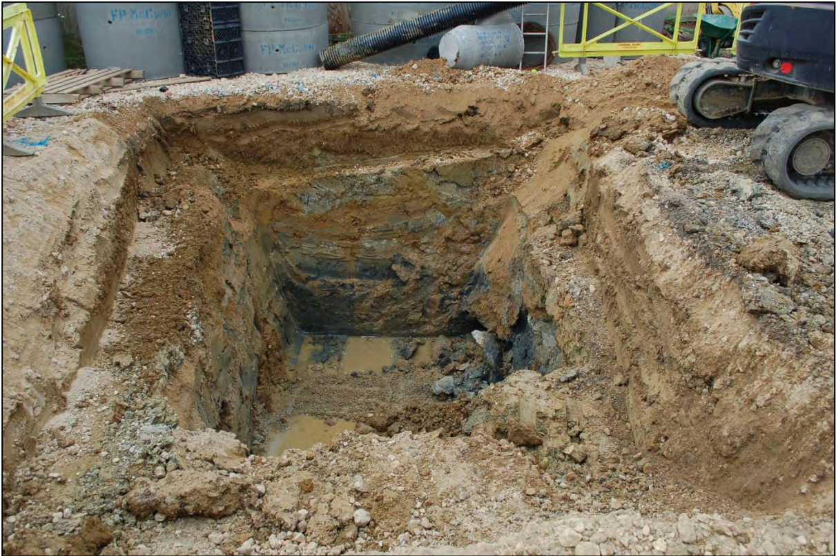
Figure 17. Attenuation Tank pit 1
