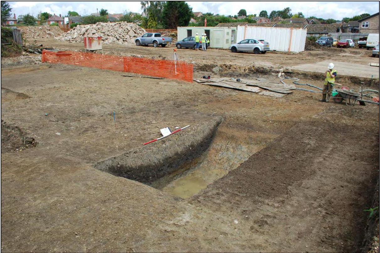
Figure 10. Pond B Segment 66, looking north (2m scale)
