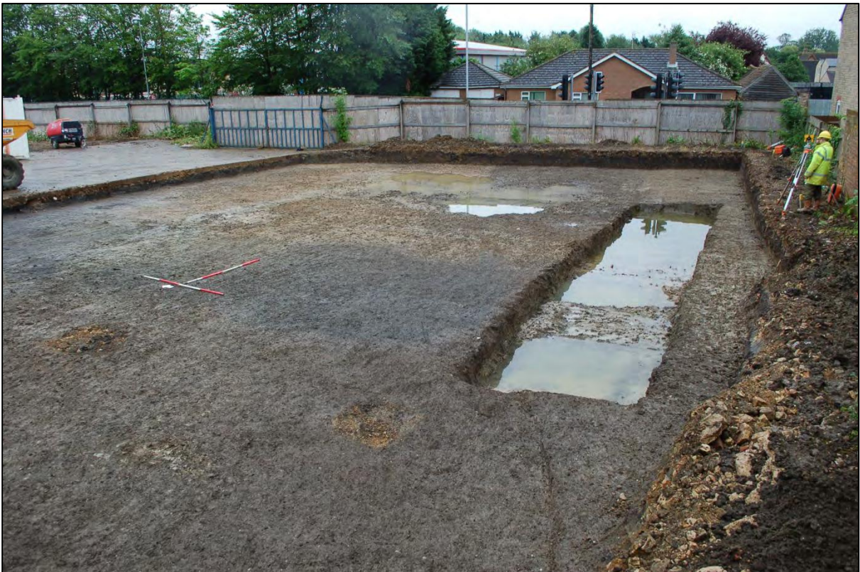
Figure 5. General site view, looking east
