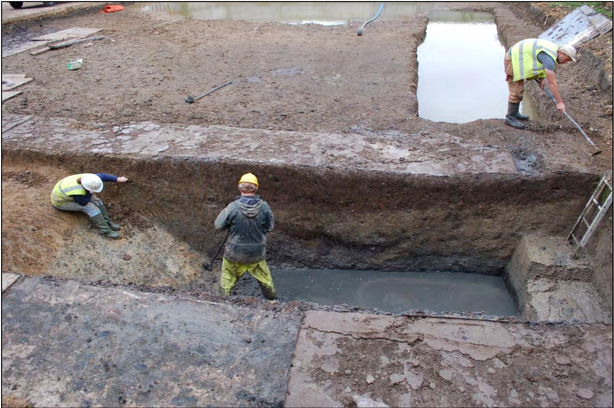
Figure 6. Pond A Segment 52, working view, looking southeast
