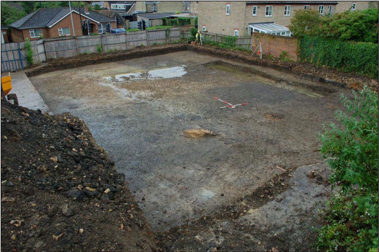
Figure 4. General site view, looking south
