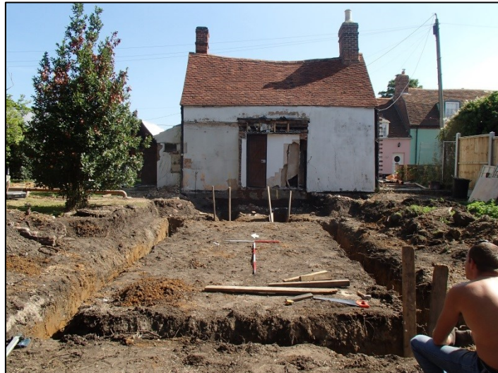
Fig. 3: Cottage extension foundation trenches, looking east (1m & 2m scale).
