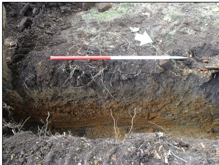
Fig. 4: Workshop/garage foundation trench, SE corner, looking west (1m scale)
