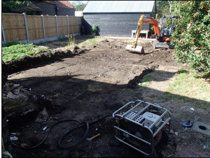
Fig. 2: Ground reduction for cottage extension, looking southwest
