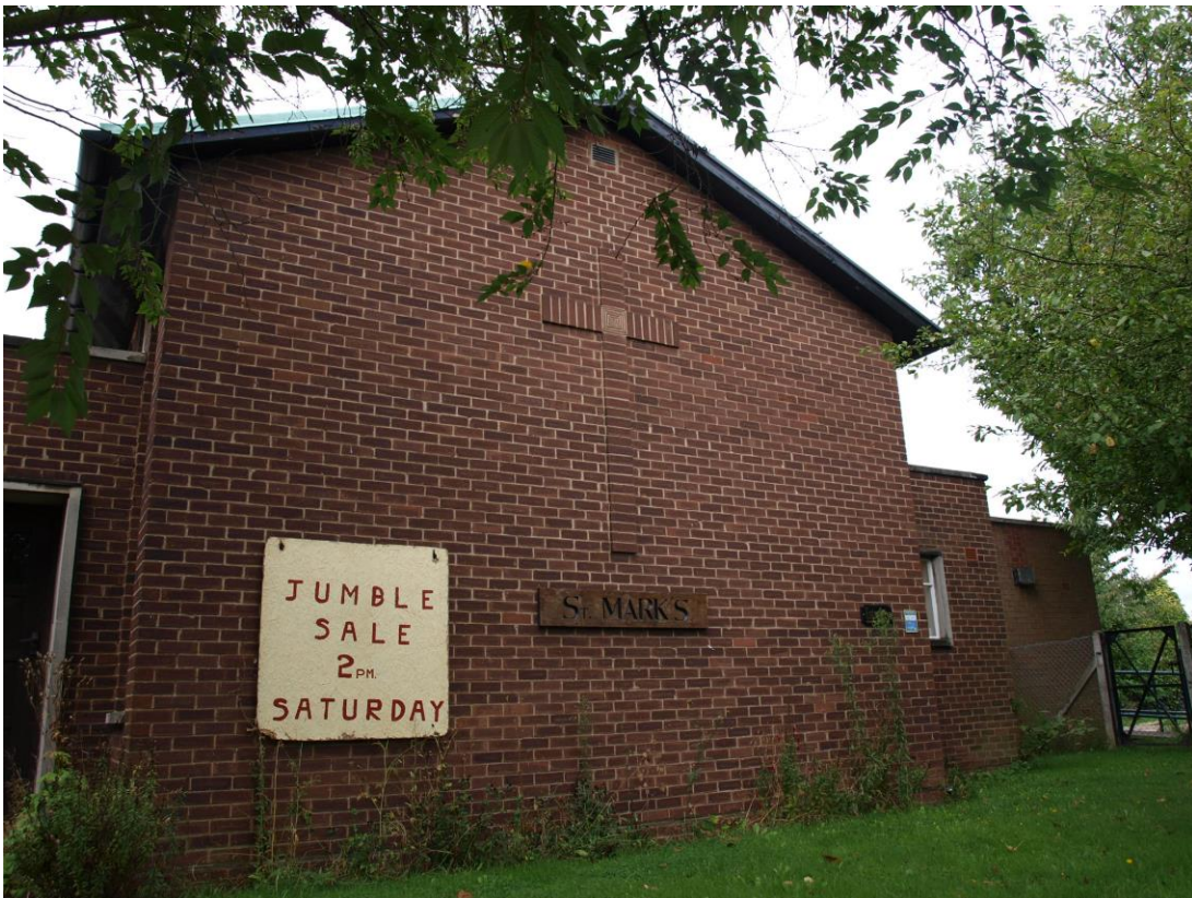
Plate 4: The east elevation of the chapel/choir and sanctuary (17).
