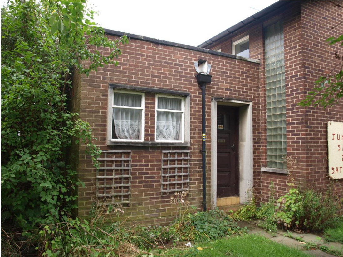
Plate 3: The east elevation of the vestry (16).
