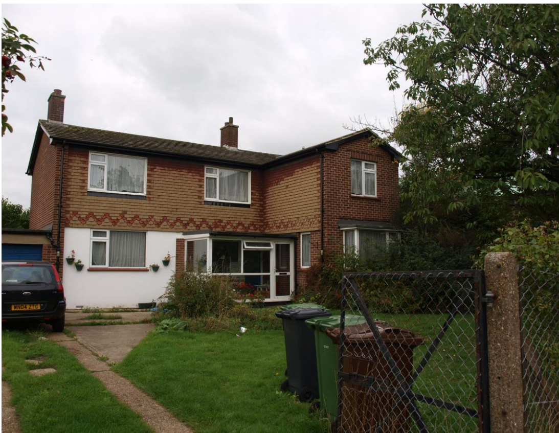
Plate 6: The Vicarage, looking north-west (13).
