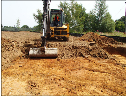
Fig. 3.1 Excavation area B looking south
