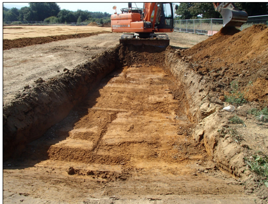
Fig. 3.2 Soakaway area 2D facing east
