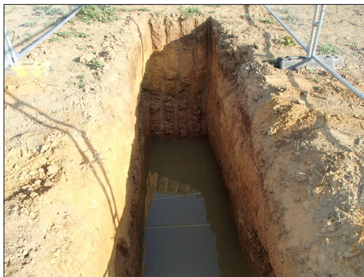
Fig. 3.3 Soakaway area 1B facing north west
