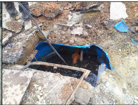
Tank 6 in watching brief phase 2, area 1
