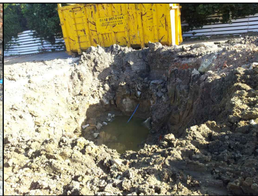
Watching brief phase 2, area 1 after removal of tank 6
