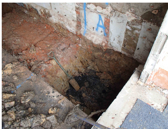
Watching brief phase 1 underpinning pit detail
