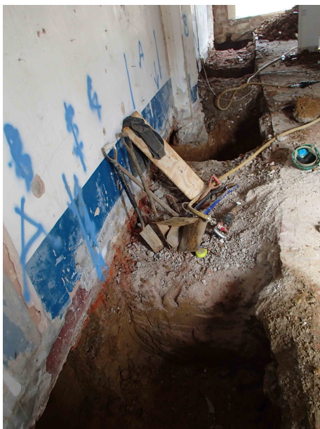
Watching brief phase 1 underpinning pits
