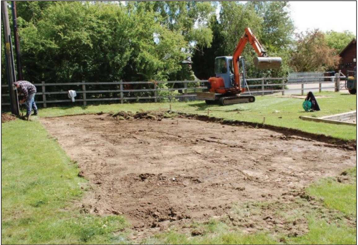
Figure 4: Garage topsoil strip looking northeast
