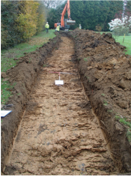
Trench 2 looking north-east
