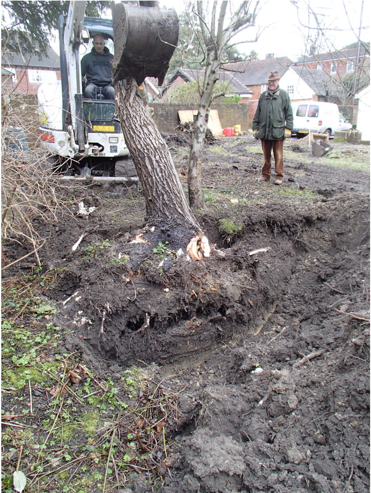
Photograph showing Phase 1 tree removal
