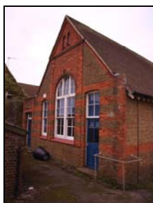
6432-10 Hall Block. Facing southwest
