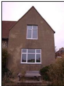
6432-04 Caretaker's Block. Facing north
