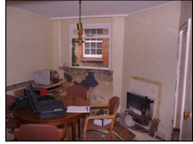
6432-39 Caretaker's Block ground. Facing north
