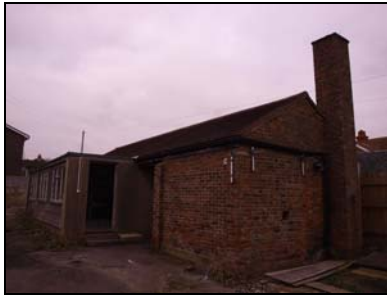
6432-13 Detached Classroom. Facing northeast
