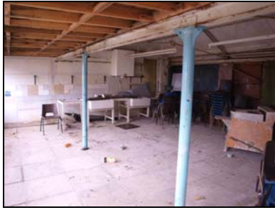
6432-16 Detached Classroom interior. Facing northeast
