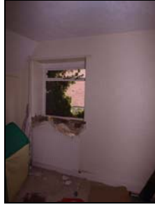
6432-50 Caretaker's Block first floor. Facing northwest
