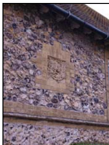
6432-07 Classroom Block shield detail. Facing east
