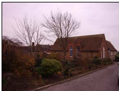
6432-08 Hall Block. Facing southeast
