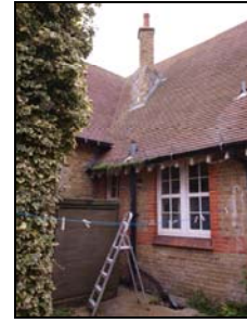
6432-42 Courtyard. Facing southwest
