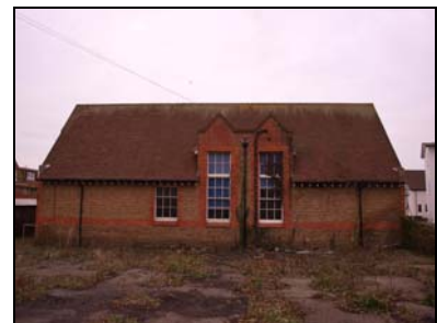
6432-09 Hall Block. Facing south
