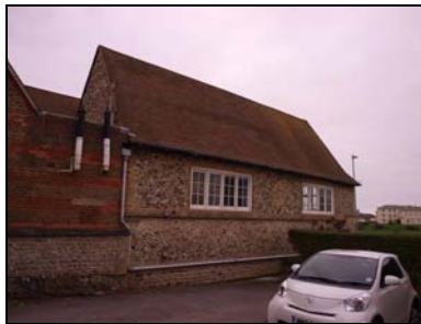
6432-05 Classroom Block. Facing southeast
