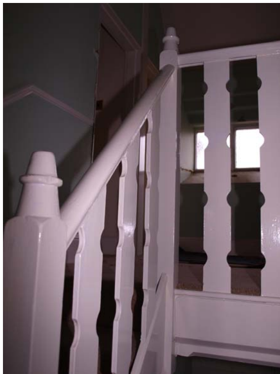
Caretaker's house, ground floor dining room
