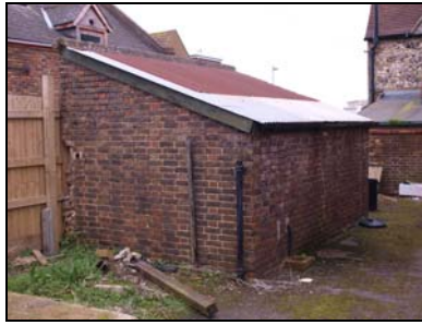
6432-14 Shed. Facing southeast
