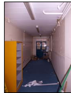
6432-21 Classroom Block corridor. Facing east
