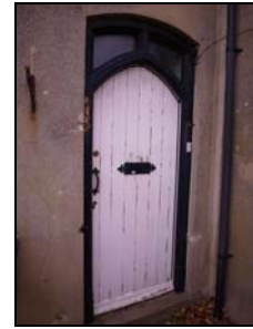
6432-03 Caretaker's Block entrance. Facing west
