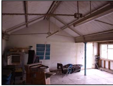
6432-17 Detached Classroom interior. Facing south
