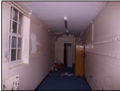
6432-22 Classroom Block corridor. Facing west
