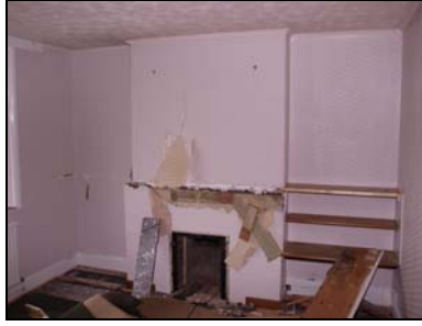
6432-38 Caretaker's Block ground. Facing southwest
