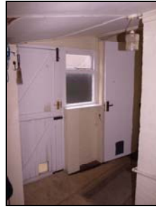
6432-41 Caretaker's Block ground. Facing southeast
