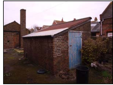
6432-15 Shed. Facing northeast
