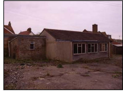
6432-18 Detached Classroom. Facing southeast
