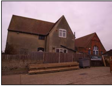
6432-01 Caretaker's Block. Facing west
