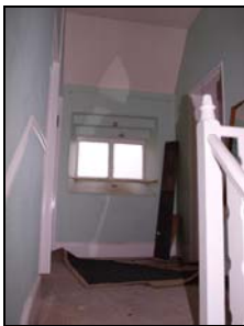
6432-46 Caretaker's Block first floor. Facing east
