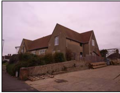
6432-02 Caretaker's Block. Facing northwest
