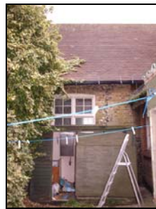
6432-44 Courtyard. Facing south
