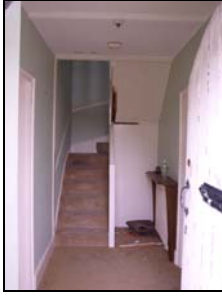
6432-37 Caretaker's Block interior. Facing west
