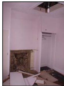
6432-47 Caretaker's Block first floor. Facing northwest
