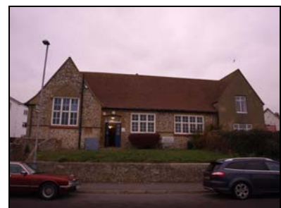
6432-12 Front Elevation. Facing north
