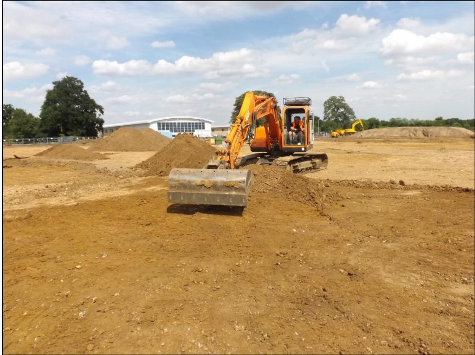
Figure 5: Site re-stripping, looking northeast
