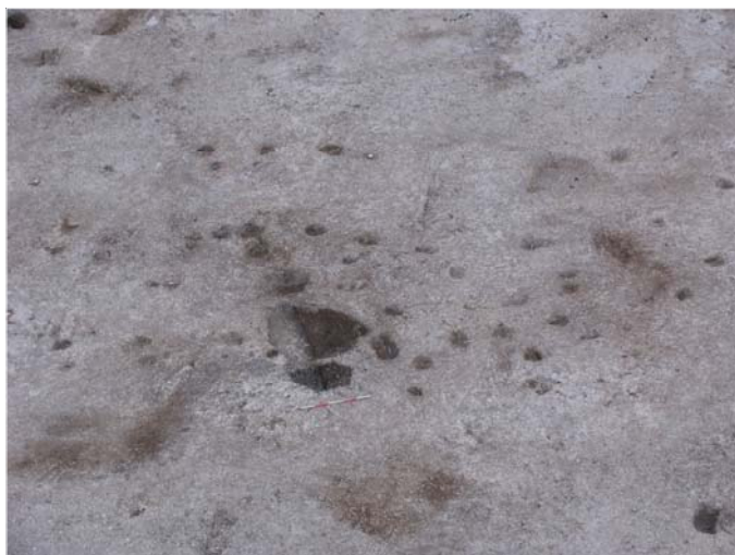
Structure S5 looking west
