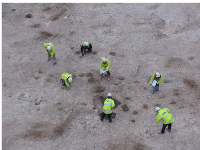
Structure S5 working shot
