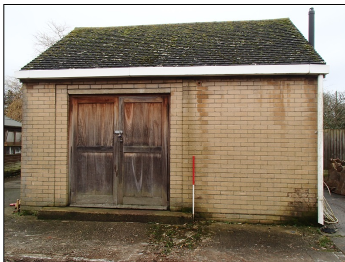
Fig. 3: Booster Station building, looking west
