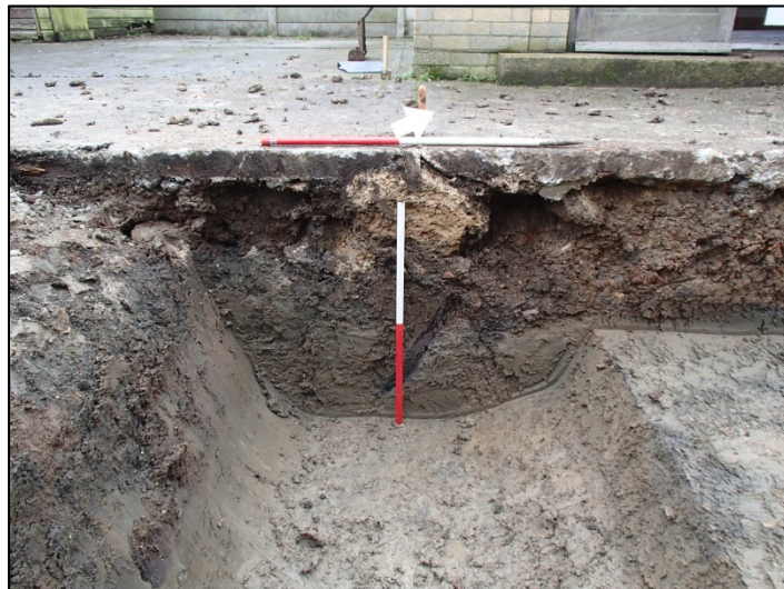
Fig. 2: Sondage at the south-west end of the trench, looking north-west
