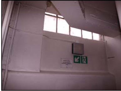
6431-076 Three Storey Block: NW Stair. Facing NW
