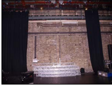
6431-026 Studio 1 Exposed Wall. Facing NW
