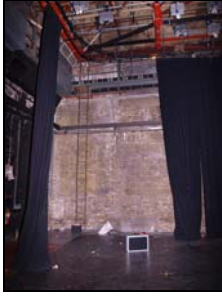
6431-025 Studio 1 Exposed Wall. Facing NW
