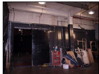
6431-024 Studio 1 Gwynnes' Factory Entrance. Facing NE
