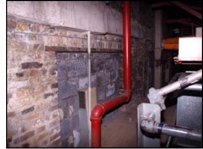
6431-030 Studio 1 Blocked Window. Facing W
