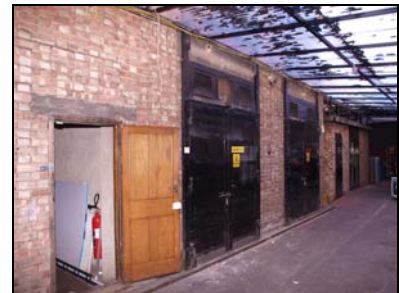
6431-006 Generator Block. Facing S
