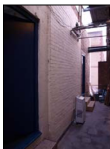
6431-095 Crisp Road Block/Three Storey Block Walkway. Facing E
