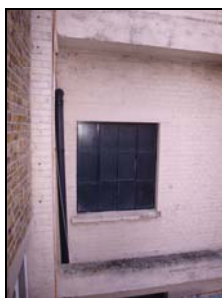
6431-214 Cinema: SE External Elevation Window. Facing NW
