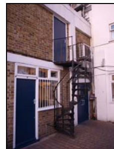
6431-132 Thameside Block. Facing N
