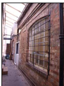
6431-094 Crisp Road Block/Three Storey Block Walkway. Facing SE
