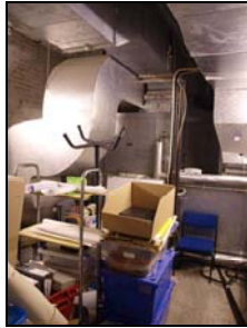
6431-088 Cinema: First Floor Plant Room. Facing W
