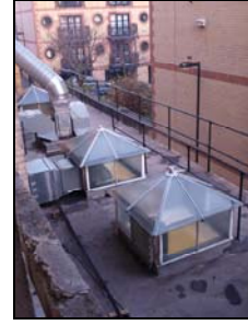
6431-123 Roof of Southeastern Block. Facing E
