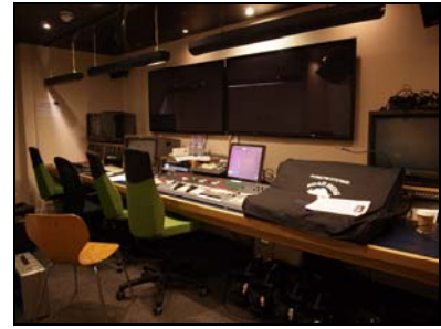
6431-099 Studio 2: Lighting Gallery. Facing S
