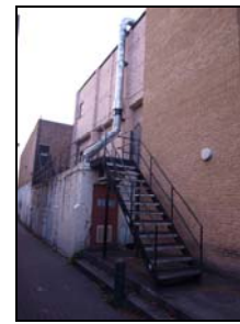
6431-225 Cinema and Lift Shaft. Facing W
