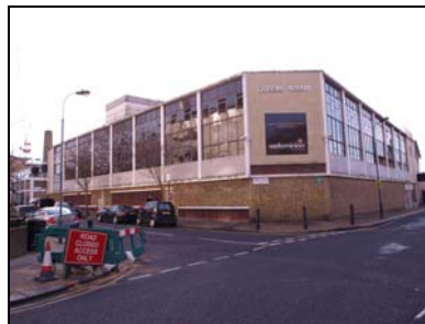
6431-239 Queens Wharf. Facing S
