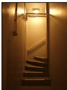
6431-166 Southeastern Block: NE Stair. Facing NE
