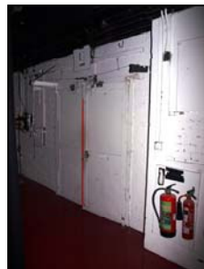
6431-068 Studio 2: Doorway to Three Storey Block. Facing N
