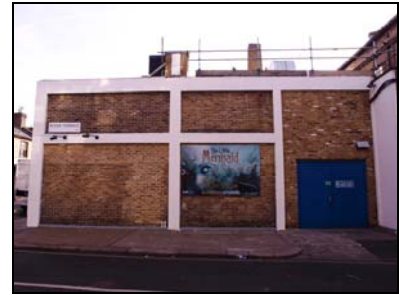
6431-003 Crisp Road Block. Facing SE
