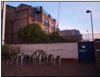
6431-127 River Terrace: Boundary Wall. Facing SE
