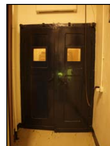
6431-084 Three Storey Block: Doorway to Cinema. Facing SW
