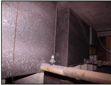
6431-208 Three Storey Block: Roofspace Tanks. Facing W
