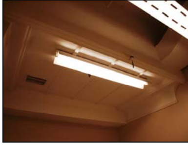
6431-074 Studio 2 Dressing Room: Ceiling Detail. Facing E
