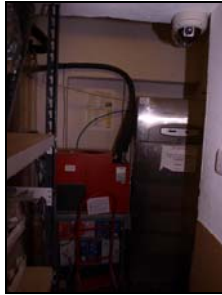
6431-160 Public Bar Store Room. Facing NW
