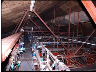
6431-184 Studio 1: Roof Trusses and Access Gantry. Facing SW
