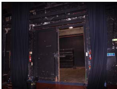
6431-023 Studio 1 Gwynnes' Factory Entrance. Facing SW
