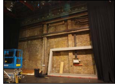
6431-186 Studio 1: Exposed Wall. Facing NW
