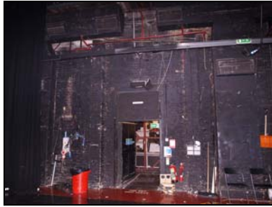
6431-065 Studio 2: Gwynnes' Factory Internal Wall. Facing SE
