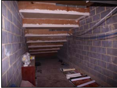
6431-100 Cinema: Void Beneath Banked Seating. Facing SW
