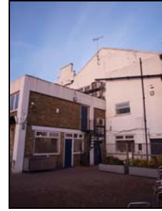
6431-126 Thameside Block. Facing N
