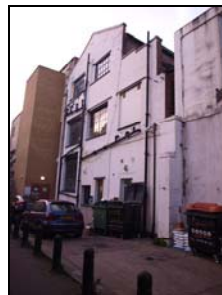
6431-224 Three Storey Block. Facing W
