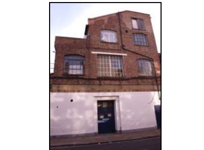
6431-009 Three Storey Block. Facing SE
