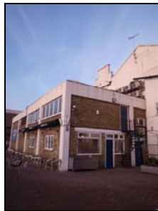
6431-128 Thameside Block. Facing NW
