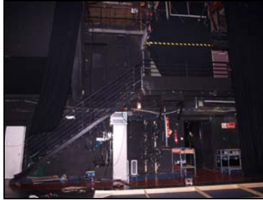
6431-185 Studio 1: Stair to Production Suite. Facing SE
