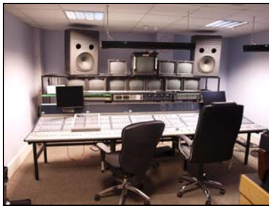
6431-175 Studio 1: Production Control Room. Facing SE
