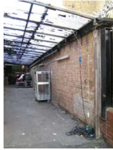
6431-242 Boundary wall between Queens Wharf and Riverside Studios. Facing SW
