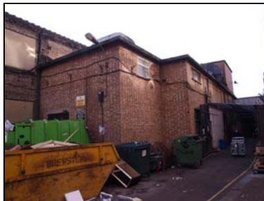
6431-005 Generator Block. Facing S
