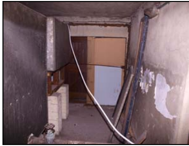
6431-209 Three Storey Block: Roofspace. Facing NW
