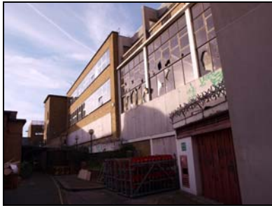
6431-241 Queens Wharf. Facing SW
