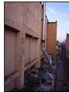
6431-213 Cinema: SE External Elevation. Facing NE
