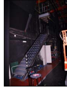
6431-027 Studio 1: Stair to Production Suite. Facing S
