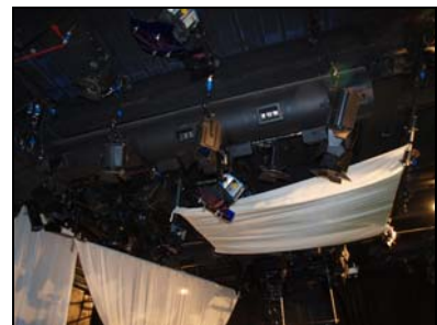
6431-048 Studio 3 Lighting Grid. Facing NW
