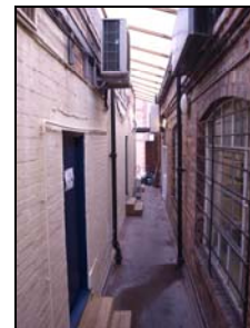
6431-093 Crisp Road Block/Three Storey Block Walkway. Facing SE
