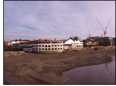
6431-234 Queens Wharf. Facing NE
