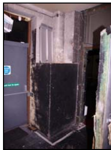
6431-056 Generator Block: Abutting Gwynnes' Factory. Facing E
