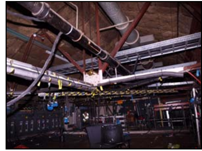
6431-039 Studio 1: Second Floor Balcony. Facing S
