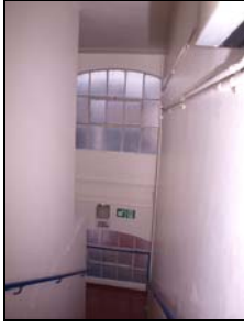
6431-229 Three Storey Block: NW Stair. Facing NW
