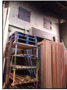
6431-194 Generator Block: Ventillation Louvre. Facing NE
