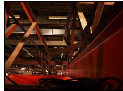
6431-201 Studio 2: Lighting Grid Bowstring Truss. Facing SE
