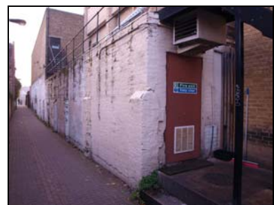
6431-228 SE Boundary Wall. Facing SW
