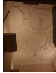
6431-138 Studio 2 Dressing Room: Ceiling Detail. Facing SW
