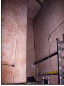
6431-121 Cinema: Store Behind Screen. Facing SE
