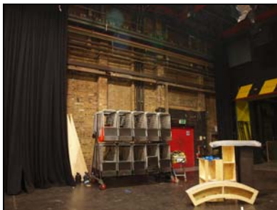
6431-187 Studio 1: Exposed Wall. Facing N
