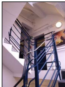
6431-092 Three Storey Block: SE Stair. Facing N
