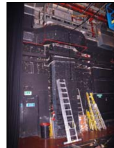
6431-021 Studio 1 Box Truss Pier. Facing SW
