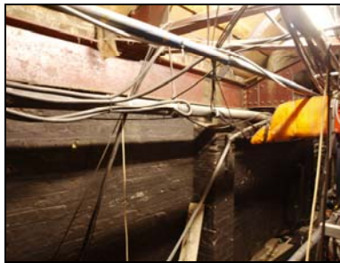
6431-200 Studio 2: Lighting Grid Bowstring Truss. Facing N
