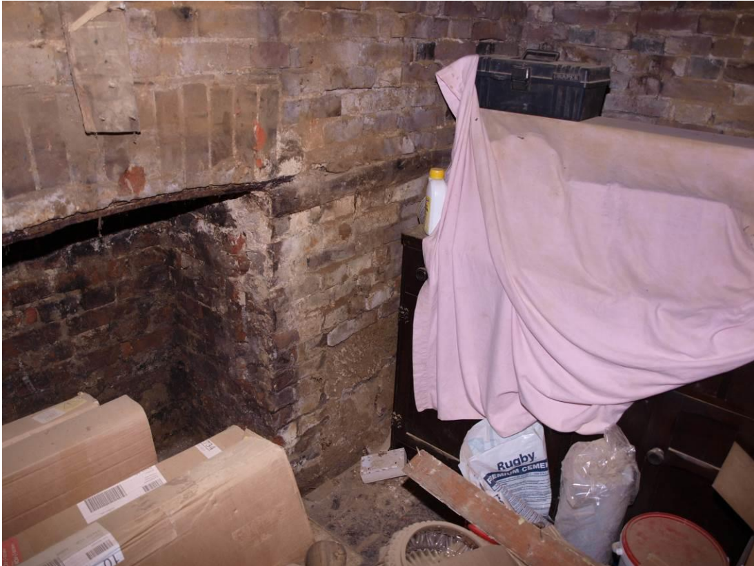
Plate 5: Detail of west wall of Living Room 02 (7)
