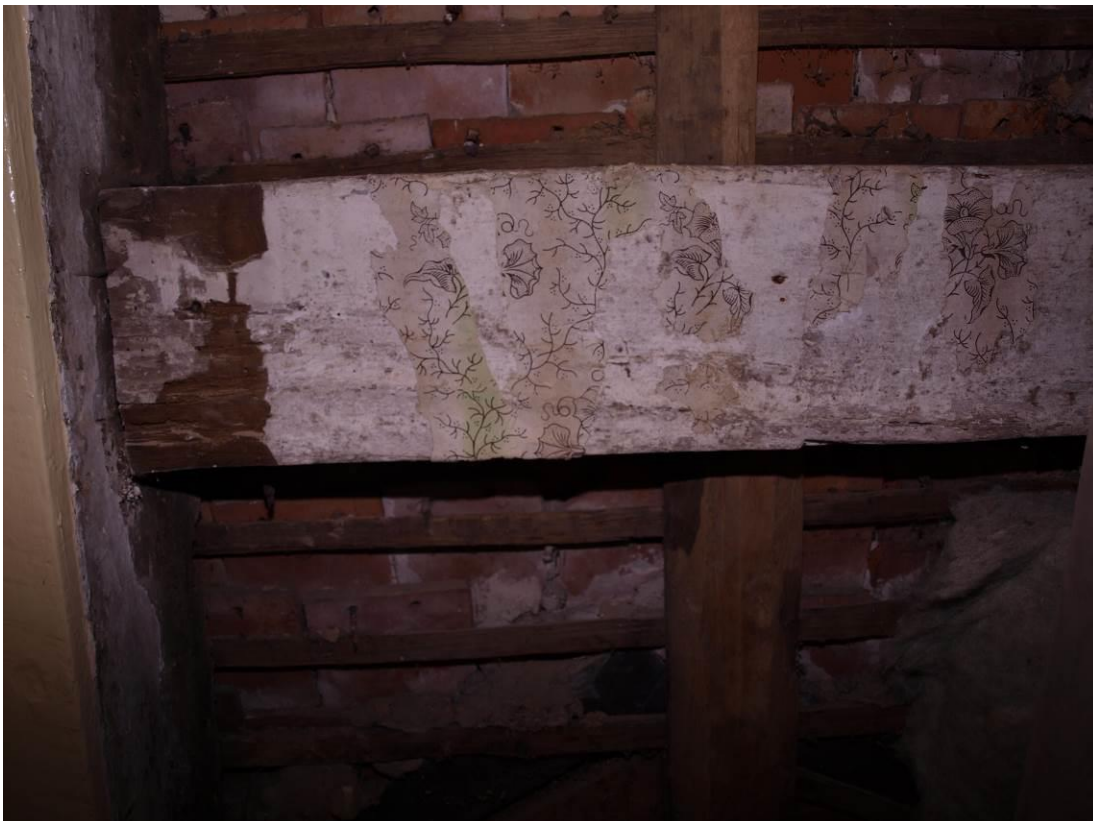
Plate 10: Midrail to north wall of Bedroom 02 (25)
