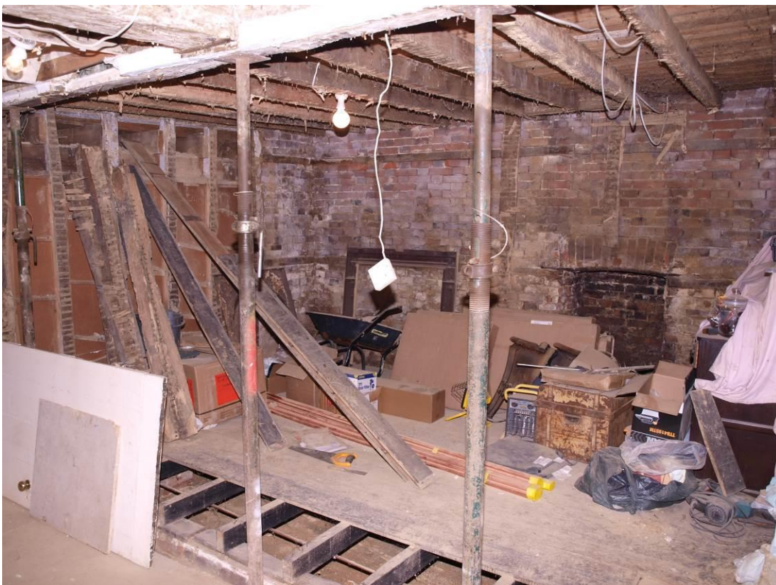
Plate 4: Ceiling to Living Room 02
