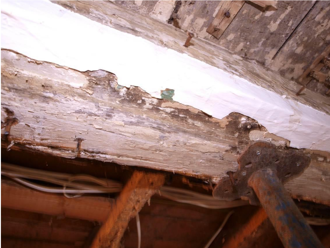
Plate 7: Stave mortices in tie beam of partition wall (13)
