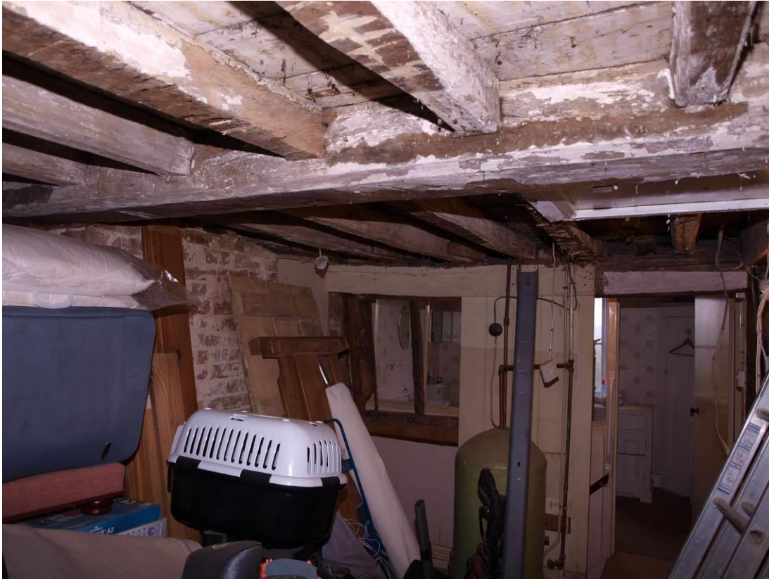
Plate 9: Ceiling to Bedroom 02 (26)
