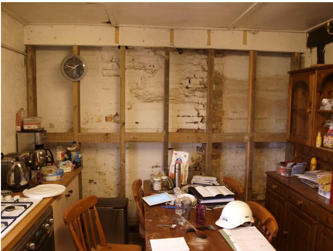
Plate 8: Site of former chimney breast on west kitchen wall (15)
