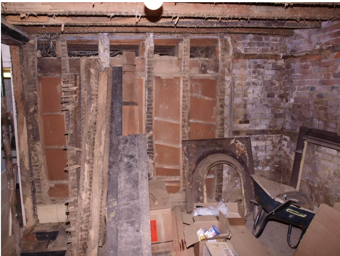
Plate 6: South wall of Living Room 02 (6)
