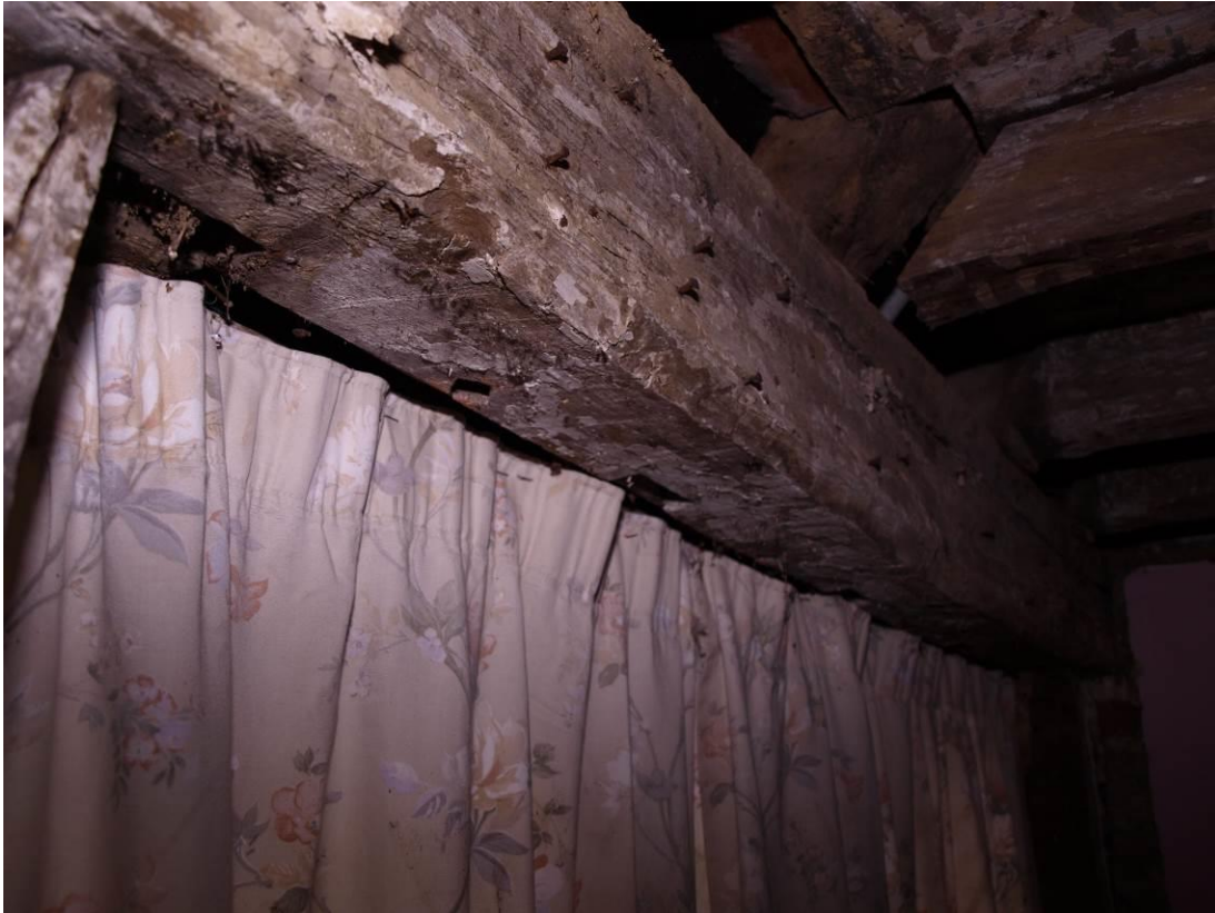
Plate 11: Head of window opening on north wall of Bedroom 02 (24)
