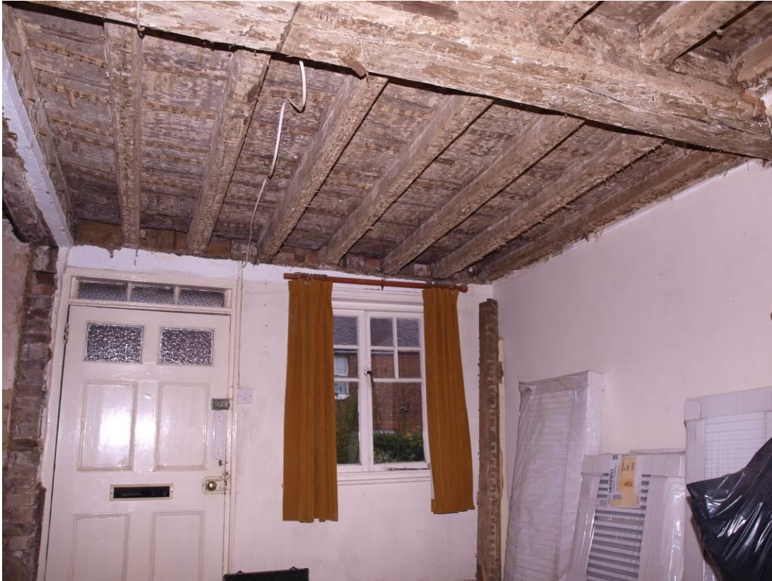
Plate 1: Ceiling to Living Room 01 (3)
