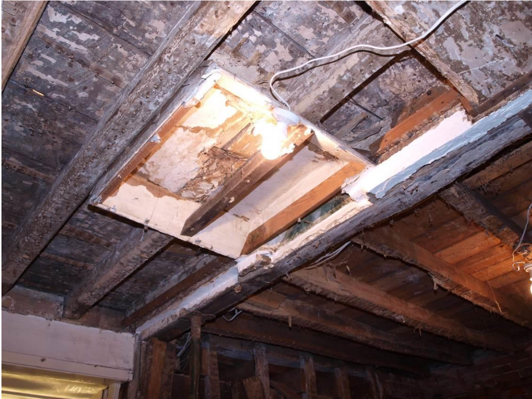
Plate 3: Feature in ceiling of Living Room 01, with concave mortice behind, and possible evidence of doorway head to left (10)
