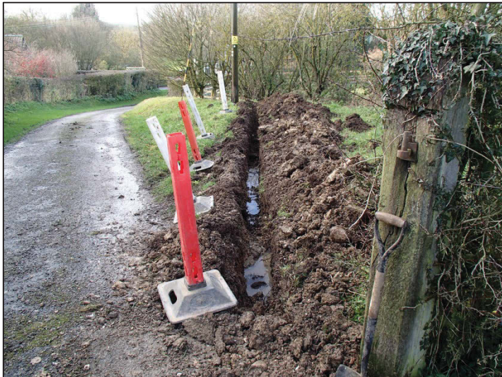
Figure 3. Trench running west from churchyard gateway, looking west
