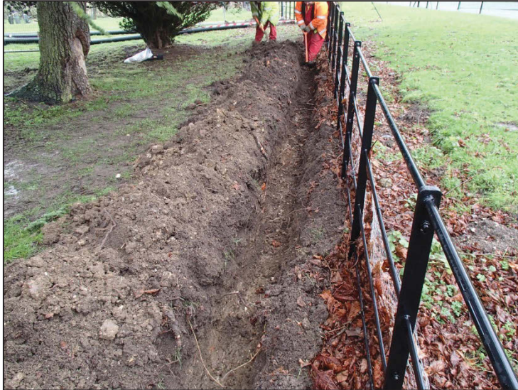
Figure 2. Trench along eastern boundary, looking north
