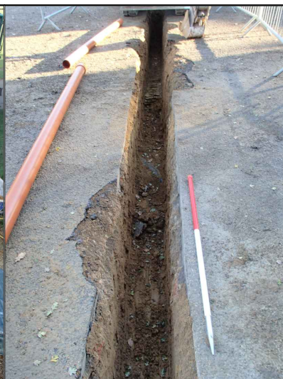
Trench 1 west end, looking west
