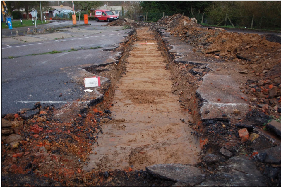
Fig. 7. Trench 6, looking north-east. 1m scale bars
