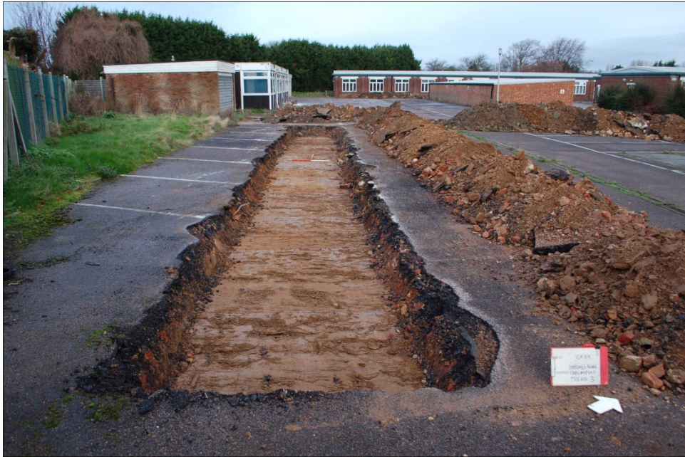
Fig. 4. Trench 3, looking north-west. 1m scale bars
