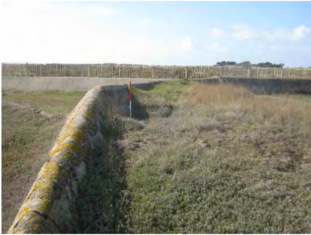
Plate 7: Area 3 northern retaining wall
