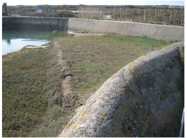
Plate 8: Area 3 northern retaining wall
