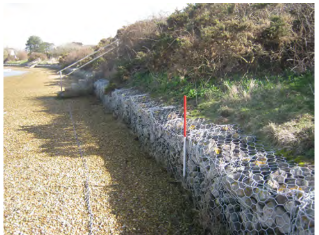
Plate 12: Area 4 gabion, looking north-east
