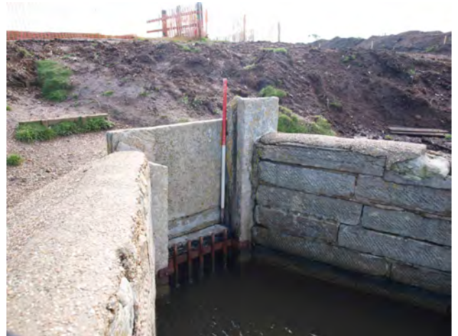
Plate 4: The stone built sluice with recessed detail in sides of slab above a narrow platform against which the iron grille has been fixed
