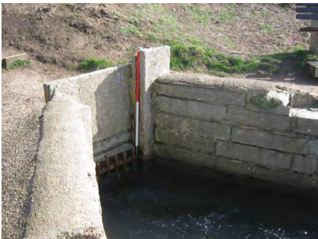
Plate 11: Area 3 inner sluice gate detail
