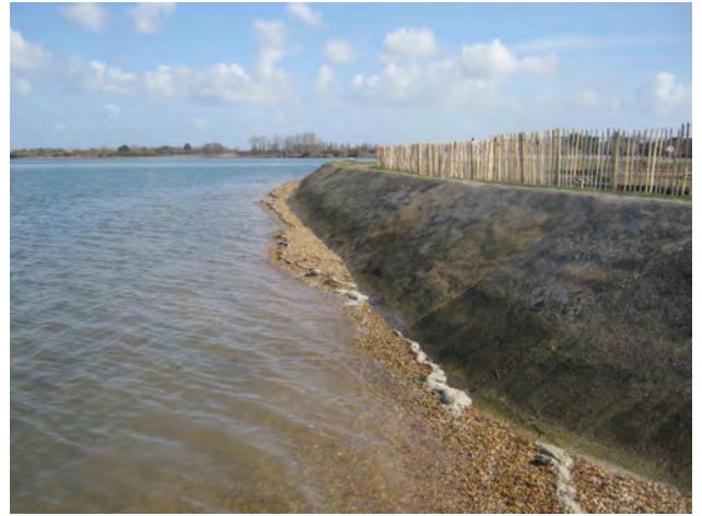
Plate 2: Area 2 looking, north-east
