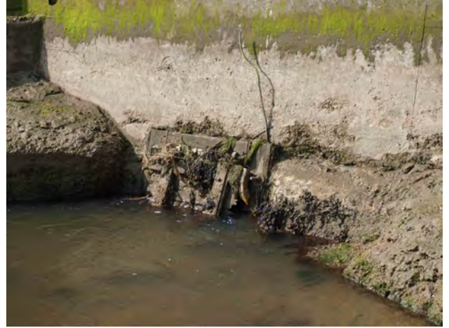
Plate 2: Detail of the culvert mouth on the Harbour side, with timber framed grille
