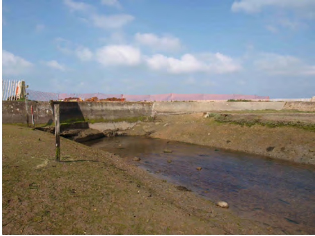
Plate 1: The retaining wall and culvert mouth on the Harbour side
