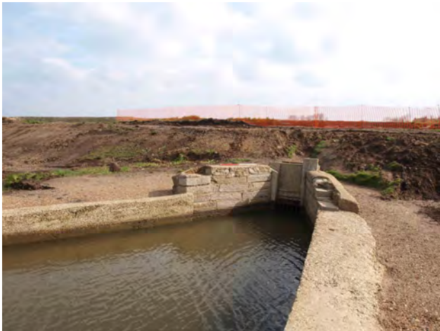
Plate 3: The sluice on the Marsh side
