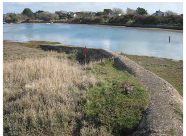
Plate 6: Area 3 northern retaining wall, looking north-east
