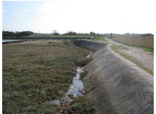
Plate 4: Area 2 looking, south-east
