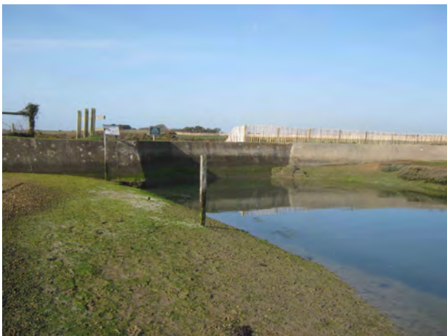
Plate 5: Area 3 sluice, looking south-west
