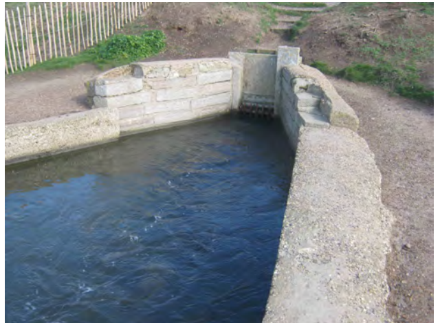
Plate 10: Area 3, inner sluice gate
