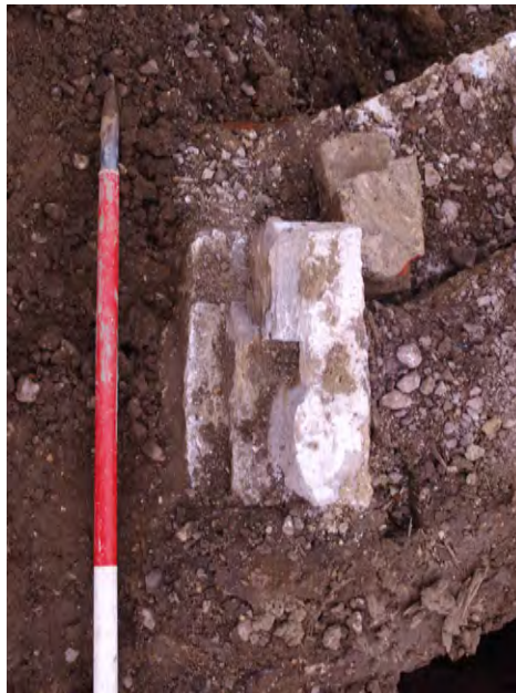
Plate 8: The north west corner of the former masonry eastern sluice gate with socket detail matching that still in situ for the west sluice gate
