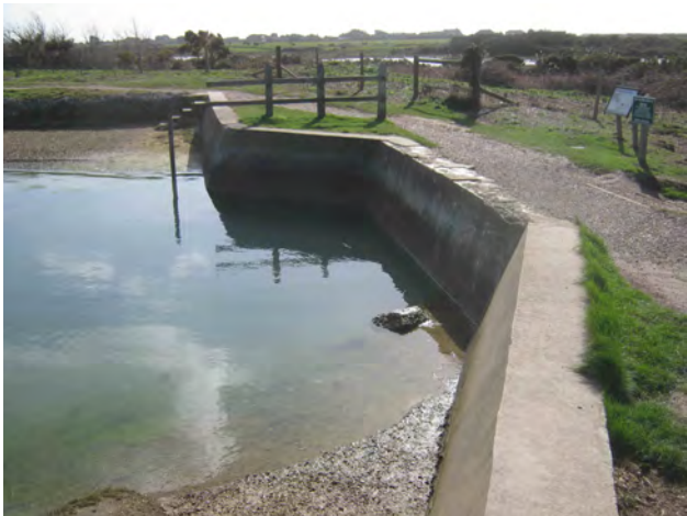
Plate 9: Area 3, looking south-east
