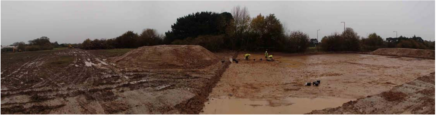
Area 1 under excavation
