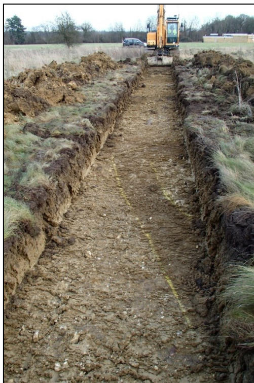
Figure 17: Enclosure ditch [127], trench 35, looking east
