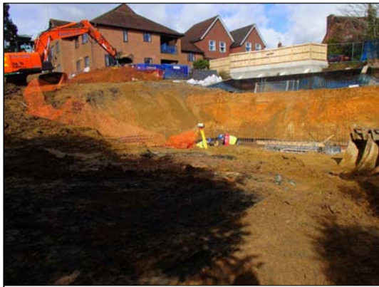
Fig. 4.1 The footprint excavations looking northwest
