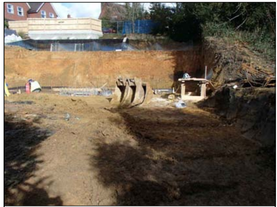
Fig. 4.2 The footprint excavations looking north
