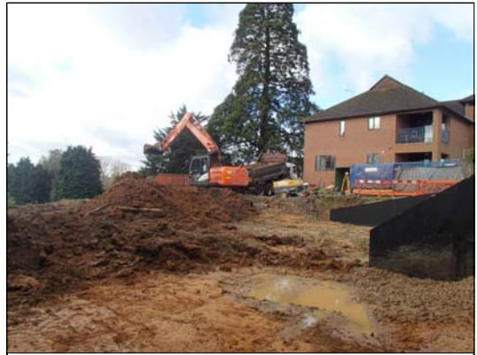
Fig. 4.3 The footprint excavations looking south-west
