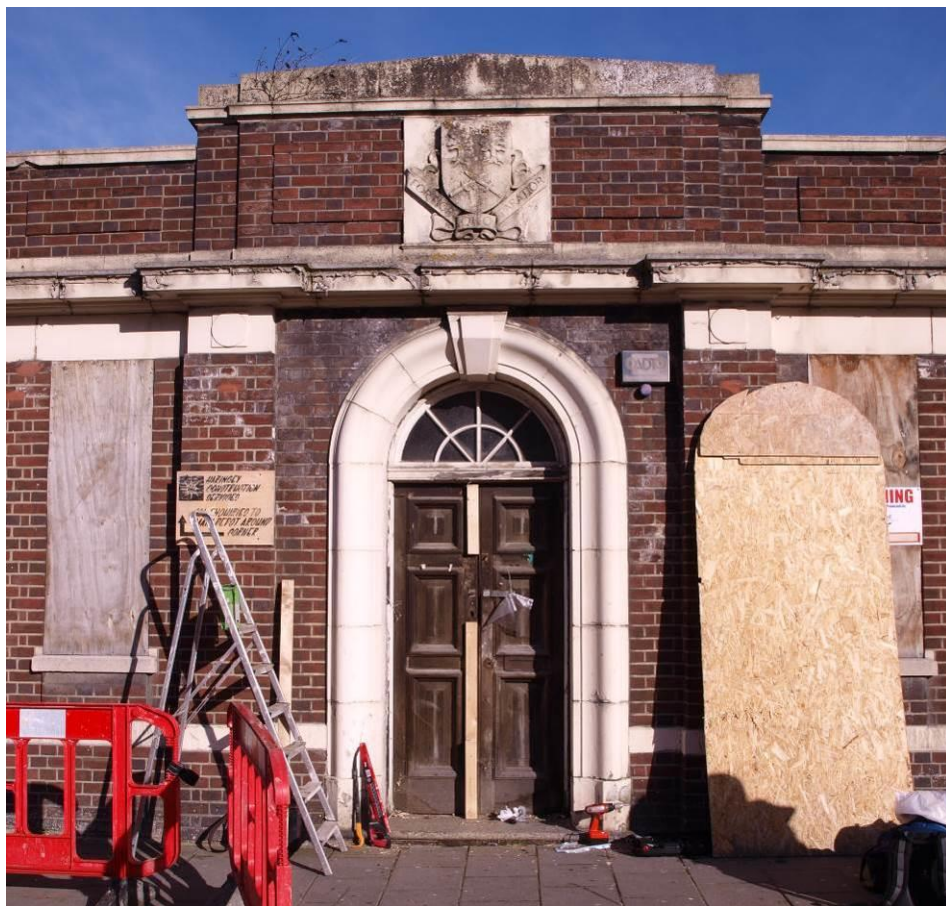
Plate 11 The central doorway in the principal (south) elevation from the south
