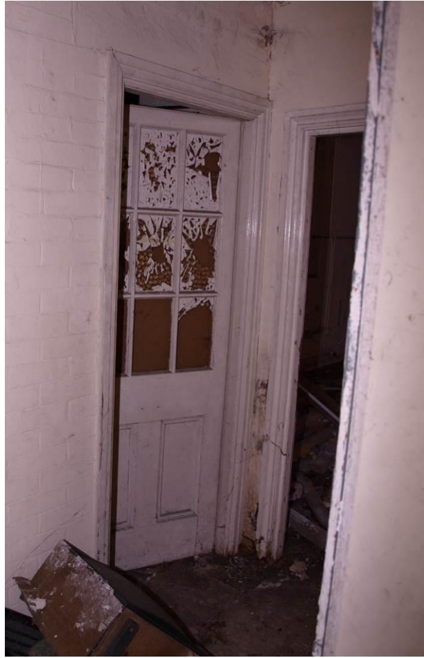
Plate 16 Door leading into Room 2. Photo from the north-east
