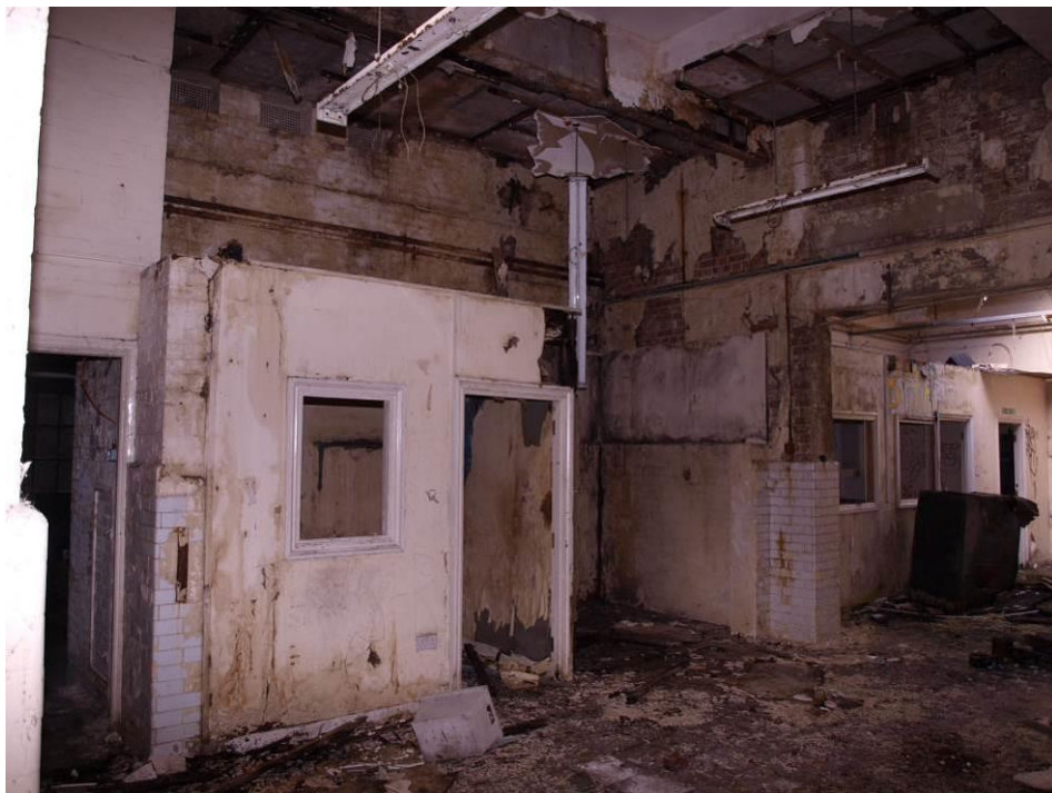
Plate 19 Room 9 from the south-west, showing Rooms 12 and 13 to the right
