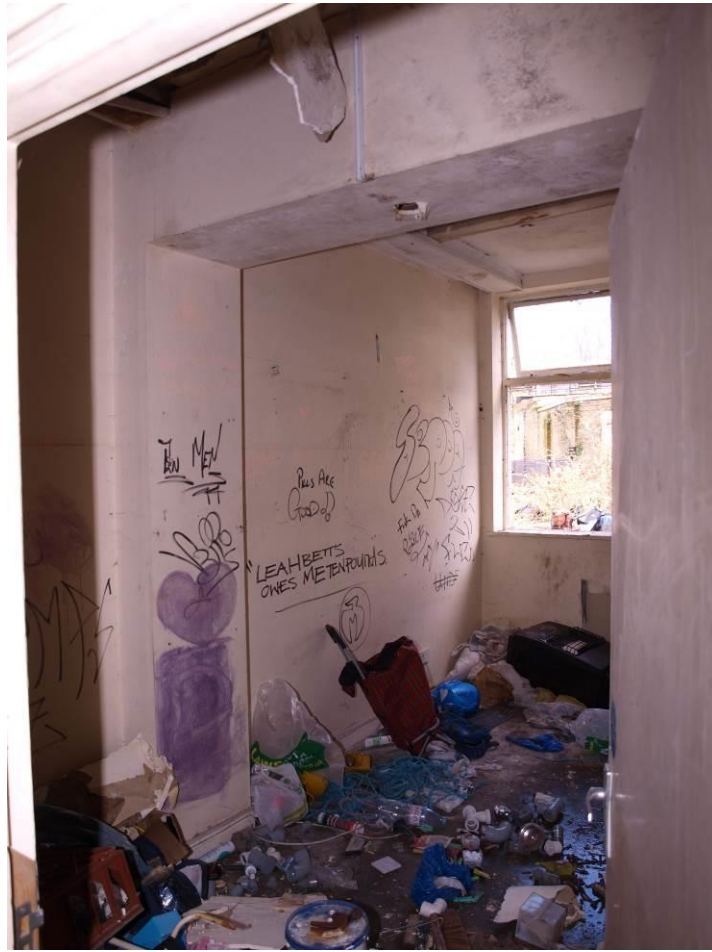
Plate 24 Room 20 from the south-west showing the wall which has been cut to create the room
