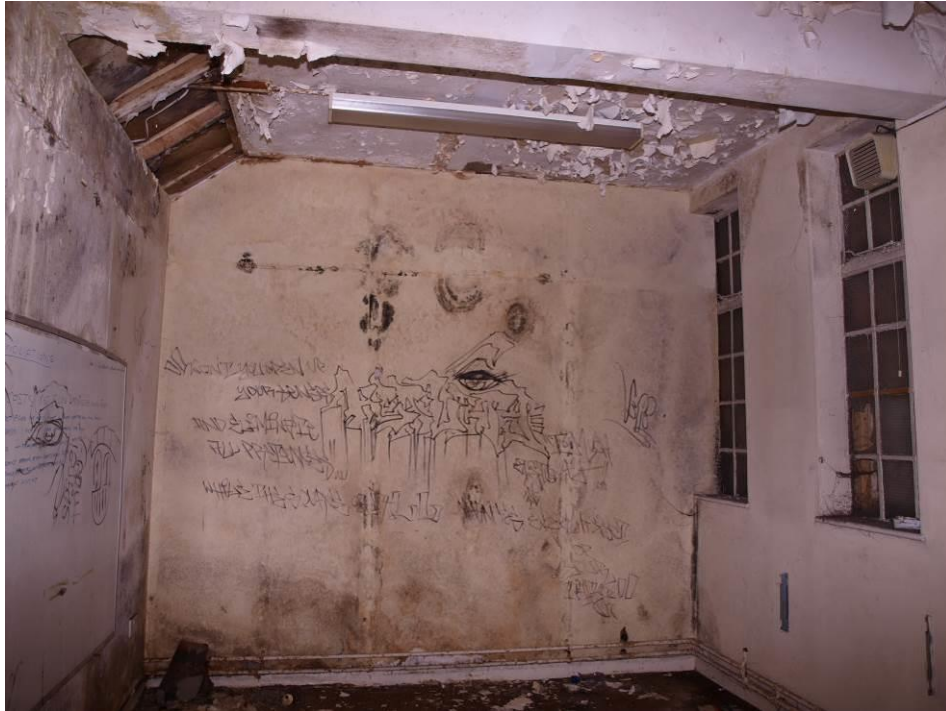
Plate 18 Room 4 from the west showing the skeling blocking the roof lantern
