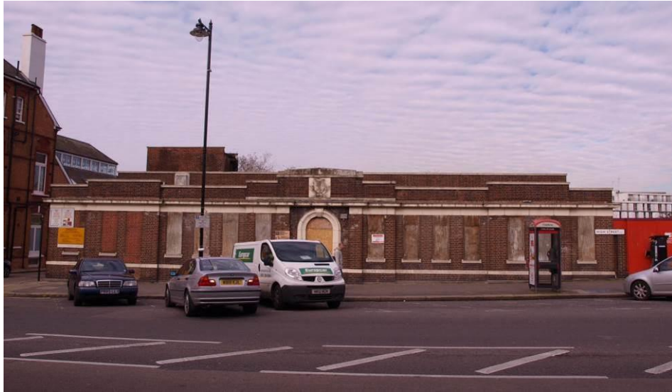
Plate 10 The principal (south) elevation of the former public baths and wash-house from the south
