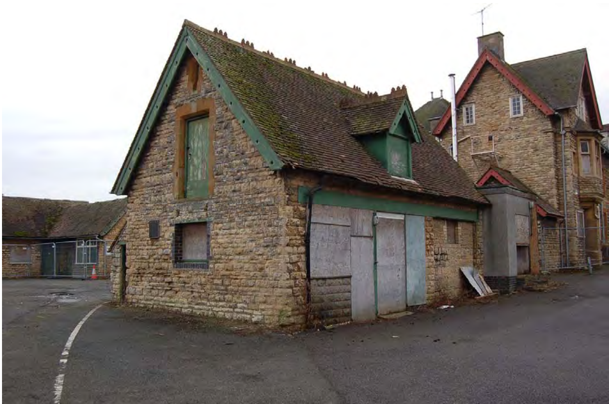
Plate 74: Mortuary (Building 3) viewed to south, with laundry/workshop (Building 4) to left and north-east end of Building 1 to right
