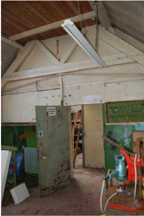
Plate 85: Roof truss in workshop G02 and corridor G03, viewed to south-west
