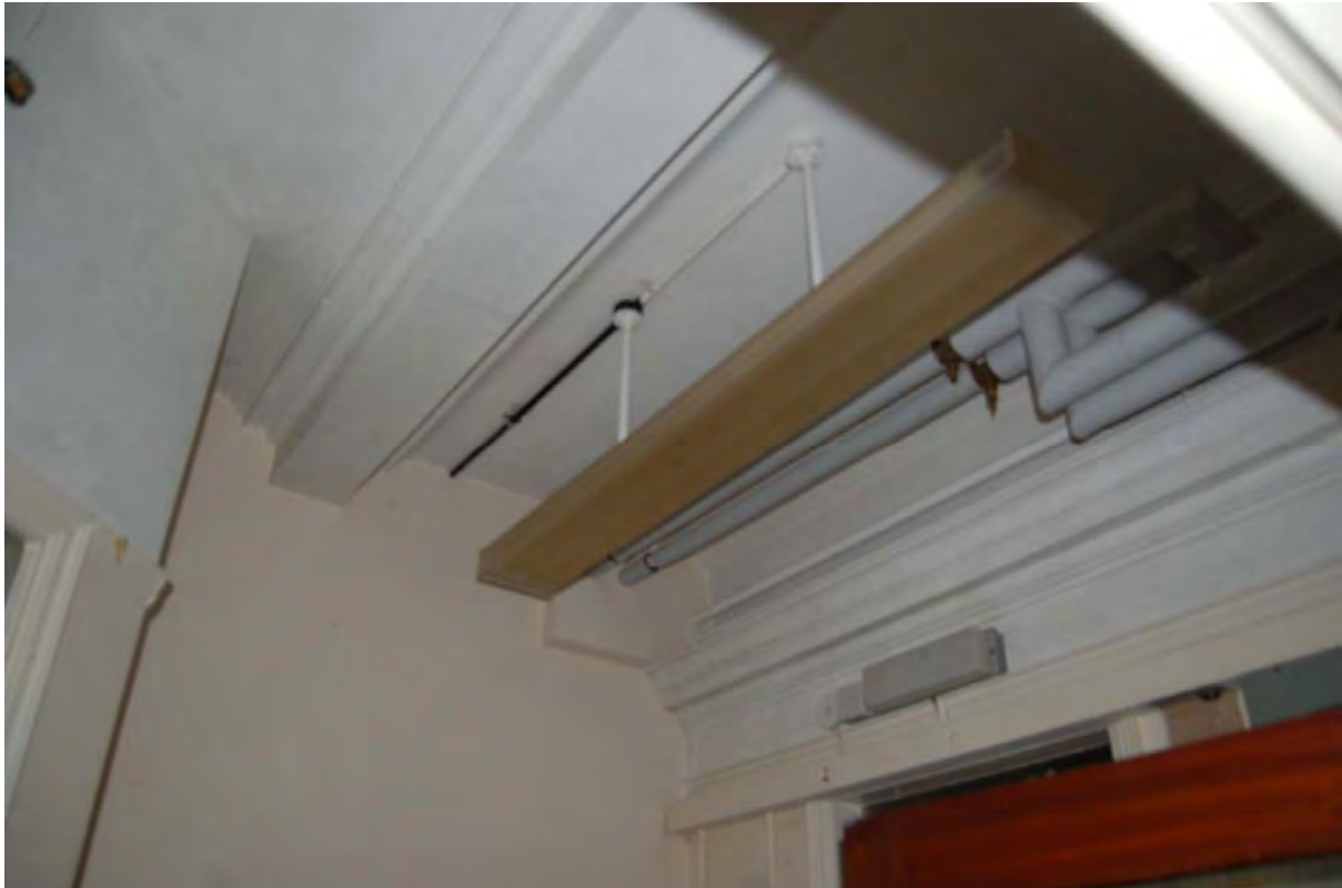
Plate 19: Detail of moulded beam and cornice in room G04 of Building 1
