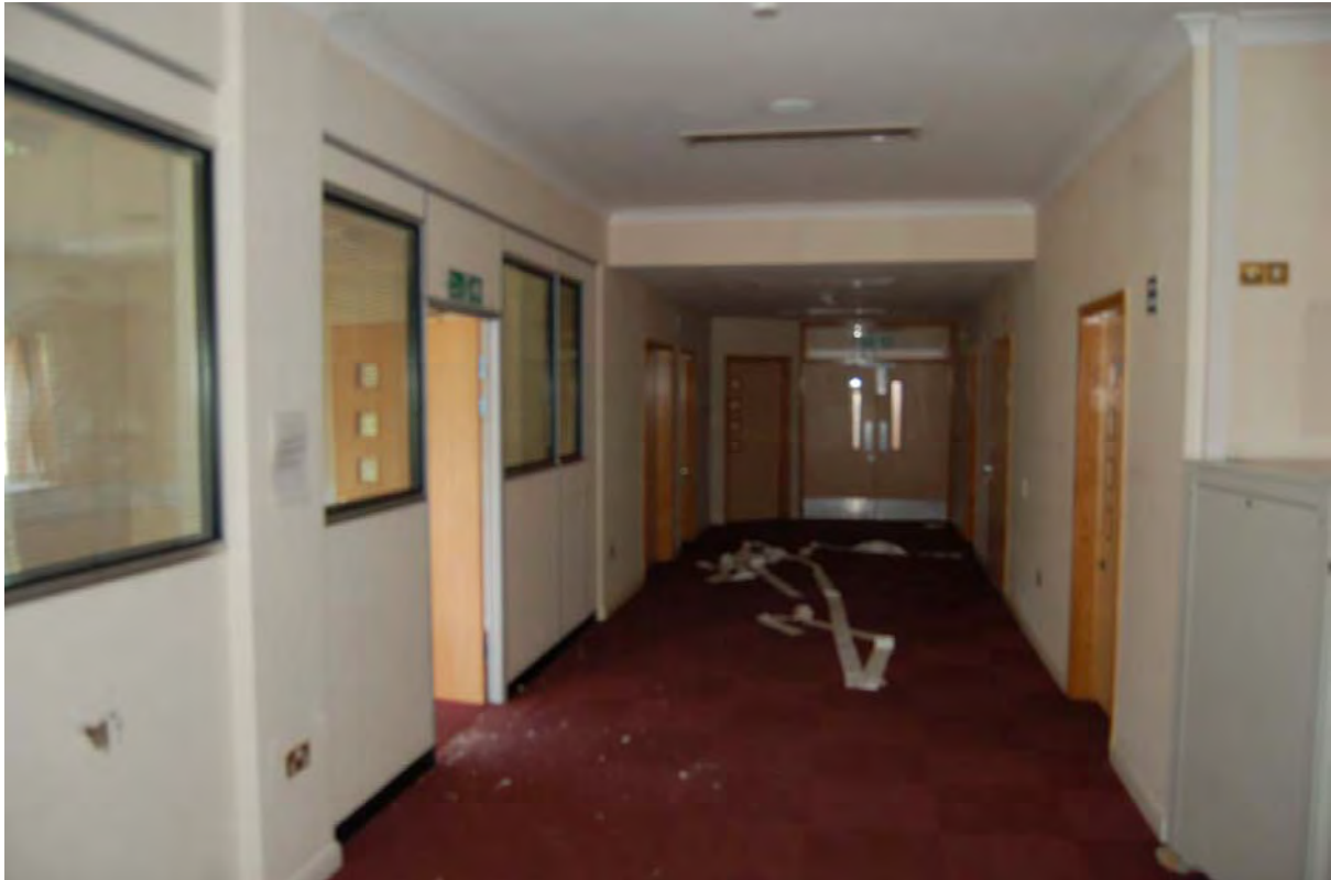
Plate 117: Main corridor inside Hargrave House Annexe (Building 11), viewed to south
