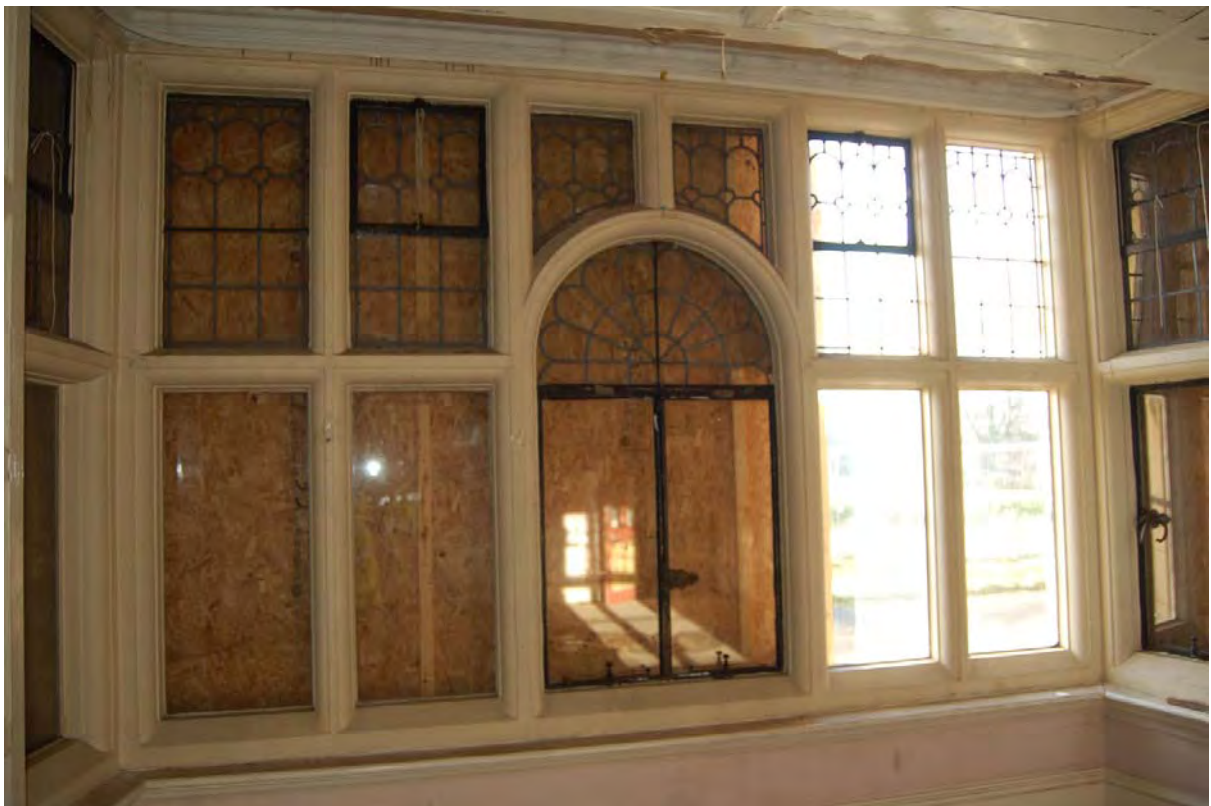
Plate 26: Leaded window detail in Room G15 viewed to south-west
