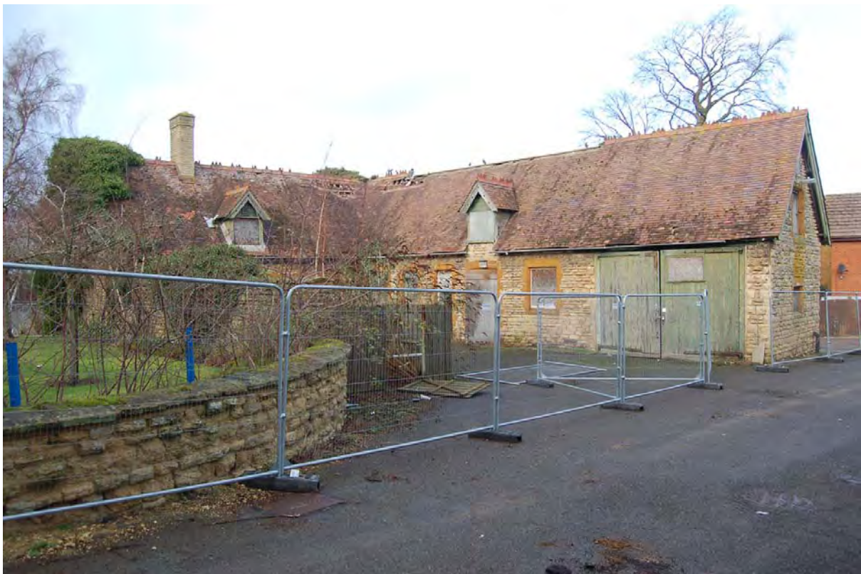
Plate 62: Stable block (Building 2) viewed to north
