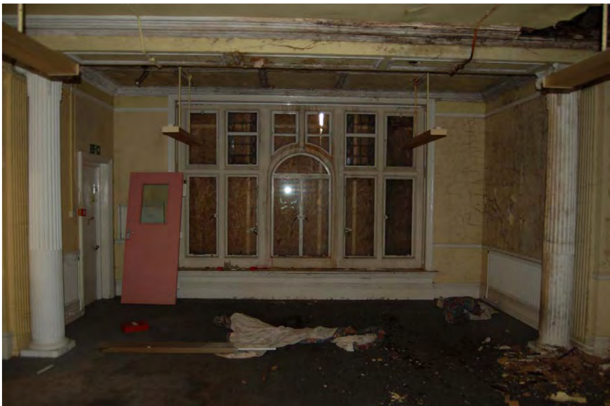
Plate 22: Room G12 in Building 1, viewed to south-west showing columns and window
