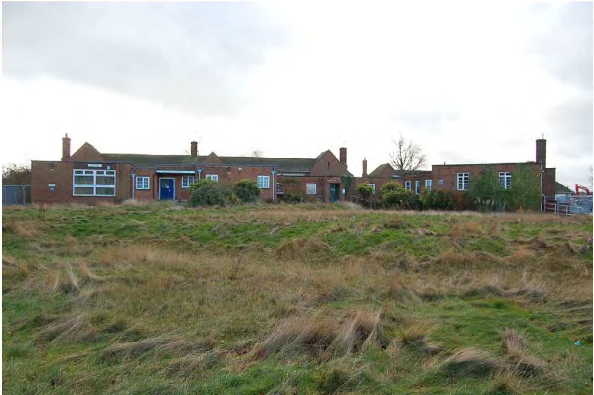
Plate 93: Ward block (Building 6) and kitchen block (Building 9) viewed to south
