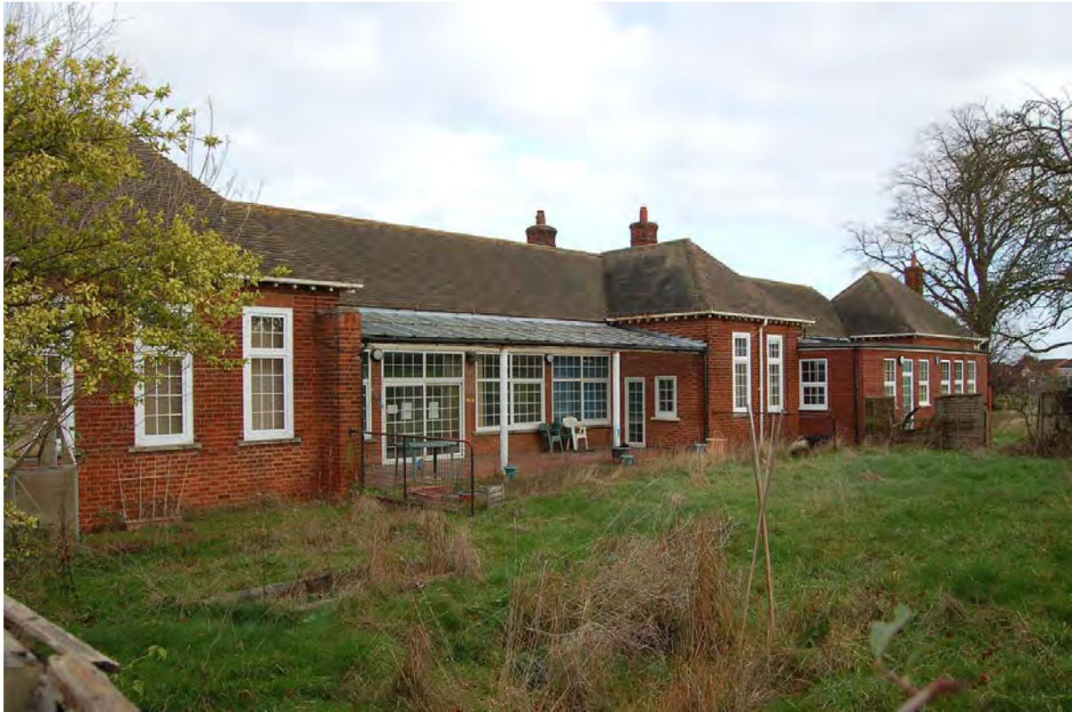
Plate 101: Main elevation of ward block (Building 8), viewed to north-east
