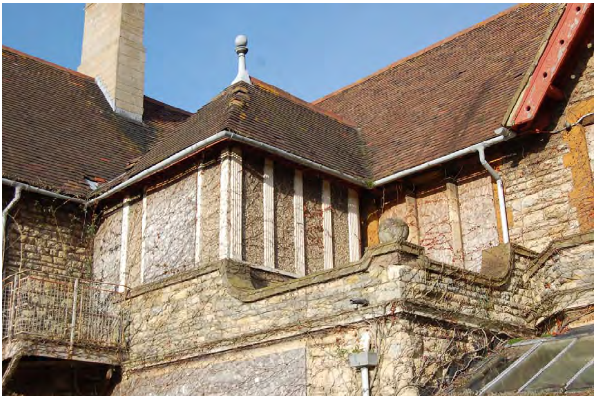
Plate 12: Detail of turret on south-west elevation of Building 1
