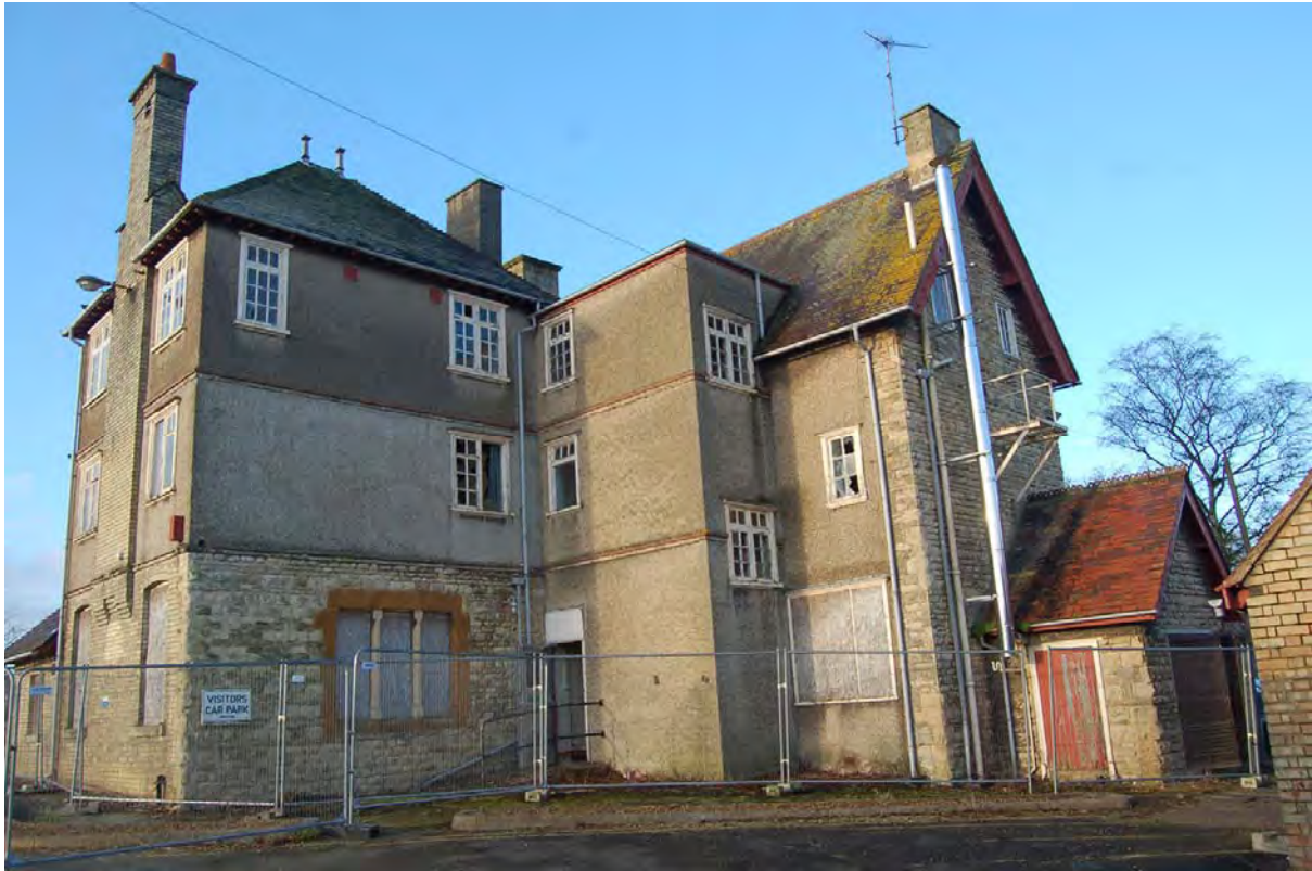
Plate 3: Building 1 viewed to east
