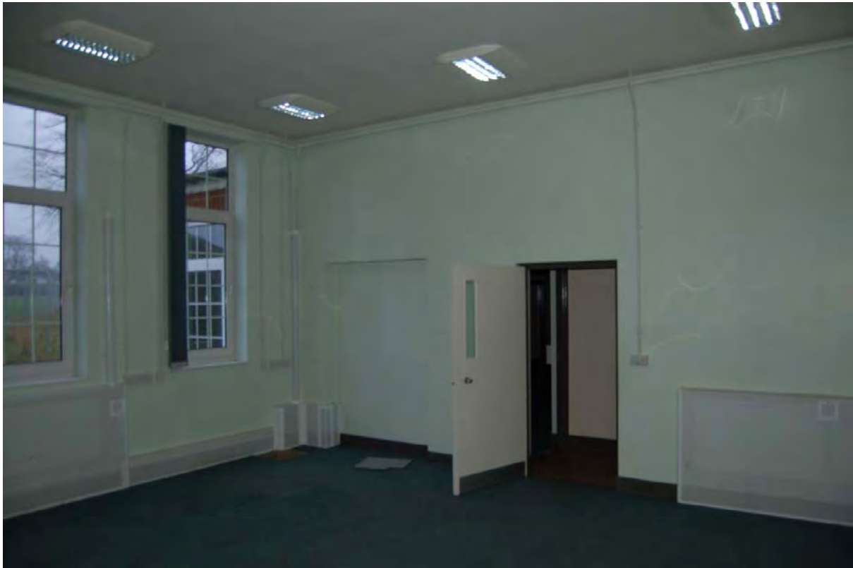
Plate 99: Former east ward of ward block (Building 7), with blocked doorway onto veranda, viewed to south-west
