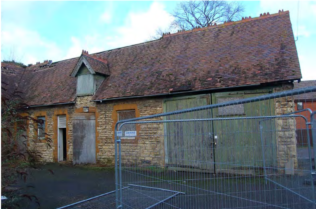
Plate 63: South-east range of stable block (Building 2) viewed to north-east
