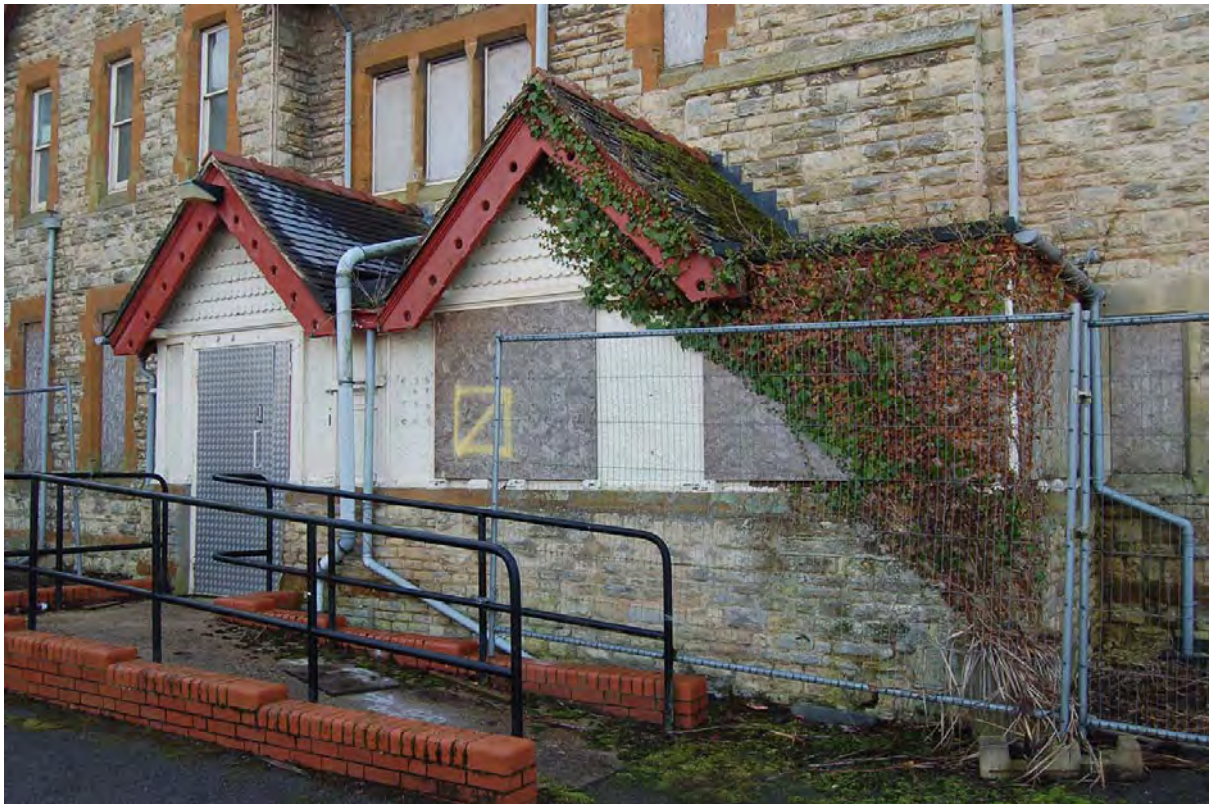
Plate 6: 1907 Entrance porches on north-east elevation of Building 1
