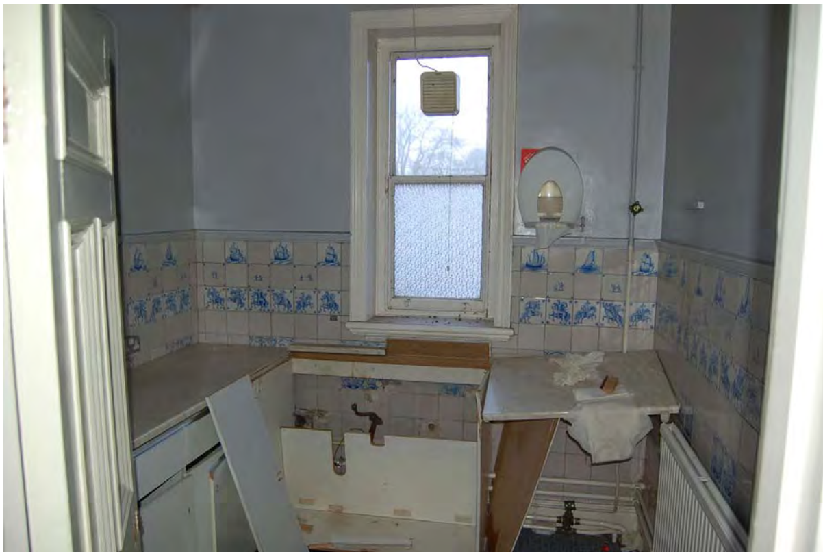
Plate 50: Staff kitchen F32 in Building 1, viewed to north-west
