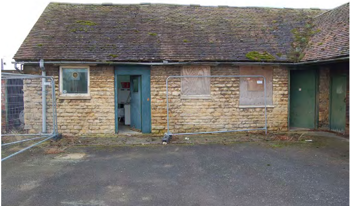
Plate 80: Laundry frontage of Building 4 viewed to south-east
