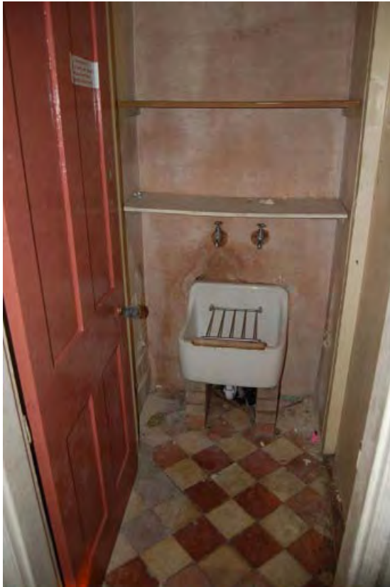
Plate 29: Interior of sluce room G16 In Building 1, viewed to north-east
