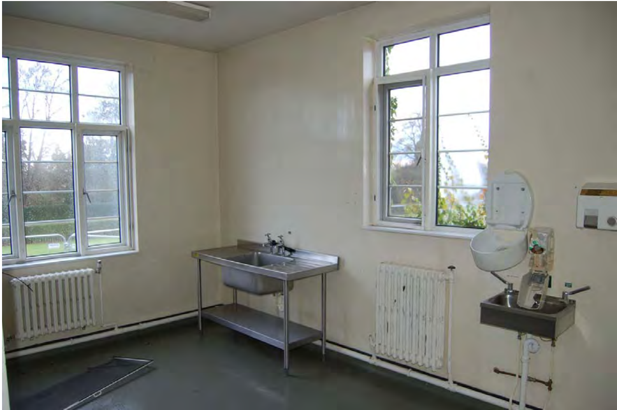
Plate 113: Former kitchen area in kitchen block (Building 9), viewed to north-east
