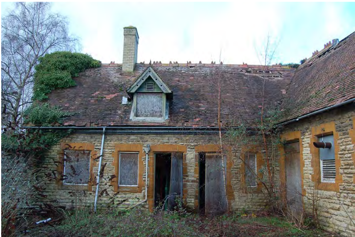
Plate 64: South-west range of stable block (Building 2) viewed to north-west
