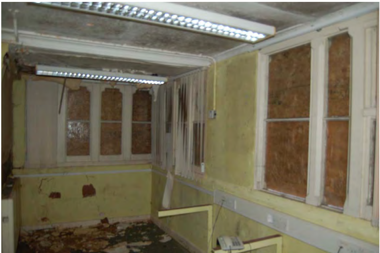
Plate 14: Interior of room G02 in Building 1, viewed to north-west
