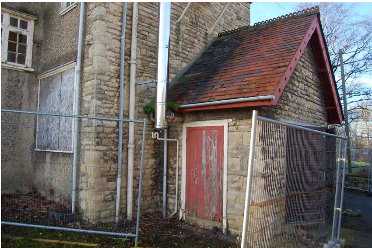
Plate 4: Boiler house on north-east end of Building 1
