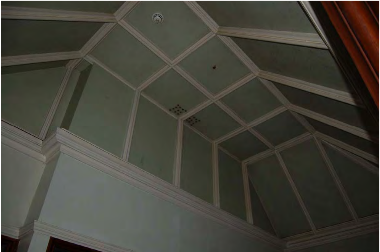
Plate 35: Partitioned stair lobby ceiling in Room F01, Building 1
