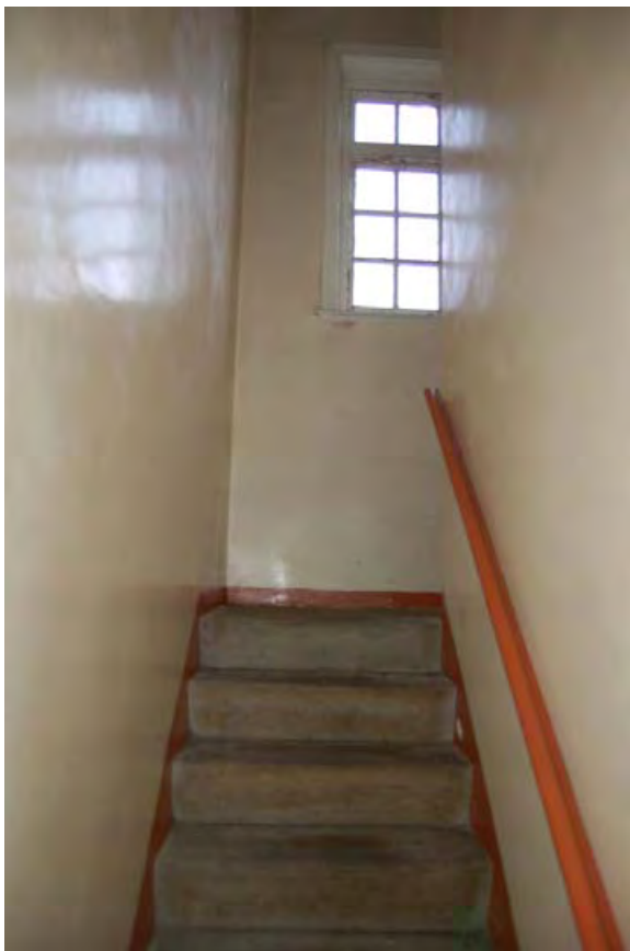
Plate 52: Stair F34 in Building 1, viewed to north-east
