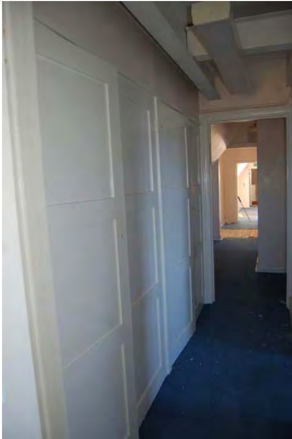
Plate 57: Laundry cupboards in Room A08 in Building 1, viewed to south
