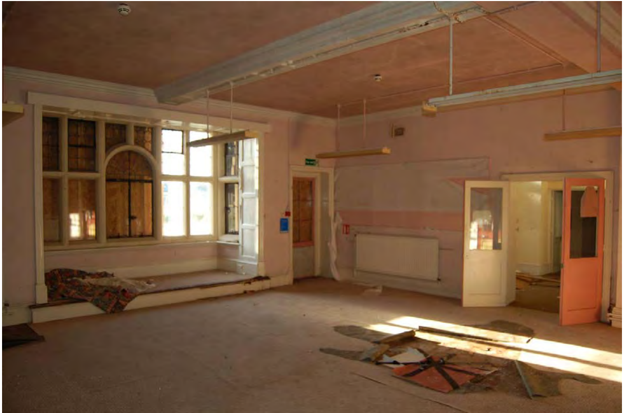
Plate 25: Interior of Room G15 in Building 1, viewed to west
