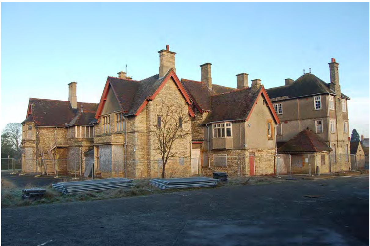
Plate 2: Building 1 viewed to north-west
