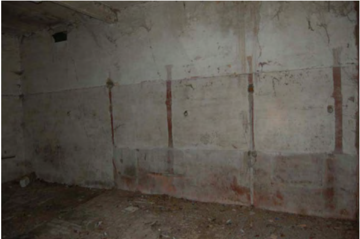
Plate 69: Former stable G06 showing removed stalls, viewed to north
