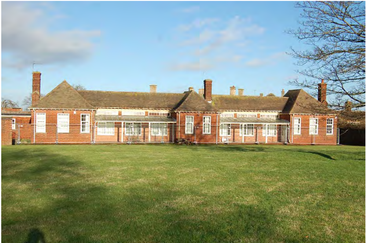
Plate 91: Well-preserved south side of ward block (Building 5), showing verandas
