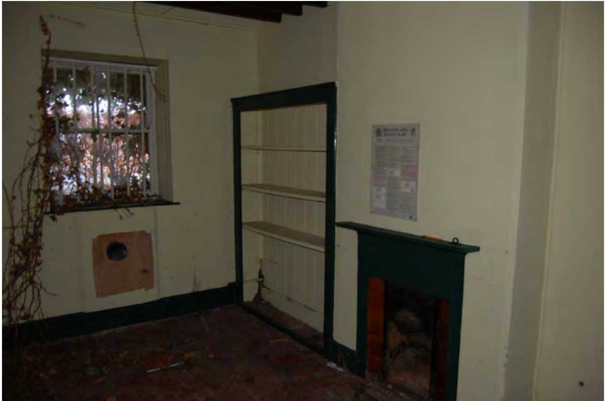
Plate 67: Room G04 in stable block (Building 2), viewed to north
