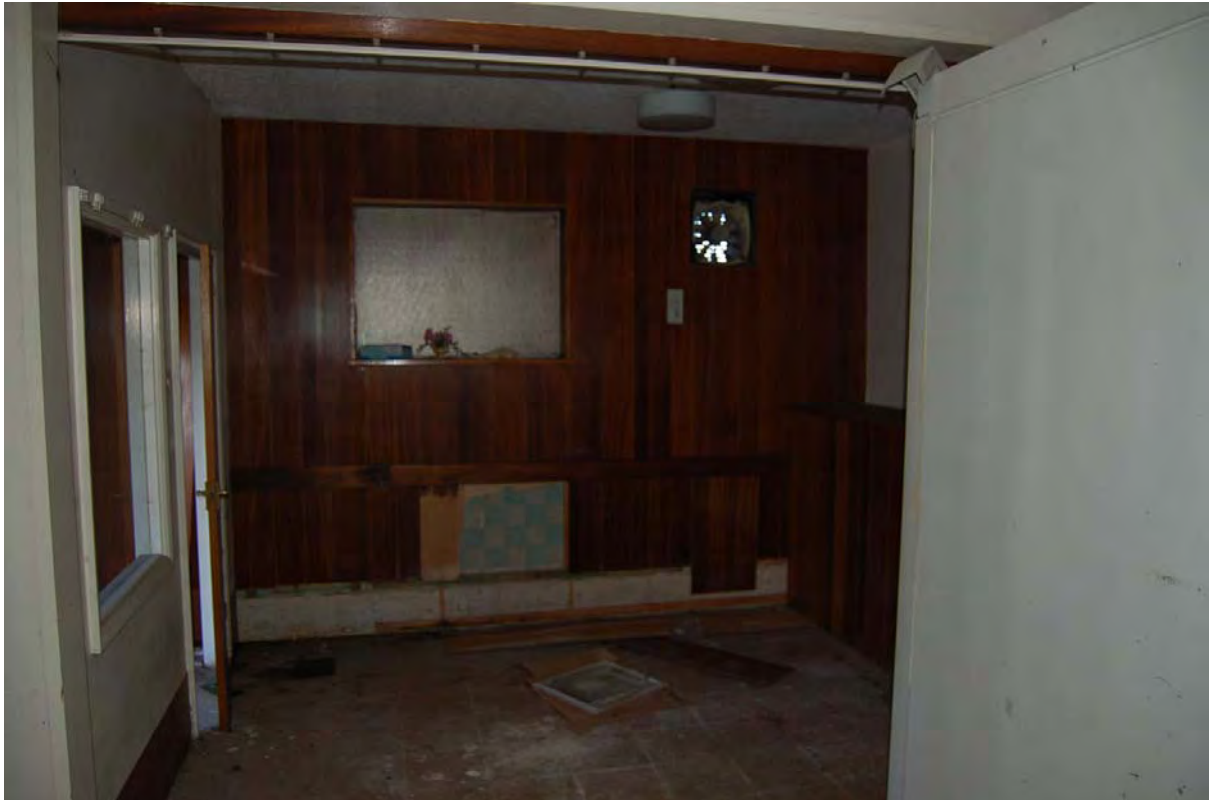
Plate 77: Room G02 inside mortuary (Building 3), viewed to north-east
