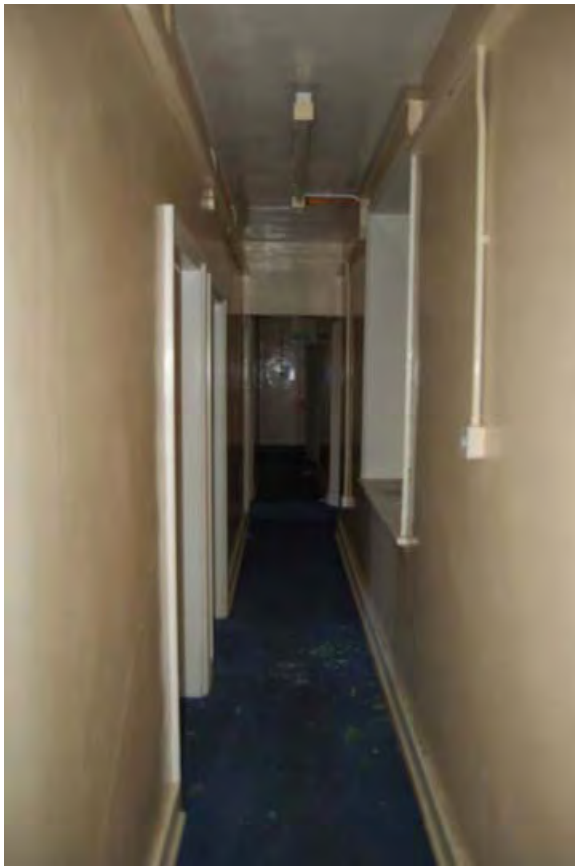
Plate 48: Corridor F25 in Building 1, viewed to north-east
