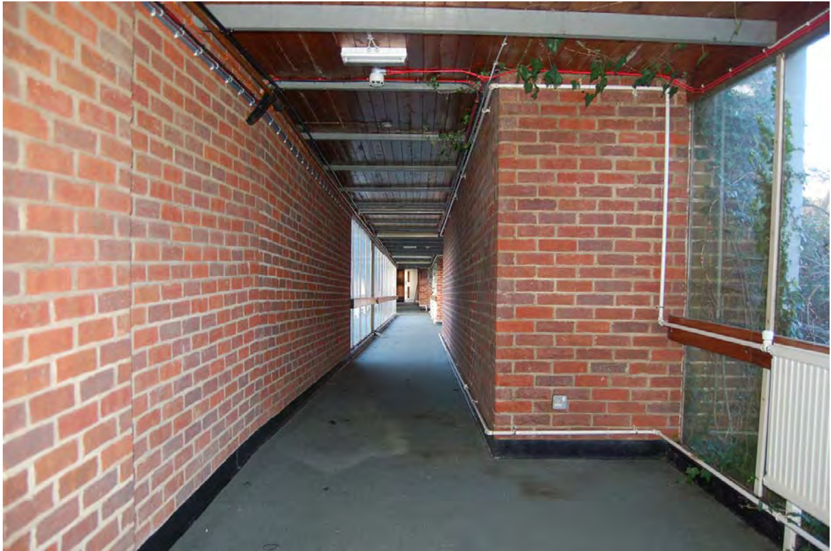
Plate 115: Interior of linking corridor (Building 10) viewed to north
