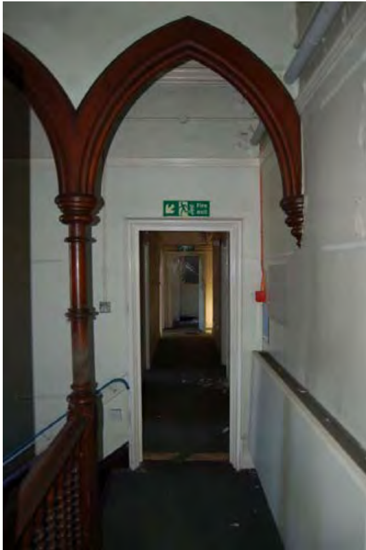
Plate 39: Gothic arch on stair landing F01, leading through to corridor F14 in Building 1, viewed to south-east
