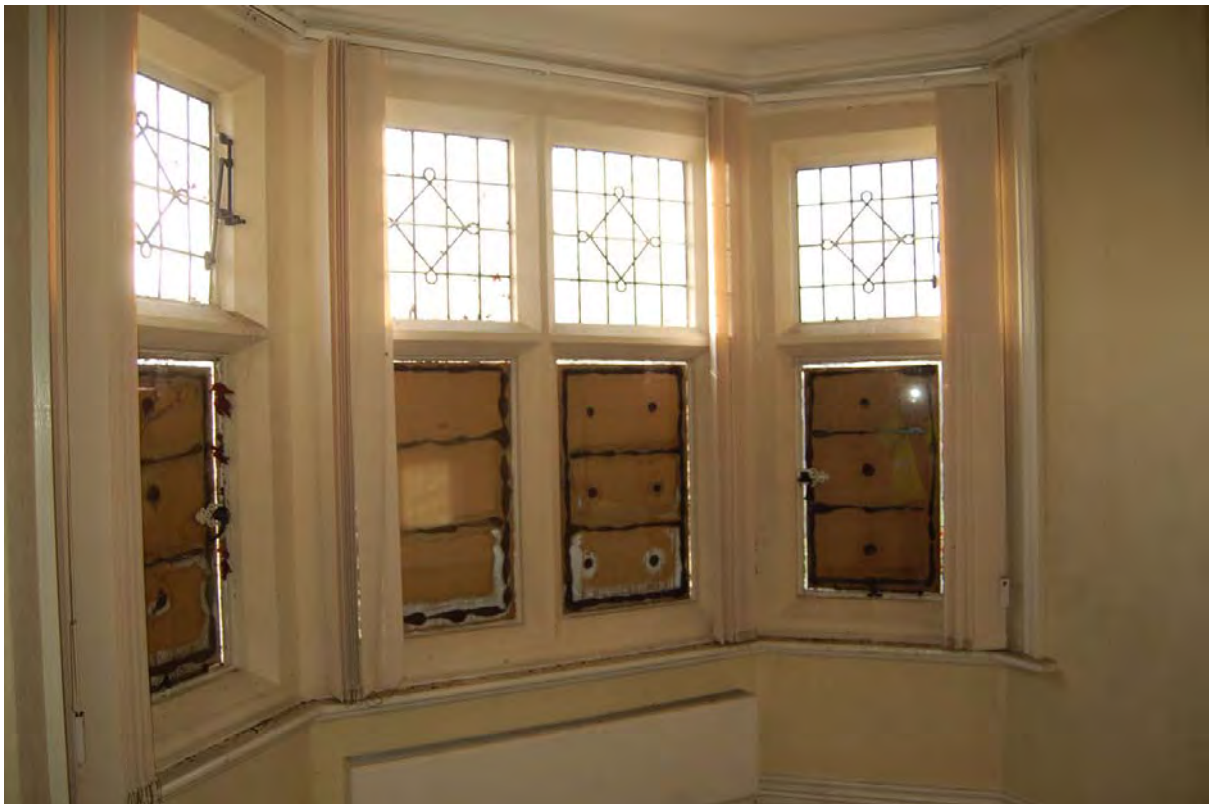
Plate 38: Leaded window in Room F9 in Building 1, viewed to west
