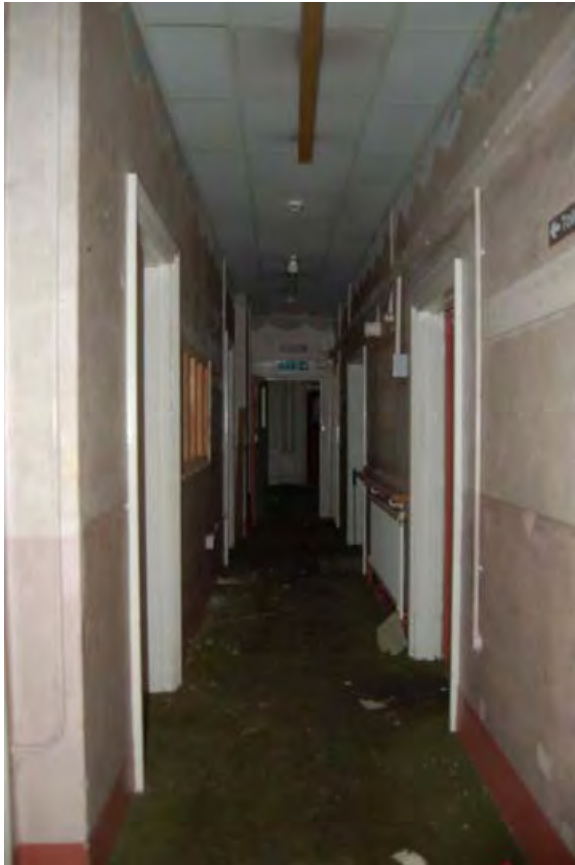
Plate 21: Corridor G05 in Building 1, viewed to north-east
