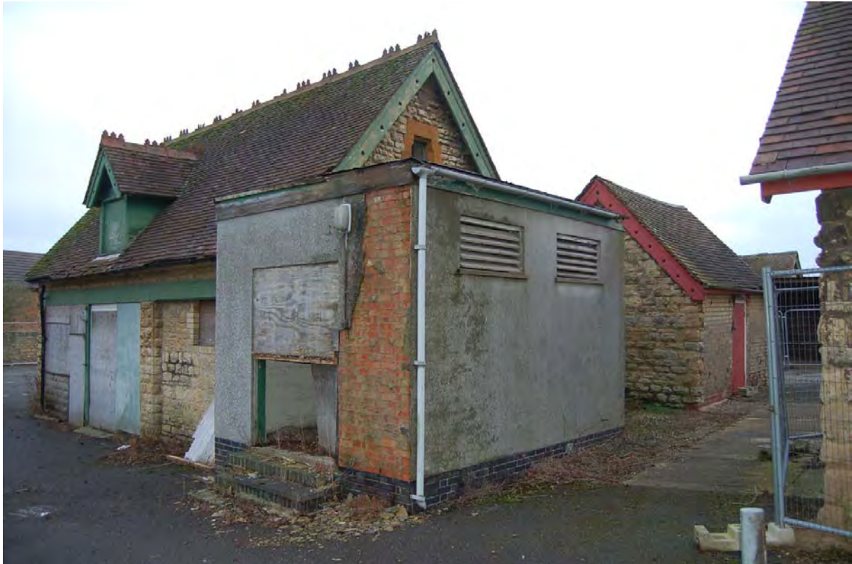
Plate 73: Mortuary (Building 3) viewed to east, with modern boiler house and clinical waste buildings
