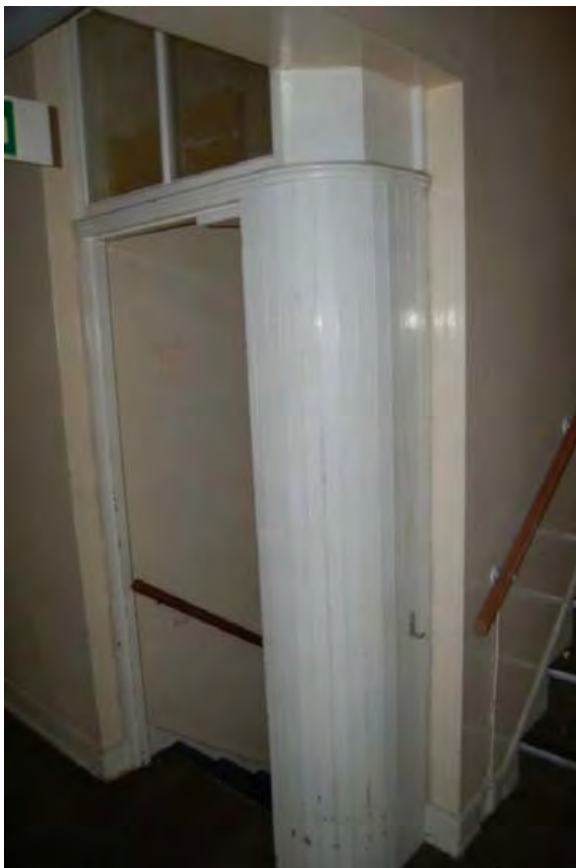
Plate 46: Entrance to service stair F24 in Building 1, viewed to south
