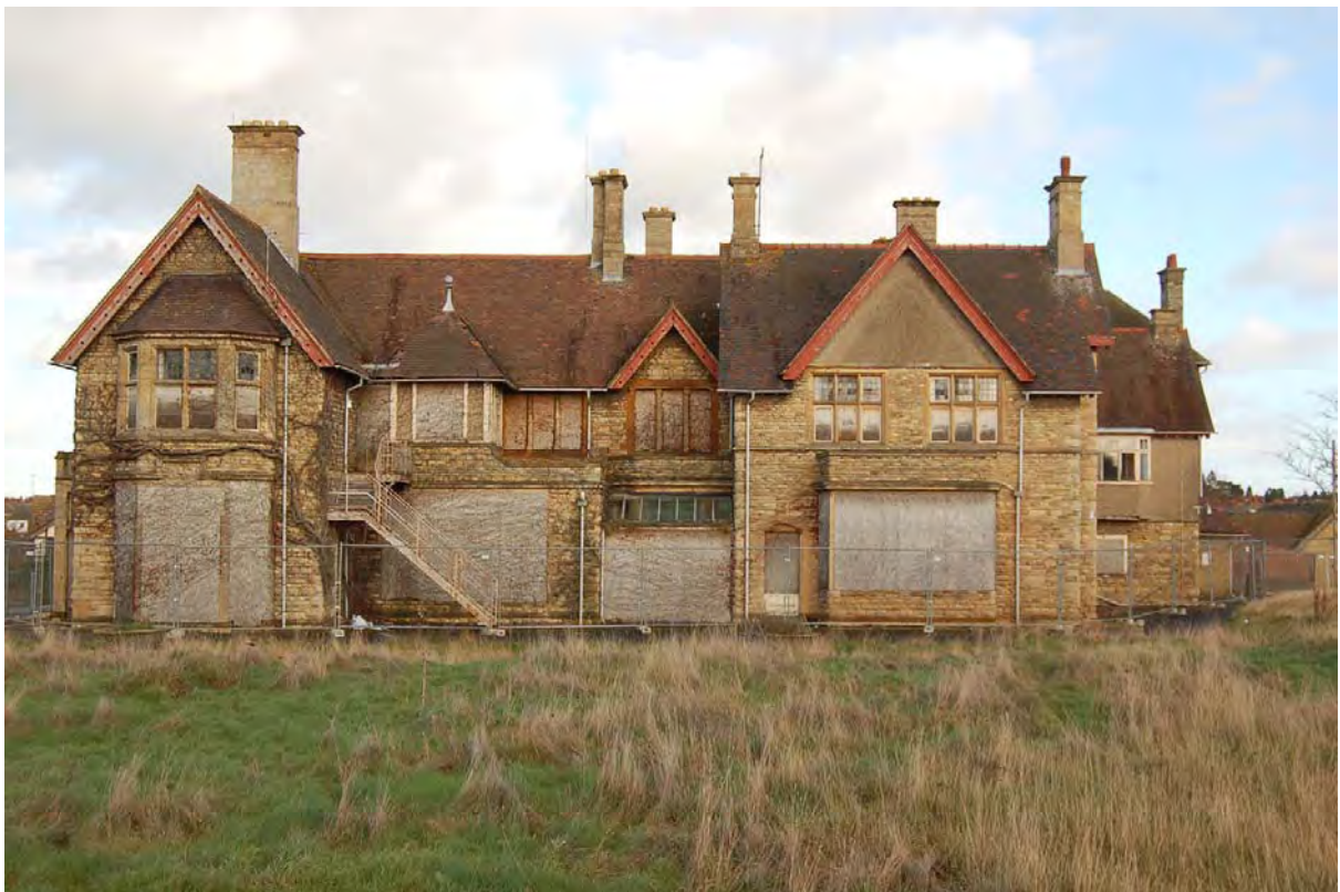
Plate 10: South-west elevation of 'house' range of Building 1
