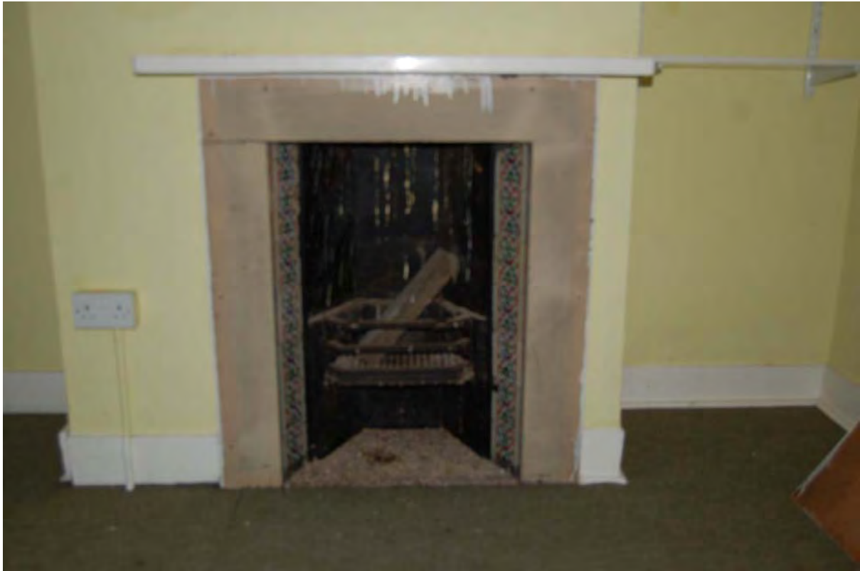
Plate 49: Fireplace in Room F29 in Building 1, viewed to north-east
