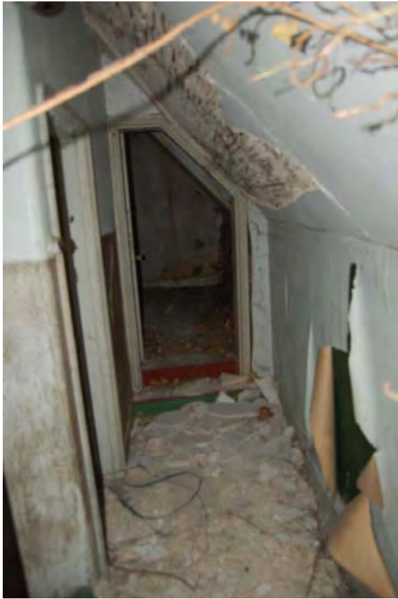
Plate 71: First floor corridor F01 in stable block (Building 2), viewed to south-west
