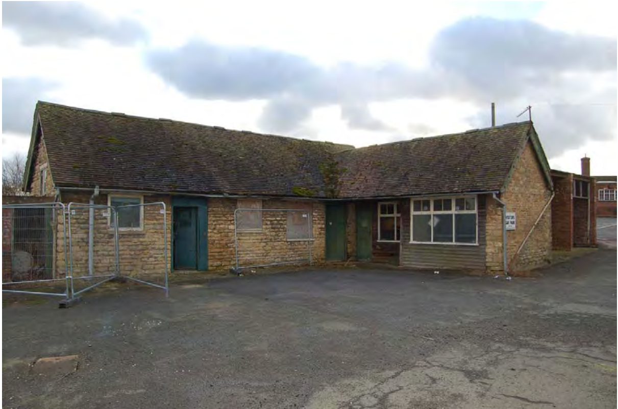
Plate 79: Laundry/workshop (Building 4) viewed to south
