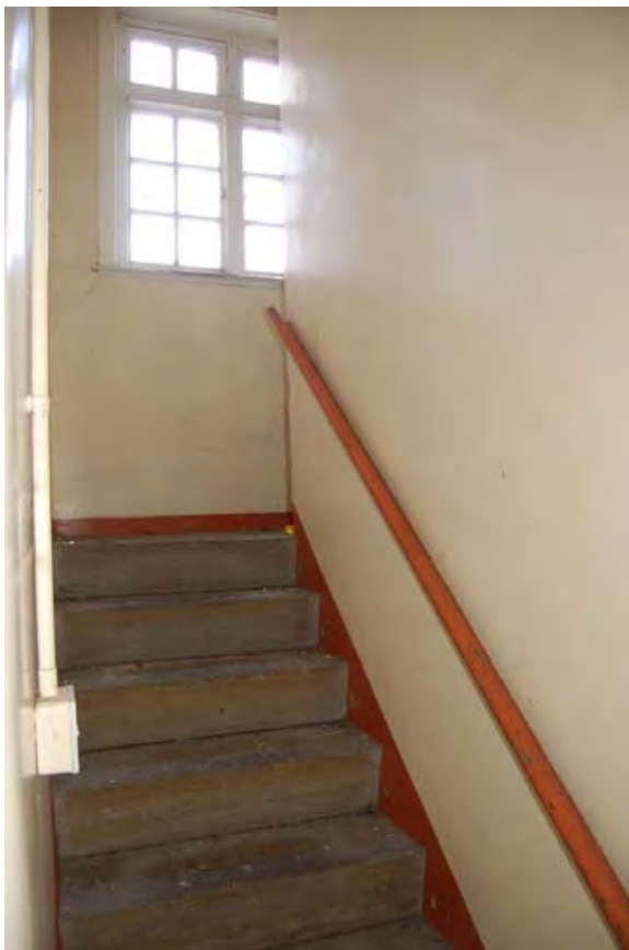
Plate 34: Stair G32 in later extension to Building 1, viewed to north-east
