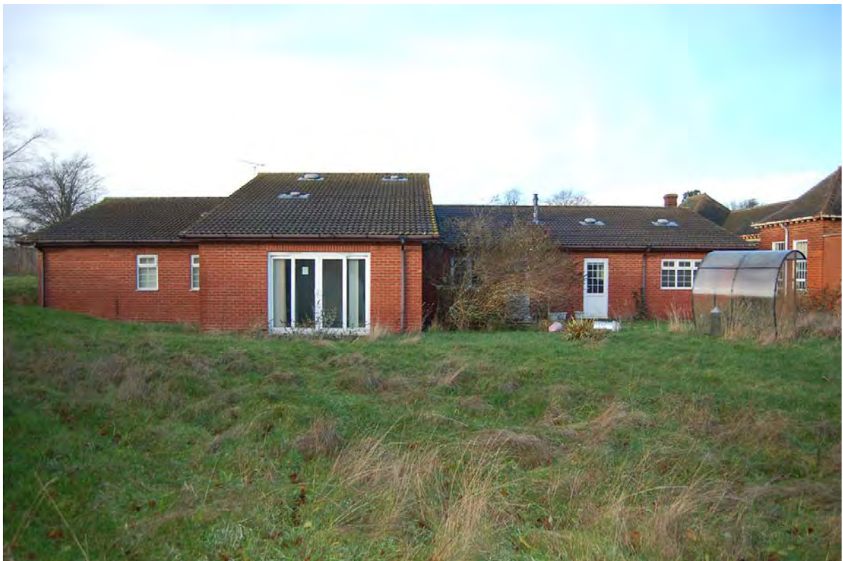
Plate 116: Hargrave House Annexe (Building 11), viewed to west
