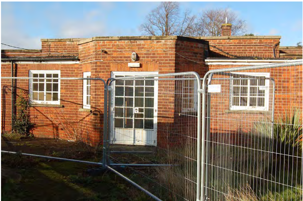
Plate 110: Entrance into kitchen (Building 9) and linking corridor viewed to north-west
