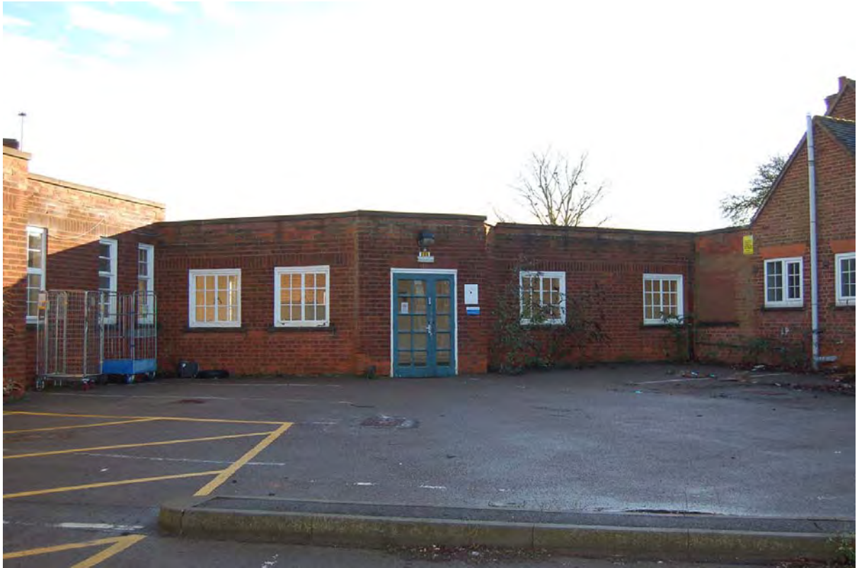
Plate 109: Kitchen linking corridor (Building 9) viewed to east
