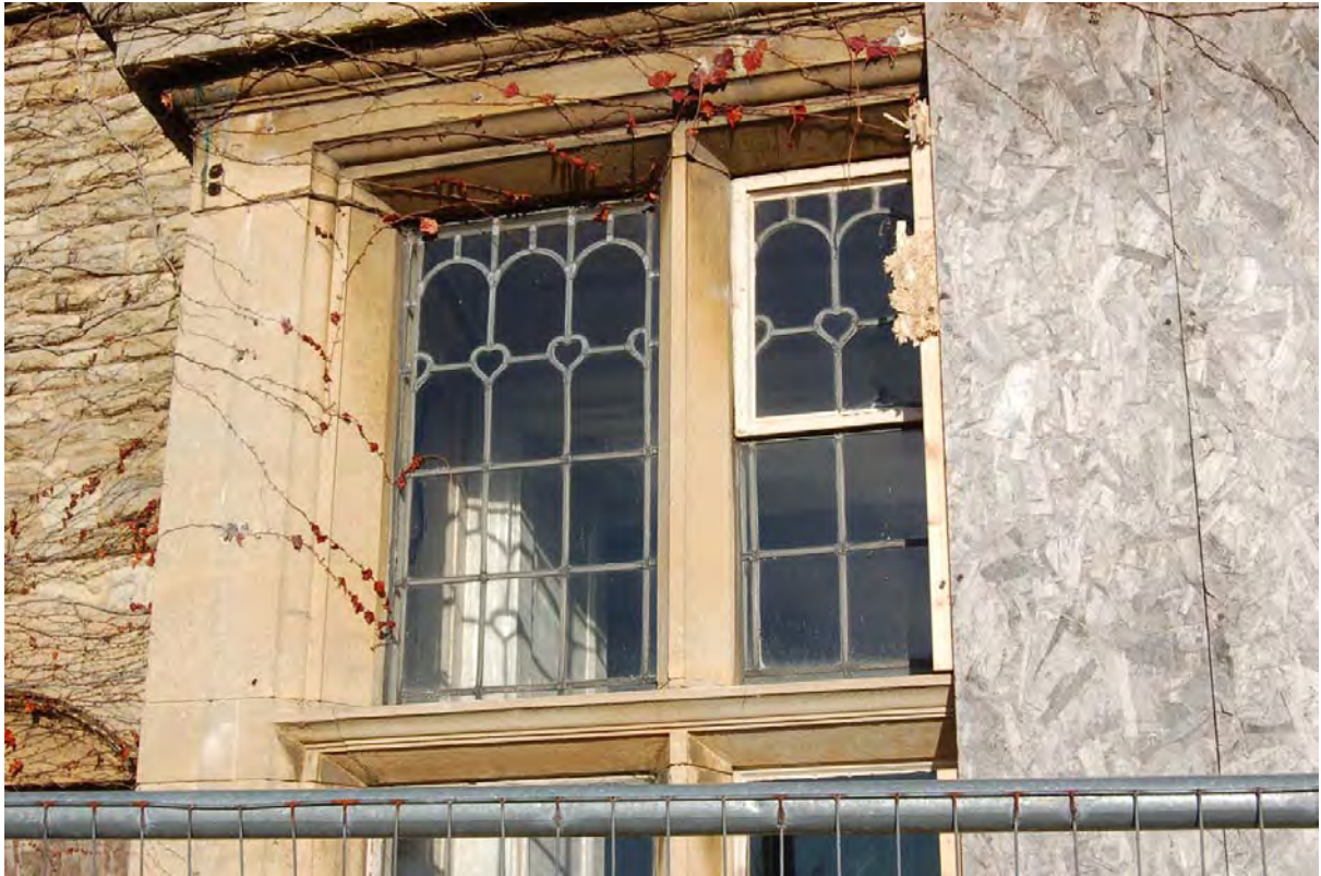
Plate 13: Window detail on Room G15 of Building 1, viewed externally
