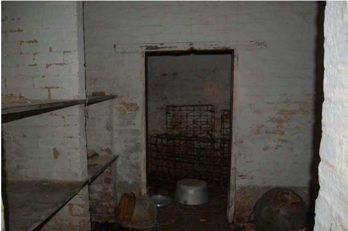
Plate 61: View through dairy B04 into wine cellar B05 in Building 1, viewed to north-west
