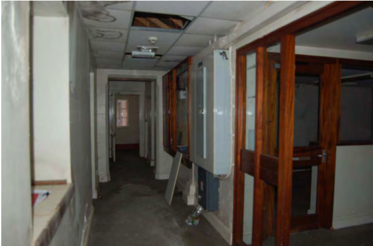
Plate 31: Corridor G22 beside modern reception area in Building 1, viewed to north-east
