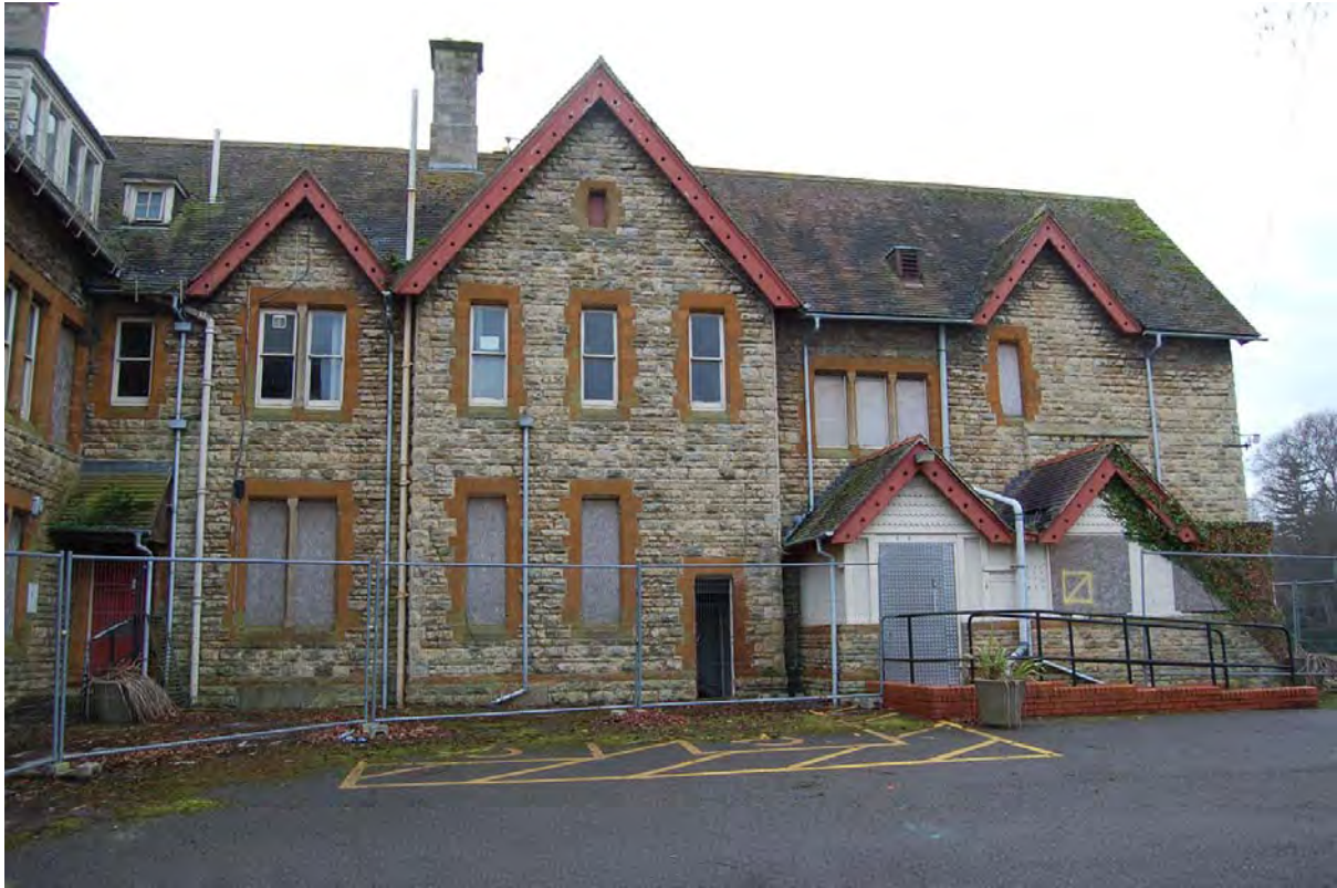
Plate 5: North-east elevation of 'house' range of Building 1
