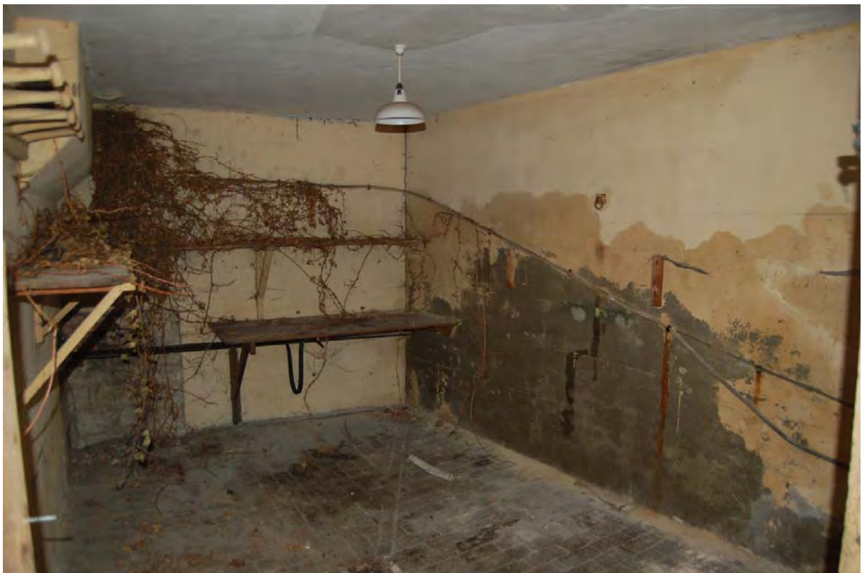
Plate 68: Washroom G05 in stable block (Building 2), viewed to north-west
