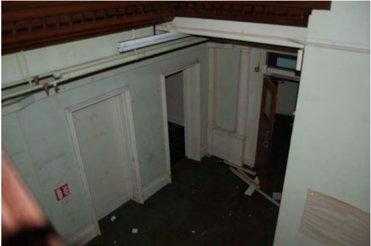
Plate 15: View from main stair of Building 1 to lobby G03
