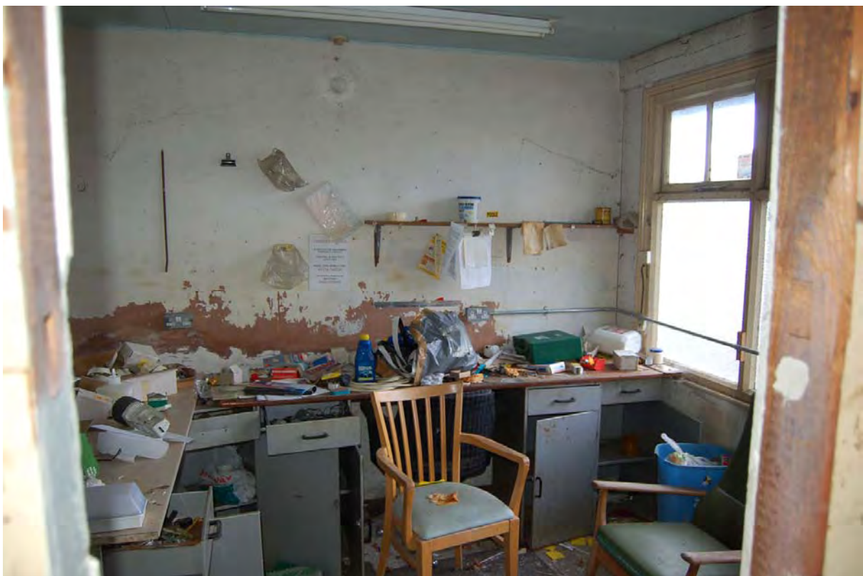
Plate 86: Staff Room G06 in workshop (Building 4), viewed to north-west
