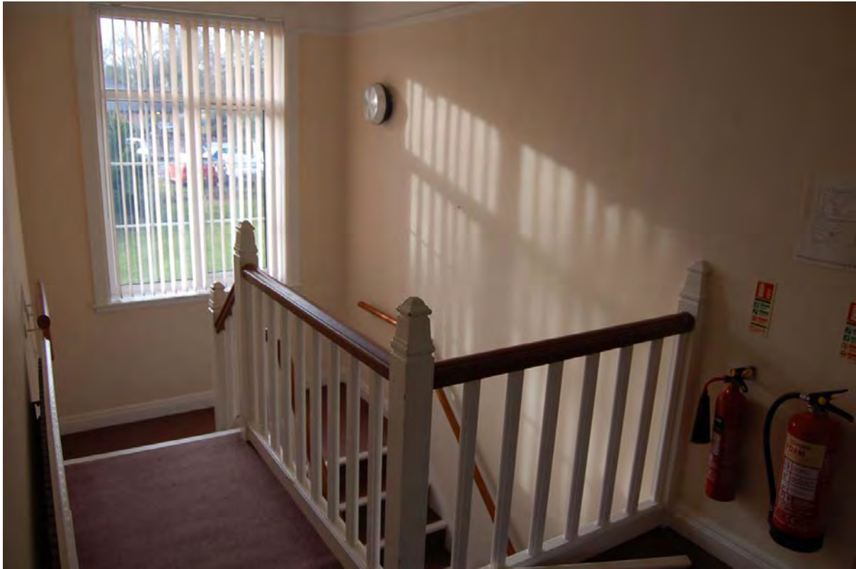
Plate 121: Grange (Building 12) stair, viewed from first floor landing towards south-west
