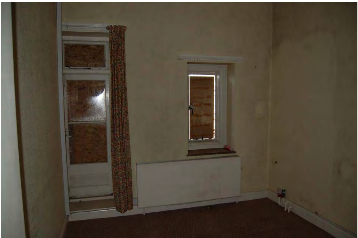
Plate 36: Divided French window in Room F07 in Building 1, viewed to north-west
