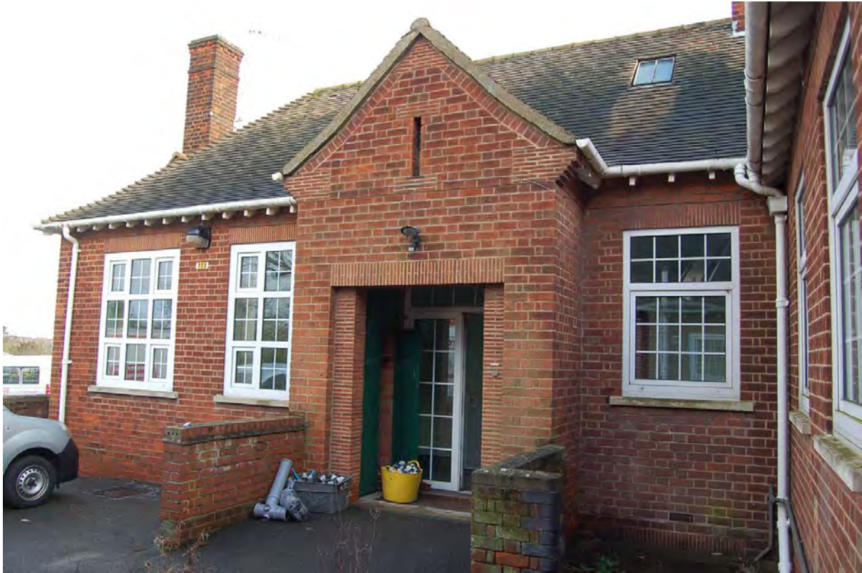
Plate 103: Porch on west side of central projecting block of ward block (Building 8)
