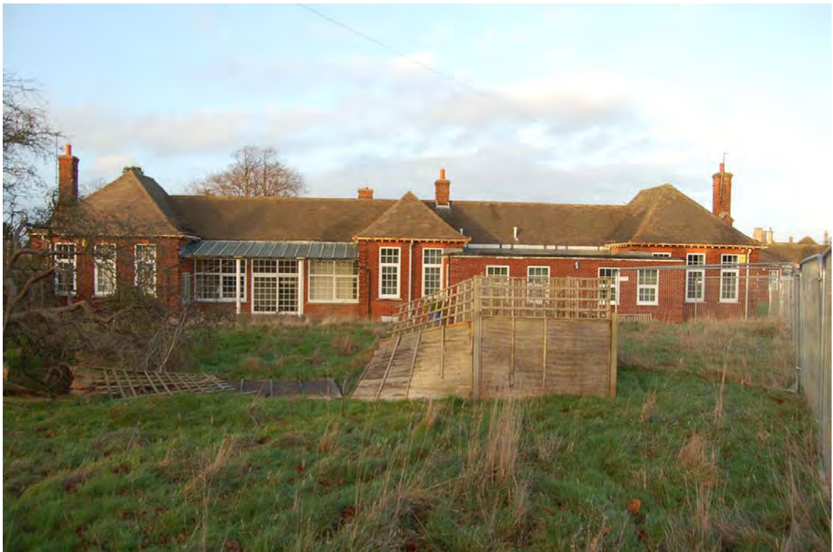
Plate 98: South elevation of ward block (Building 7)
