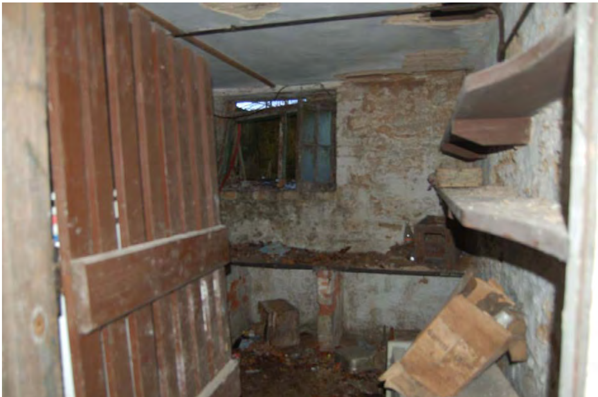
Plate 60: Beer cellar B03 below Building 1, viewed to north-east
