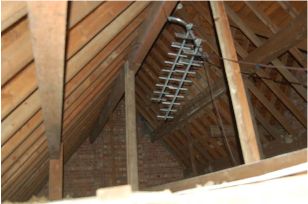
Plate 43: Roof space over 1907 south block of Building 1, viewed to south-east
