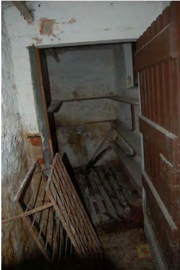
Plate 59: Larder B02 in basement of Building 1, viewed to north-west
