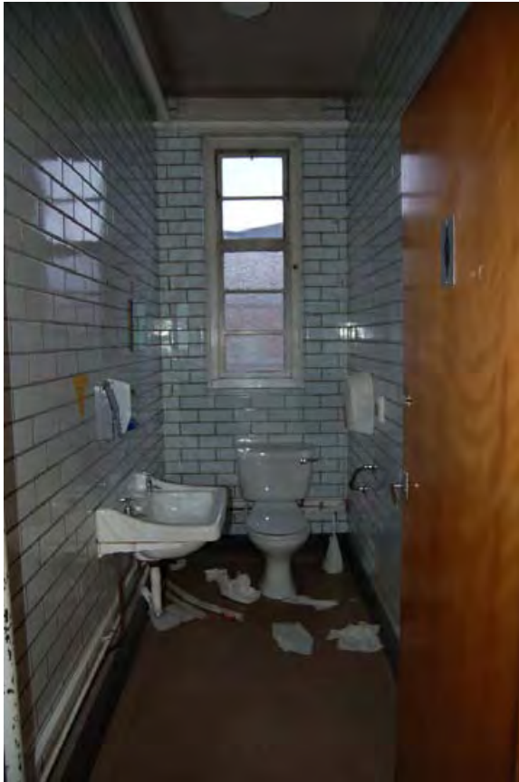
Plate 111: White 'brick' wall tiling in kitchen block toilet, viewed to south-east
