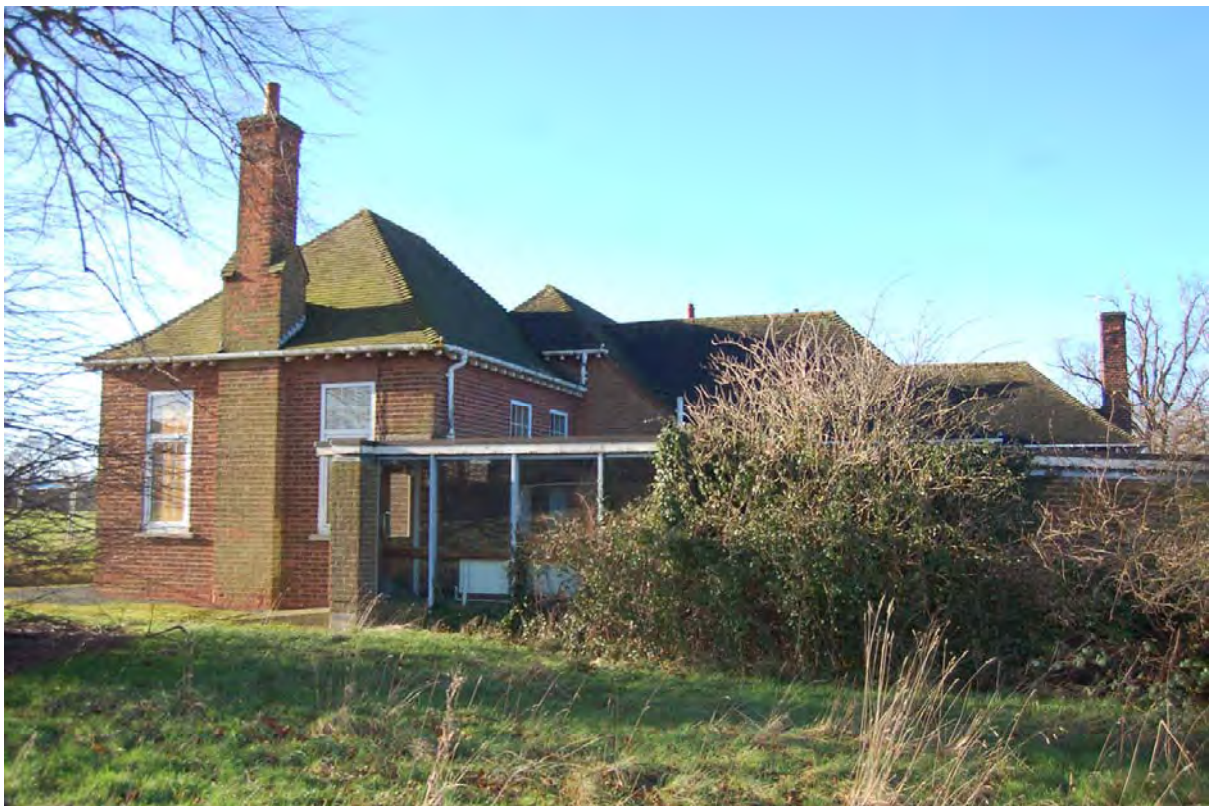
Plate 114: Linking corridor (Building 10) viewed to west, with ward block (Building 8)
