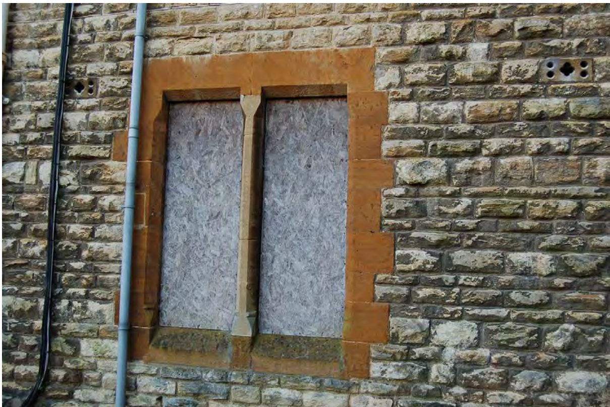
Plate 8: Building 1 window detail
