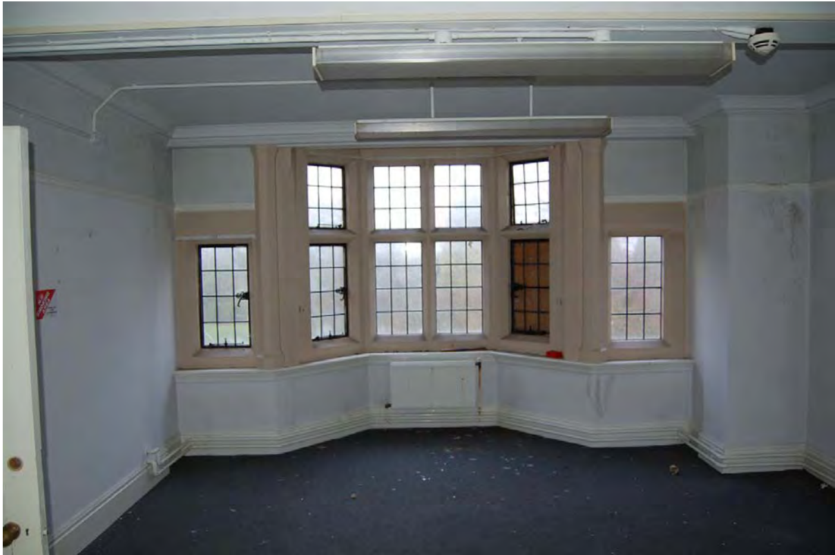
Plate 51: Room F33 in Building 1, viewed to north-west
