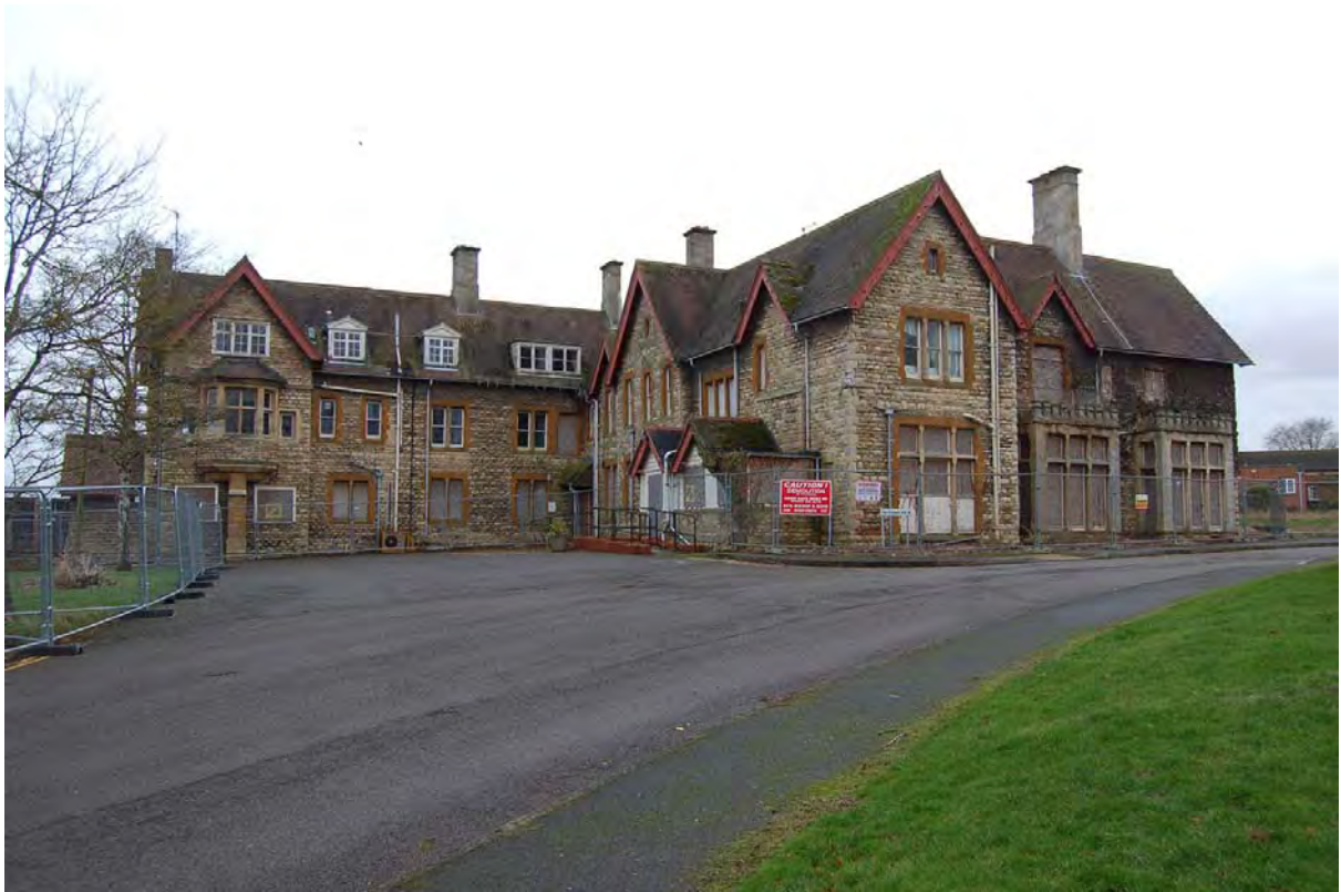
Plate 1: Building 1 viewed to south
