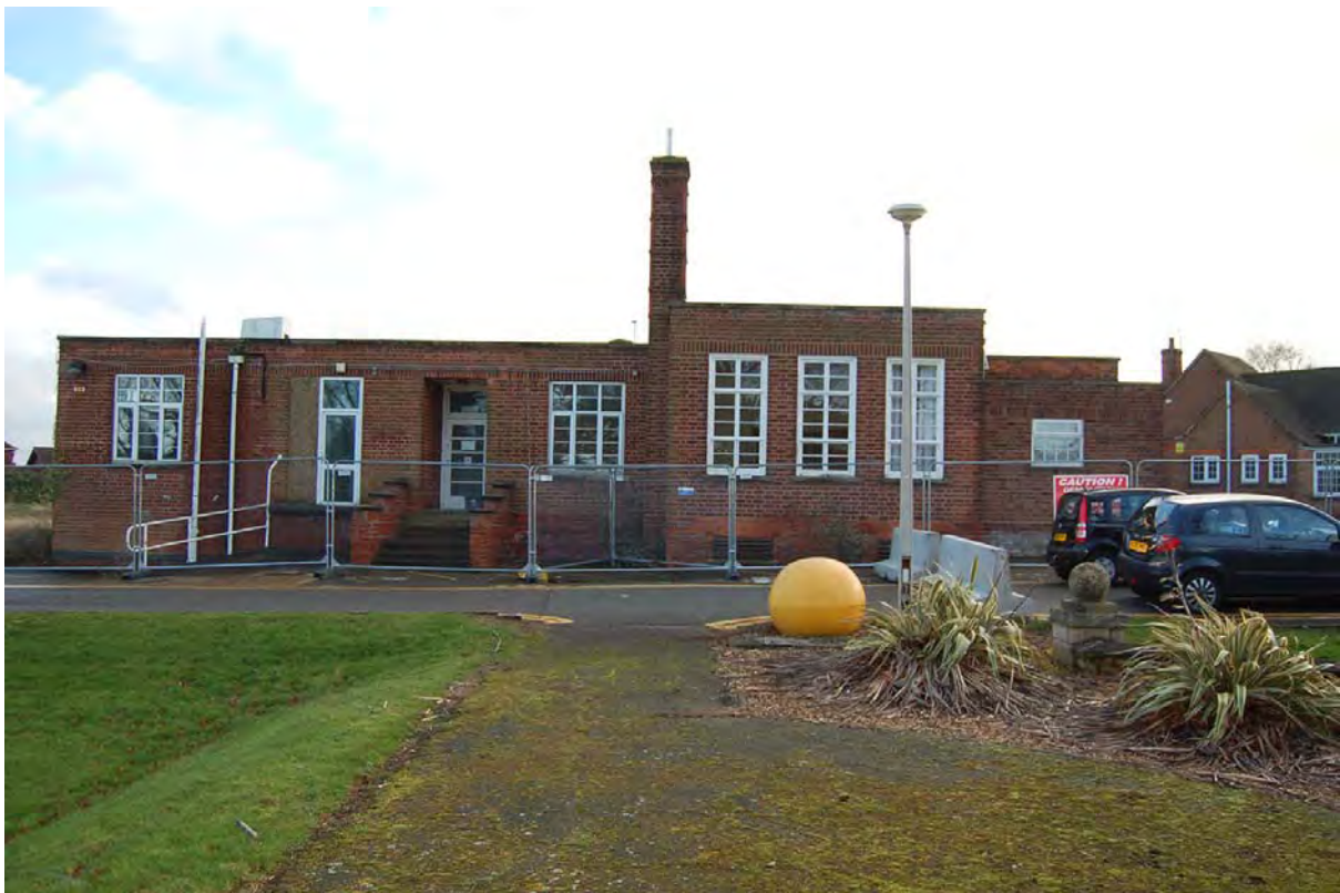
Plate 106: Main façade of kitchen block (Building 9), viewed to south-east
