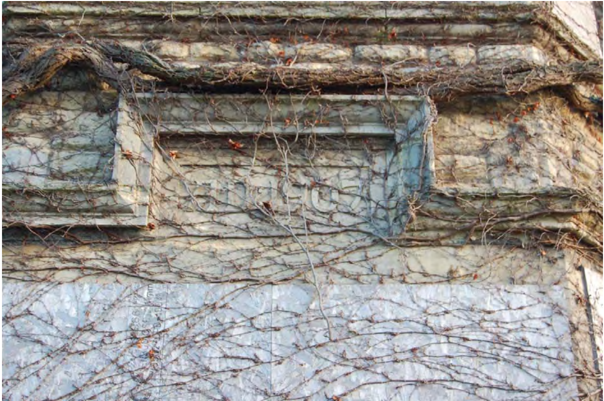
Plate 11 1907 Date plaque on south-west elevation of Building 1
