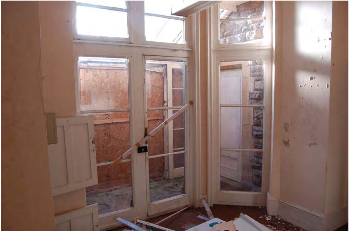
Plate 23: Room G13 in Building 1, viewed to south-west east into 1907 lobby
