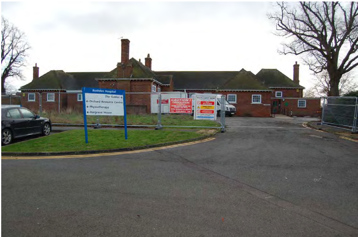
Plate 100: North elevation of ward block (Building 8)
