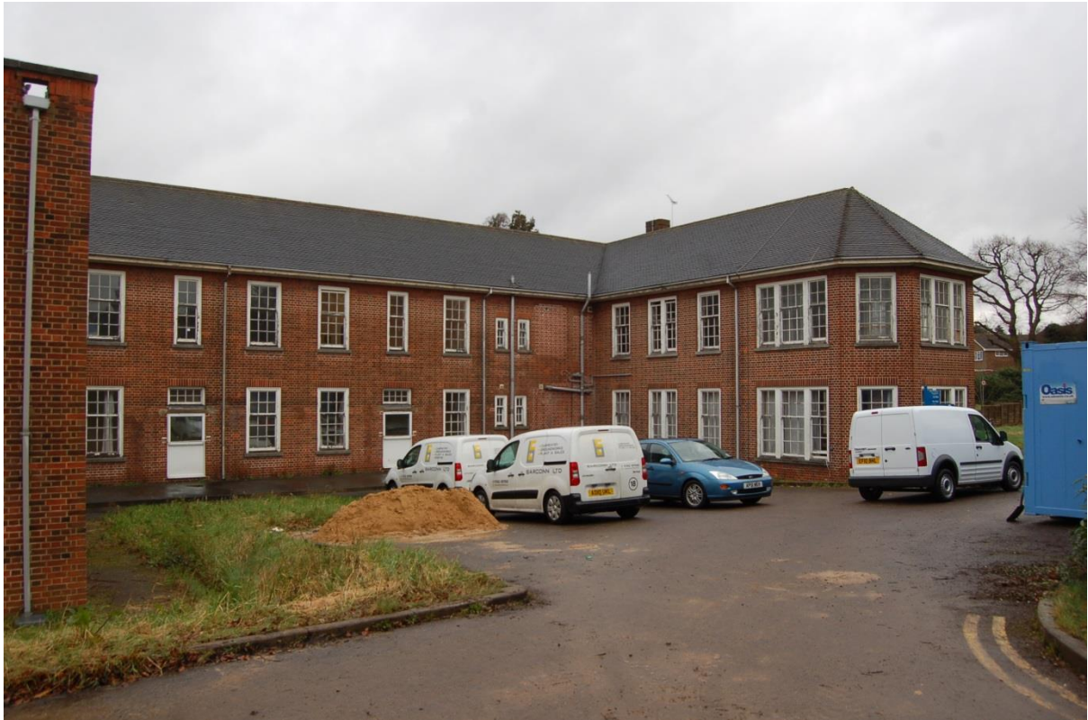
Plate 25: Building 2, dayroom block viewed to northeast
