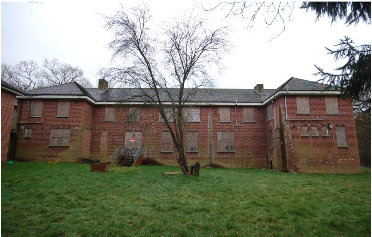
Plate 88: Building 4, south elevation
