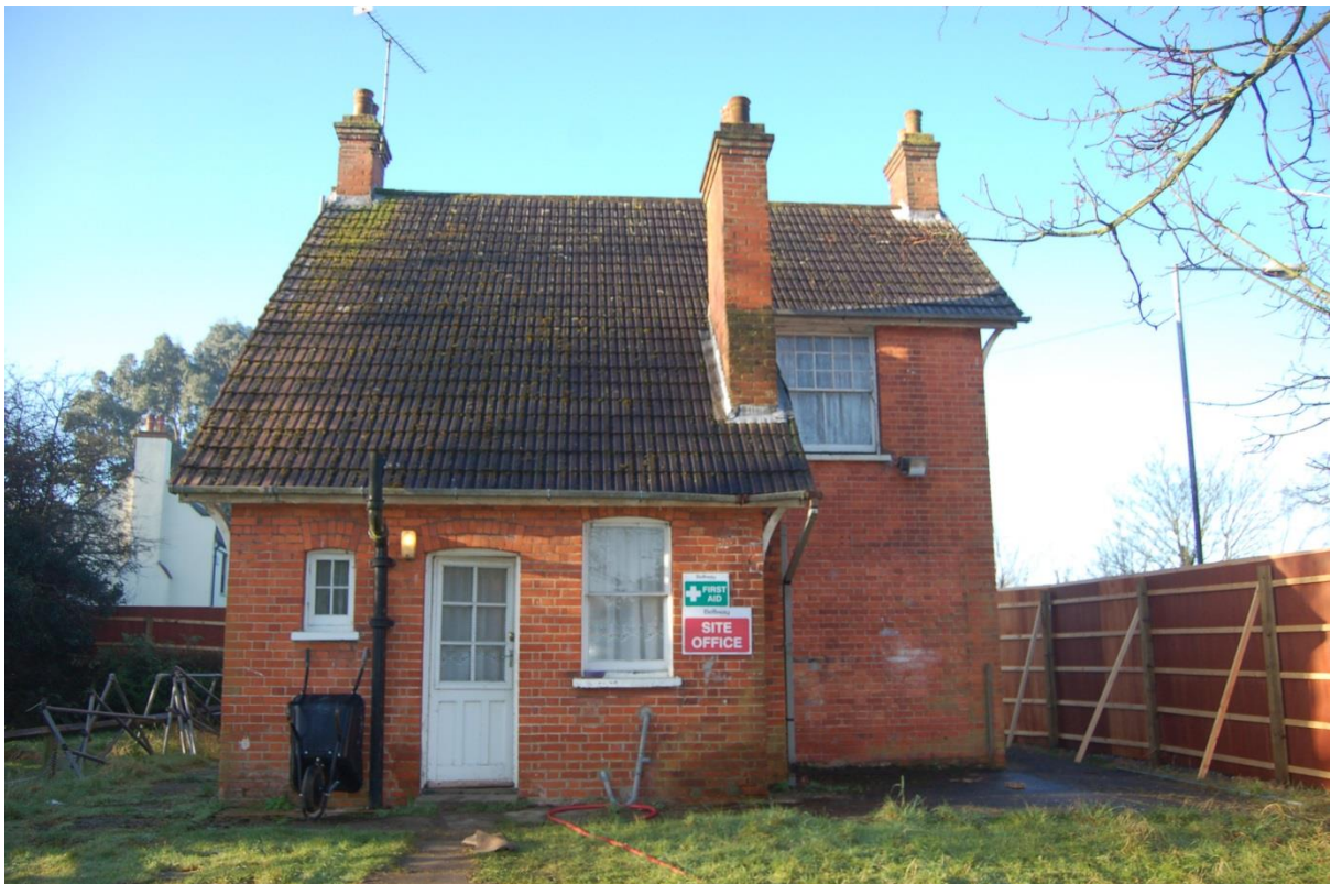
Plate 107: Building 6, northeast elevation
