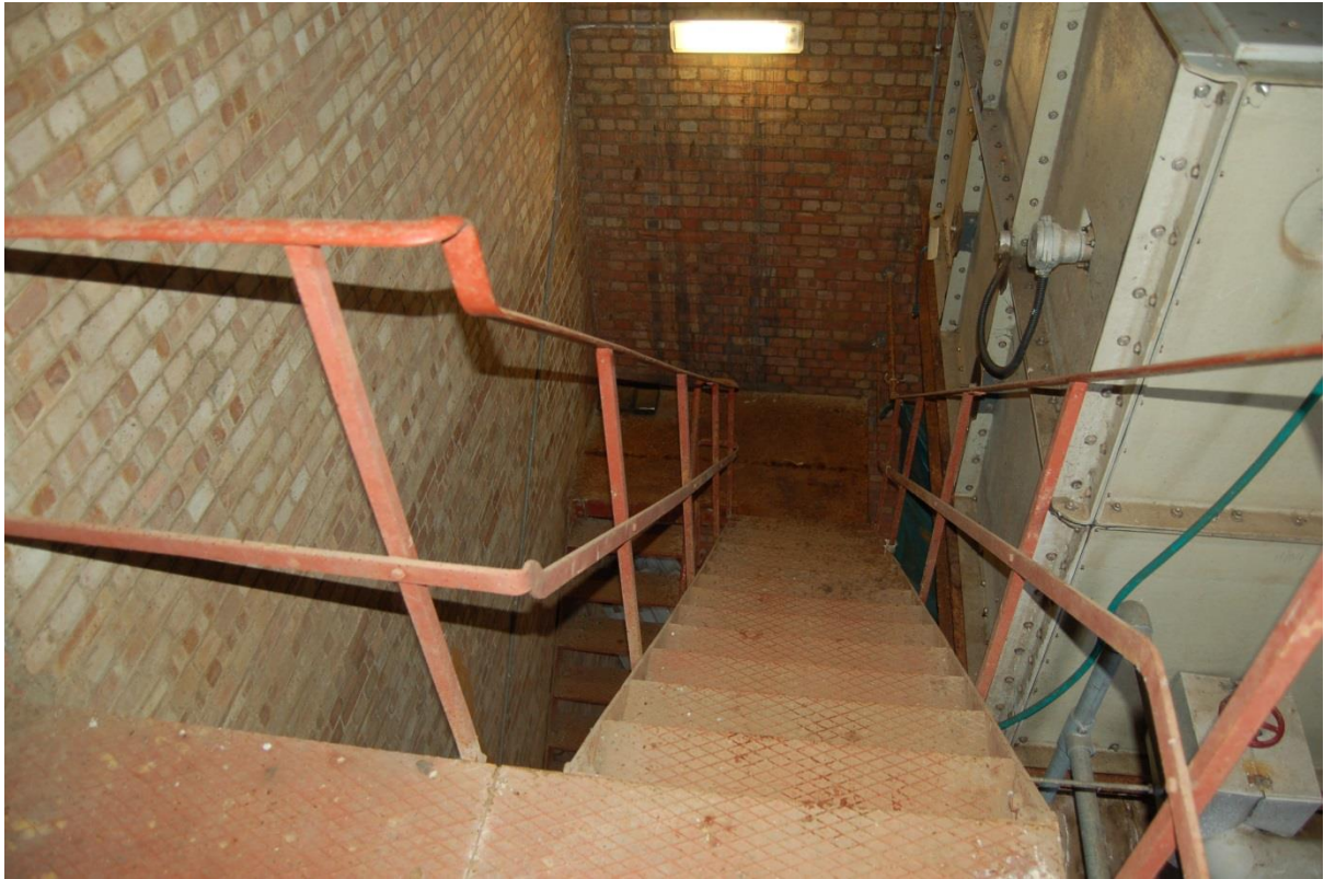
Plate 102: Stair, second floor
