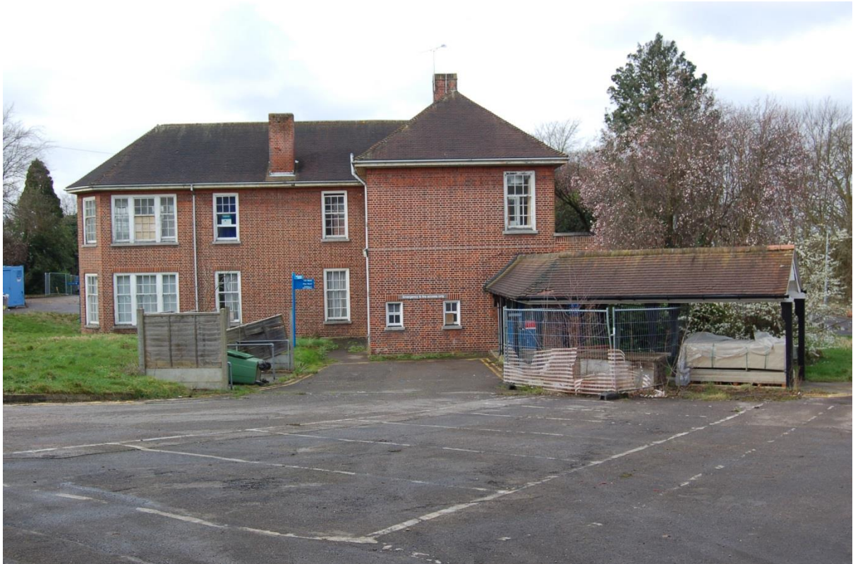
Plate 27: Building 2, east end, with covered passage remains
