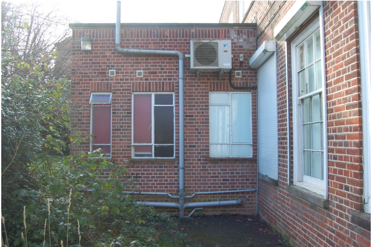
Plate 3: Building 1, southwest wing, northeast elevation
