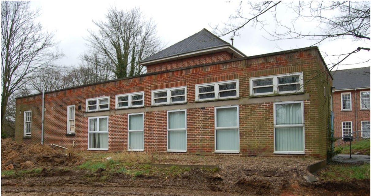
Plate 35: Building 2, east wing viewed to northeast
