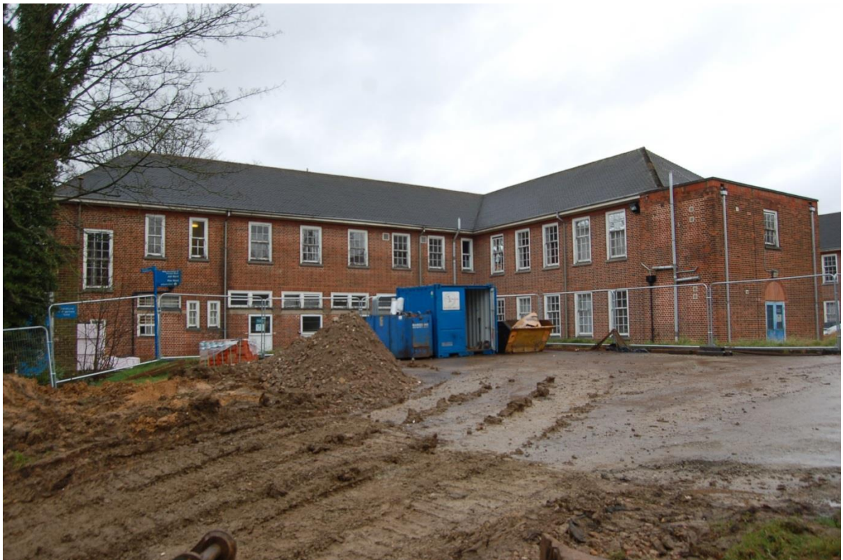
Plate 22: Building 2, western end viewed to northeast
