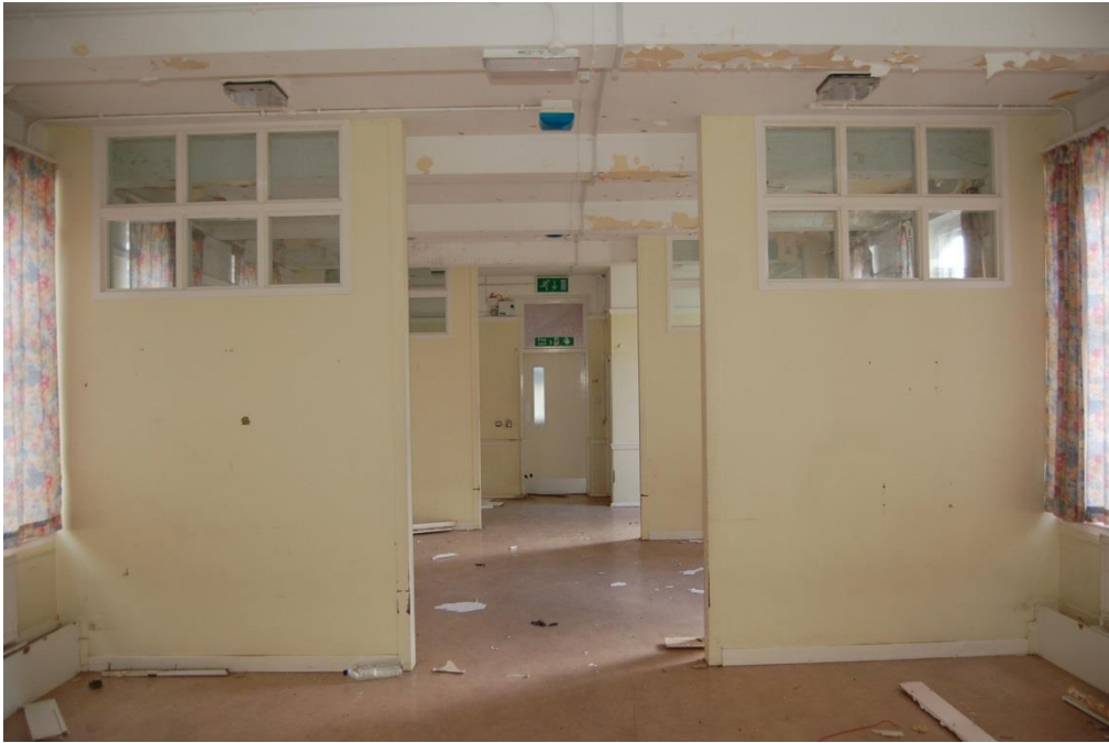
Plate 49: Room 35, viewed to north
