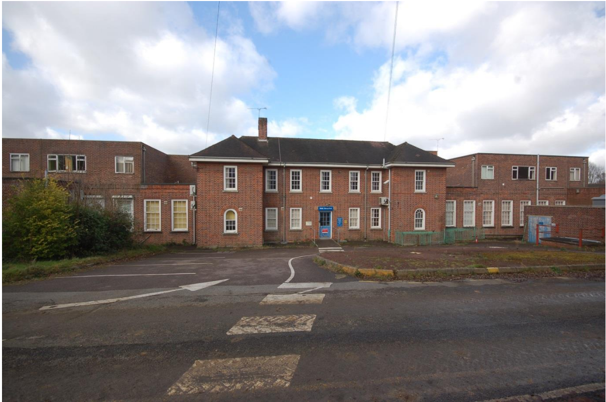
Plate 1: Building 1, southeast elevation
