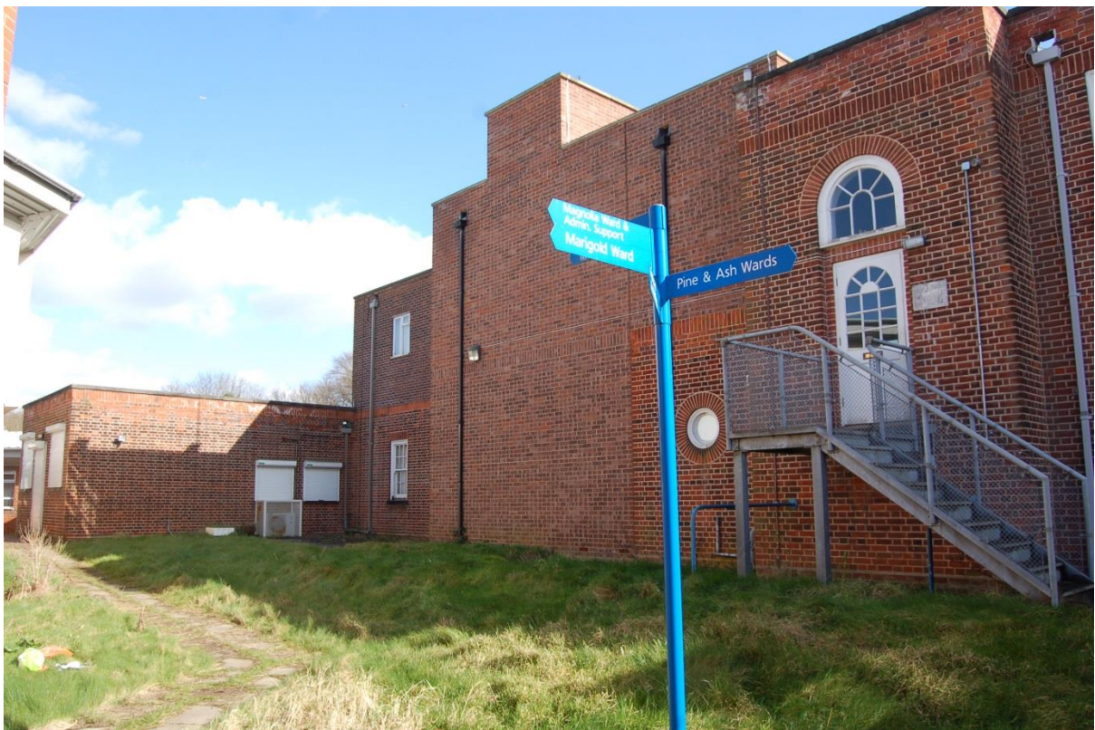
Plate 6: Building 1, northeast end, viewed to east
