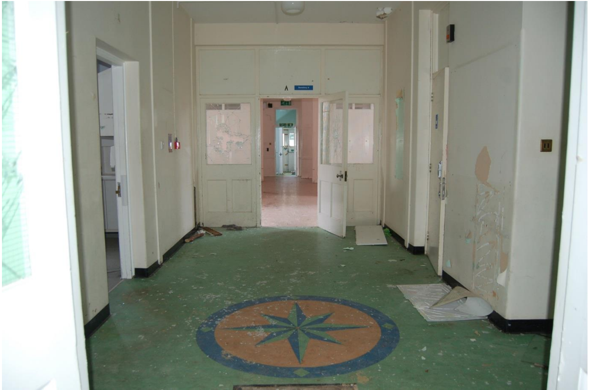
Plate 77: Lobby 18, viewed to southwest
