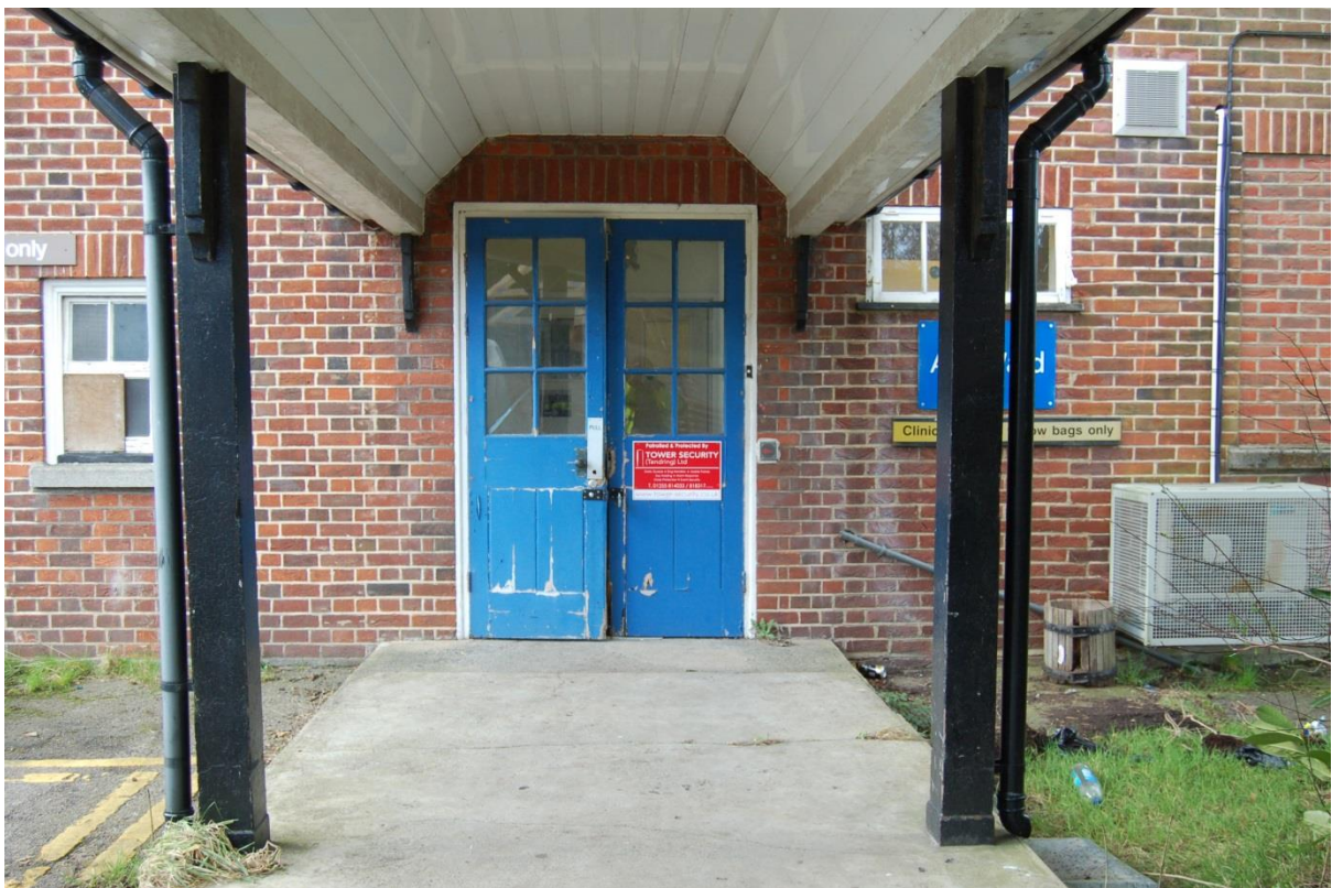
Plate 28: Building 2, east entrance
