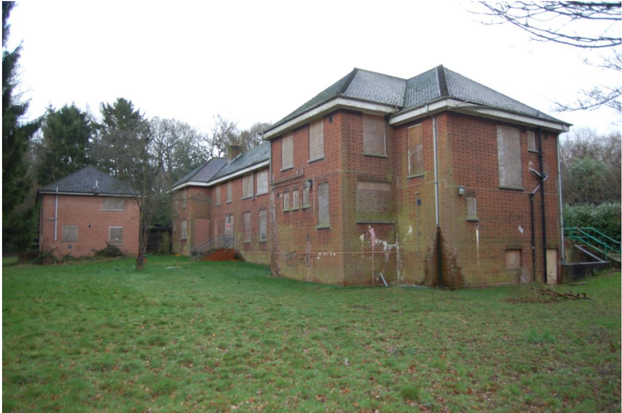
Plate 89: Building 4, viewed to southeast
