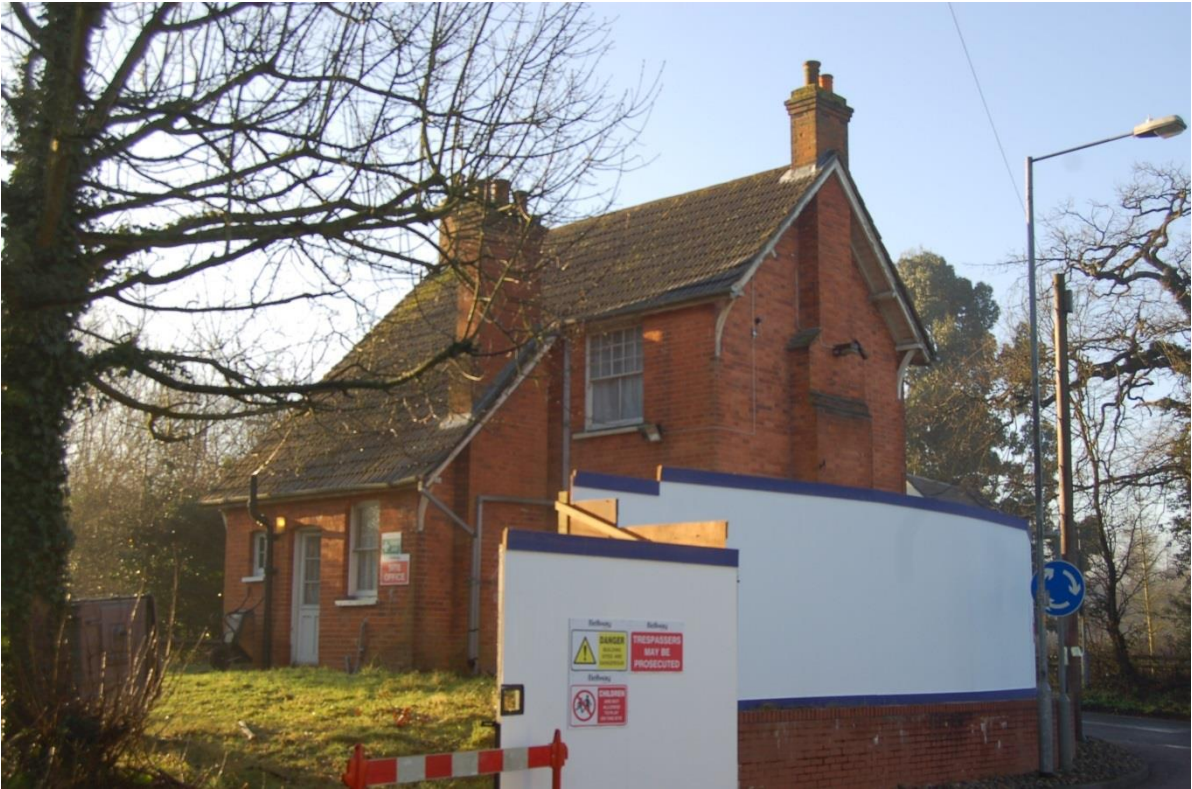
Plate 108: Building 6, viewed to south
