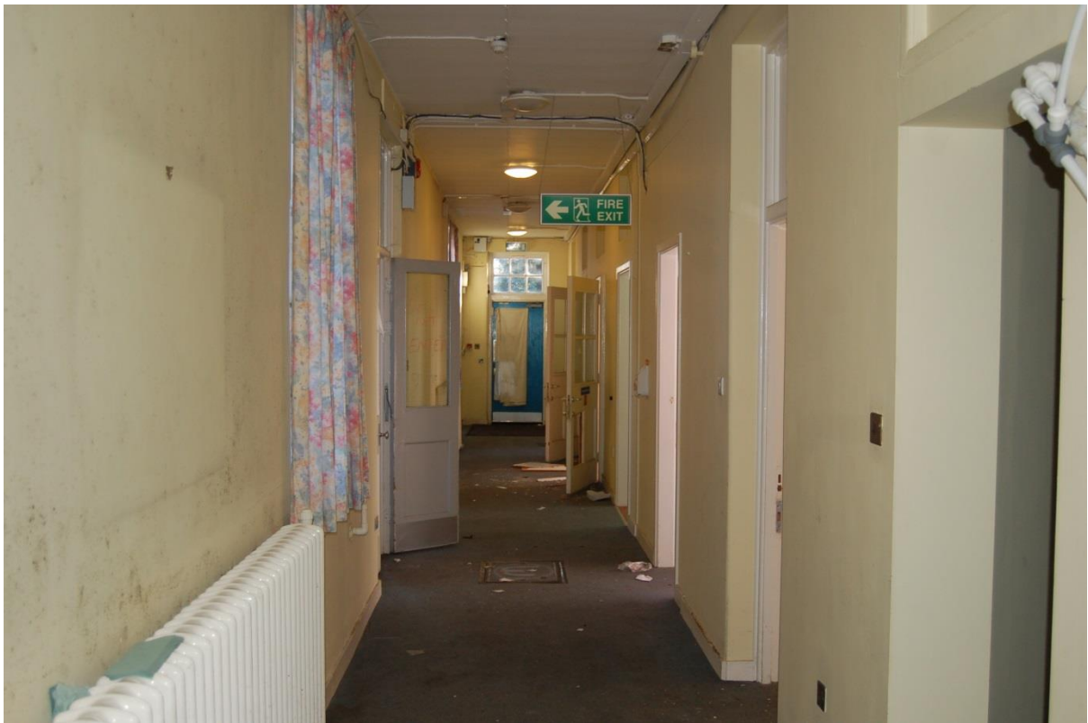
Plate 52: Corridor 55, viewed to south
