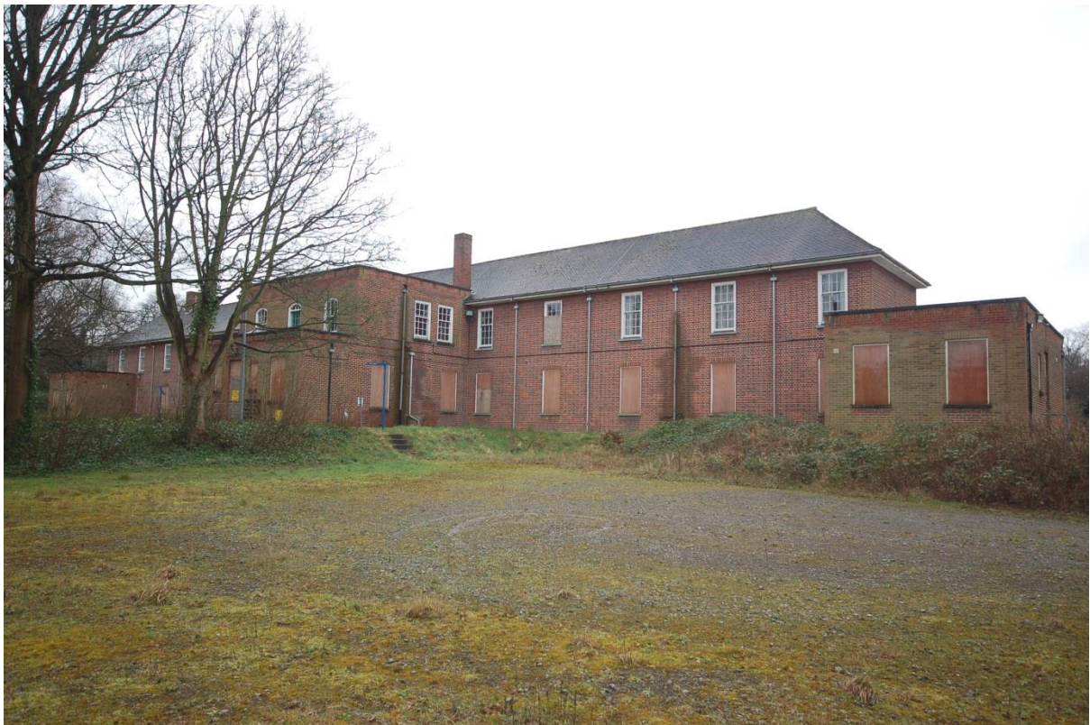
Plate 72: Building 3, rear, viewed to south
