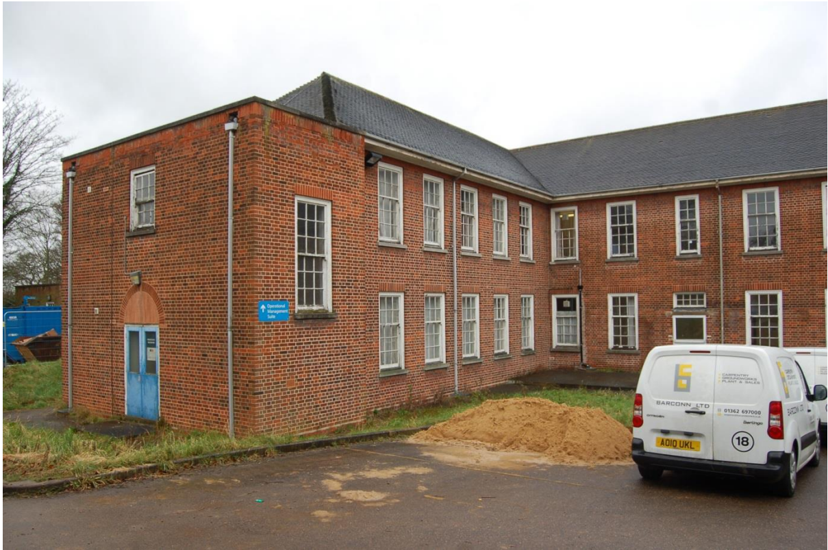
Plate 23: Building 2, dormitory block, viewed to northwest
