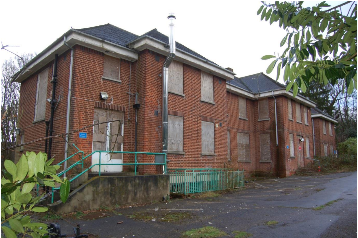
Plate 85: Building 4, viewed to northeast
