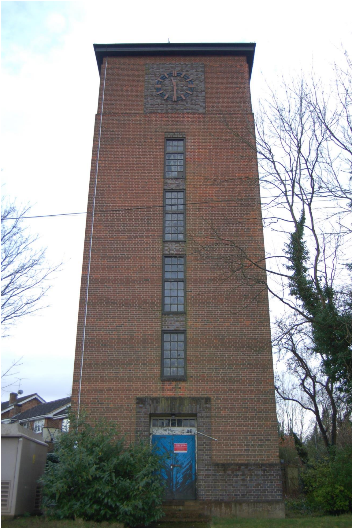
Plate 99: Building 5, northwest elevation
