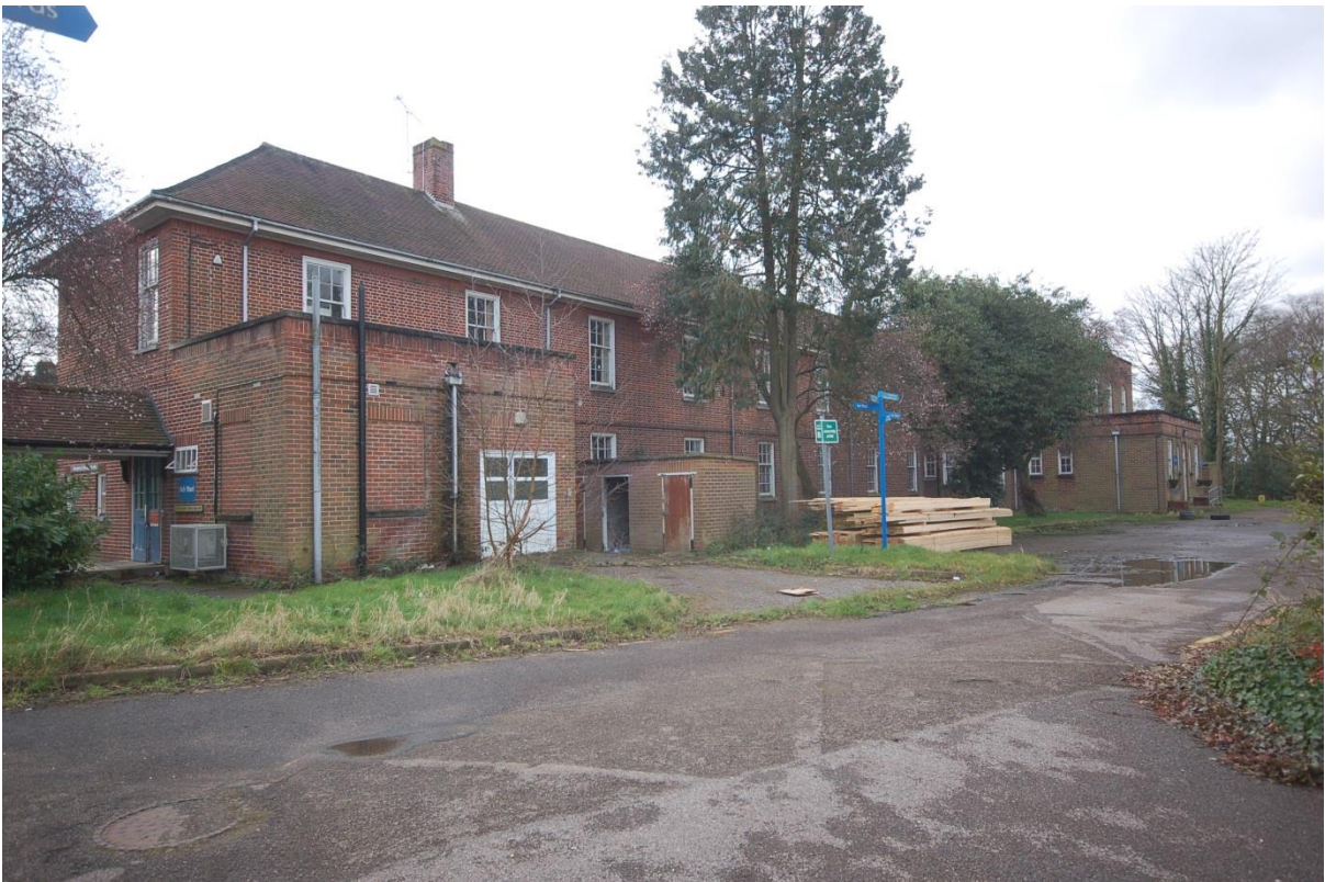
Plate 30: Building 2, viewed to southwest
