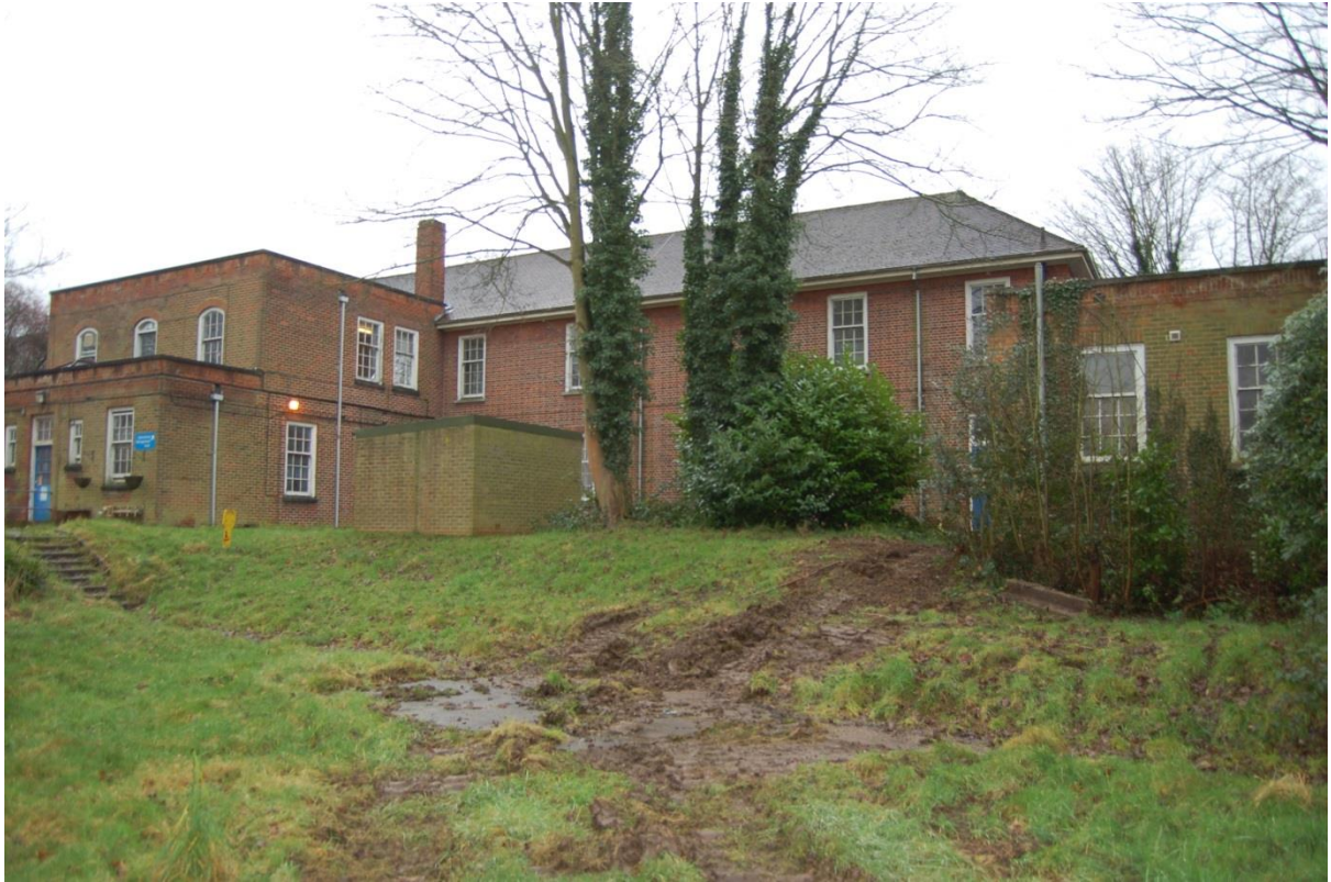
Plate 33: Building 2, viewed to southeast
