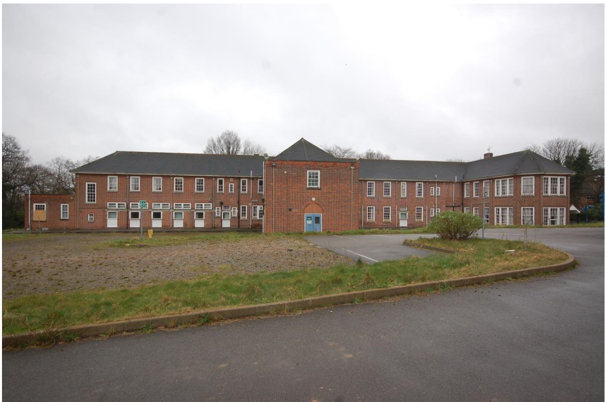
Plate 66: Building 3, viewed to northeast
