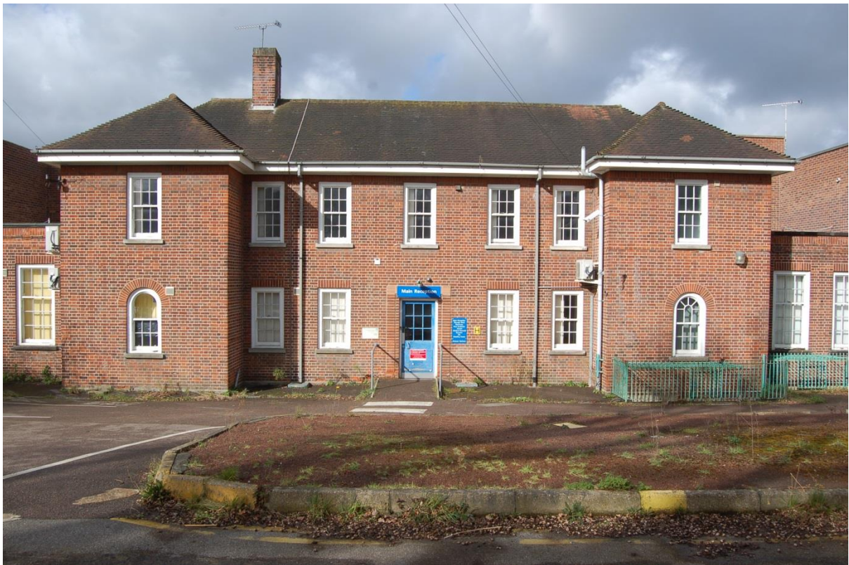
Plate 2: Building 1, Main Block
