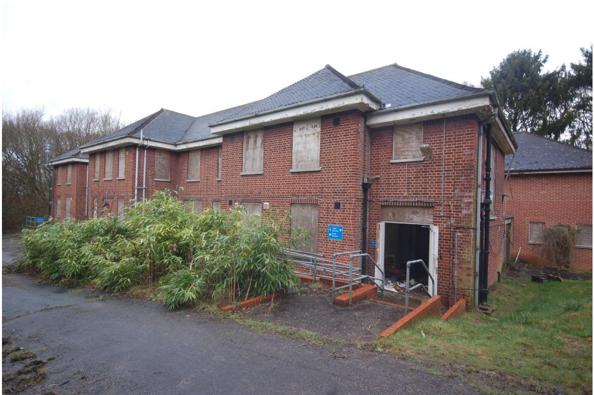
Plate 86: Building 4, viewed to northwest
