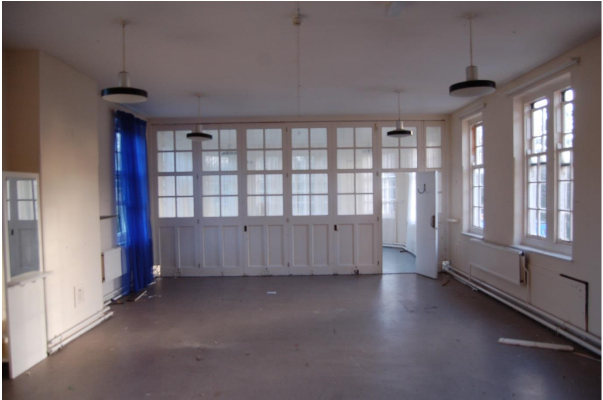
Plate 57: Room 7, viewed to south
