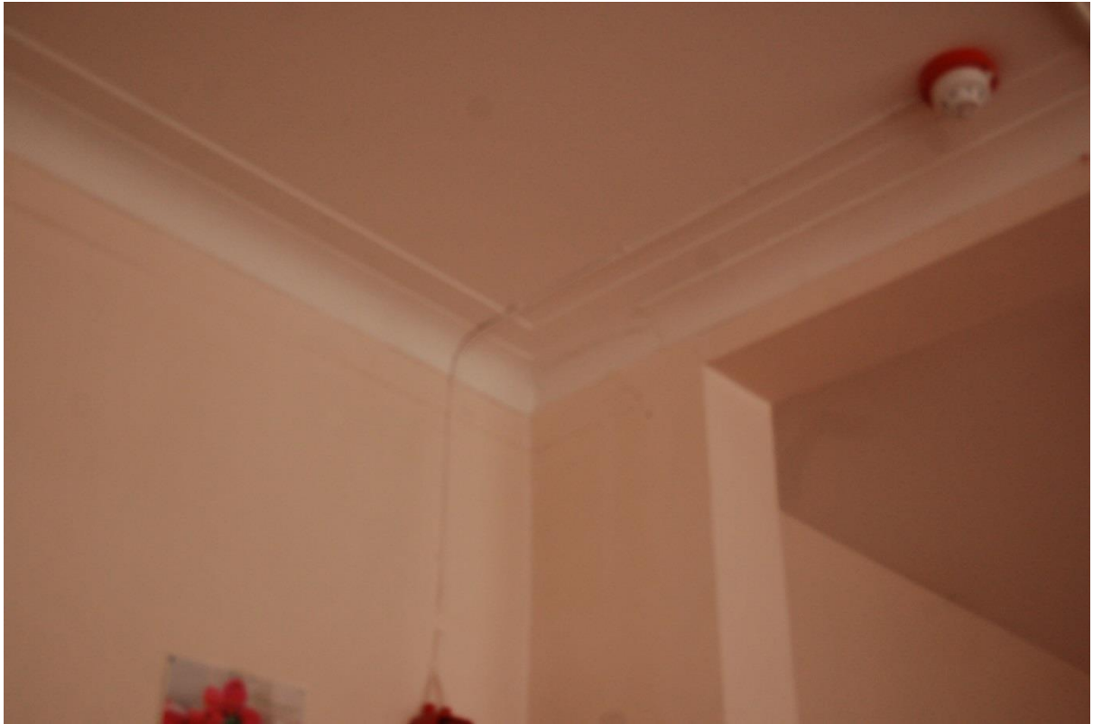
Plate 15: Room 14, ceiling detail
