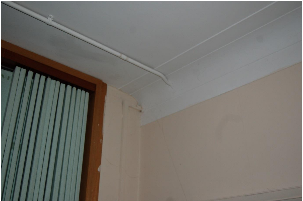
Plate 21: Room 8, ceiling detail
