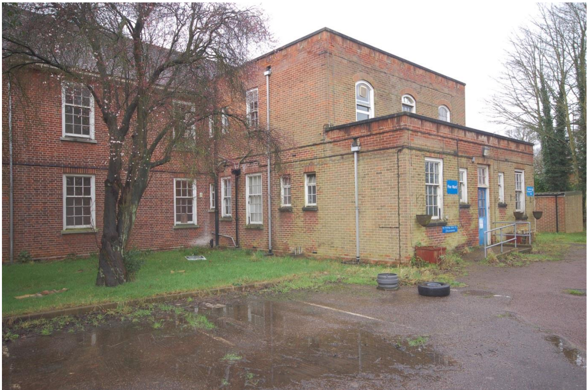
Plate 32: Building 2, central block, viewed to southwest
