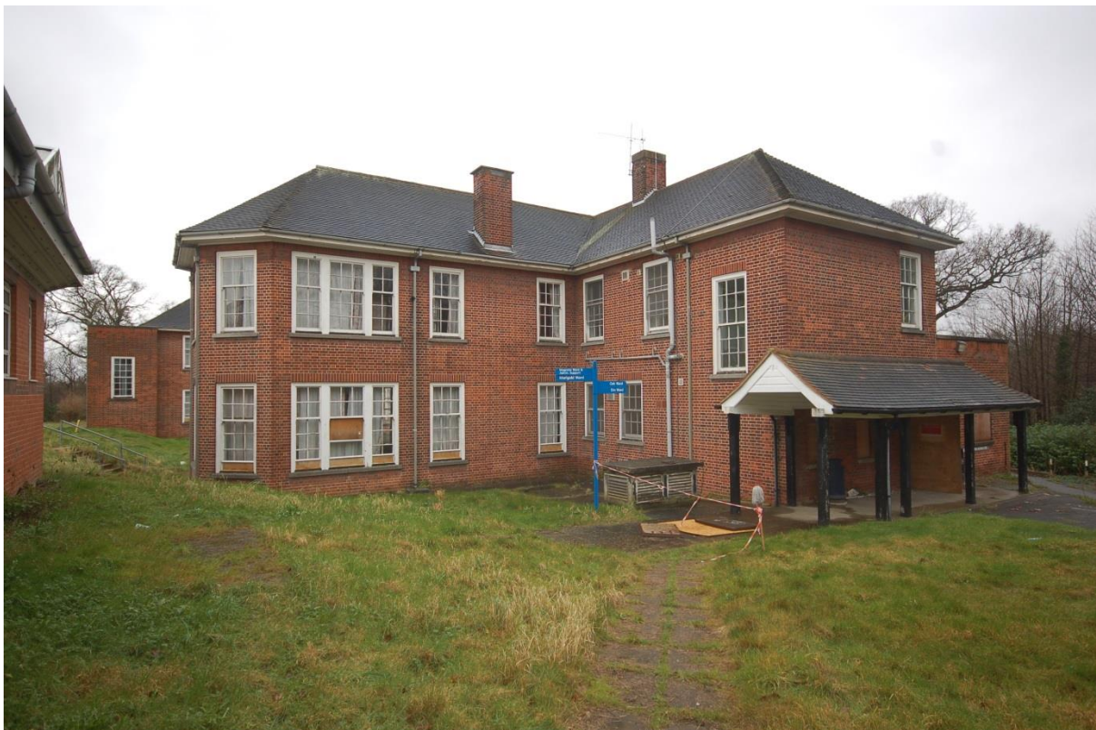
Plate 70: Building 3, southeast end, including covered passage remains
