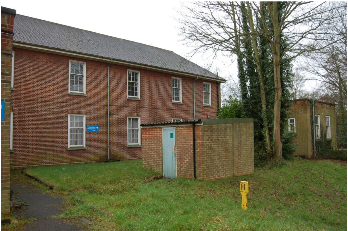
Plate 34: Building 2, west end, viewed to southwest
