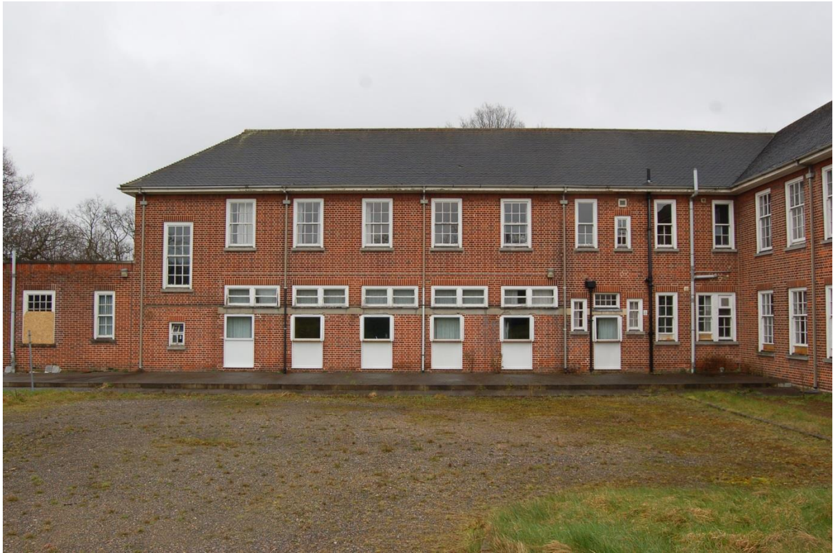
Plate 67: Building 3, northwest end, viewed to northeast
