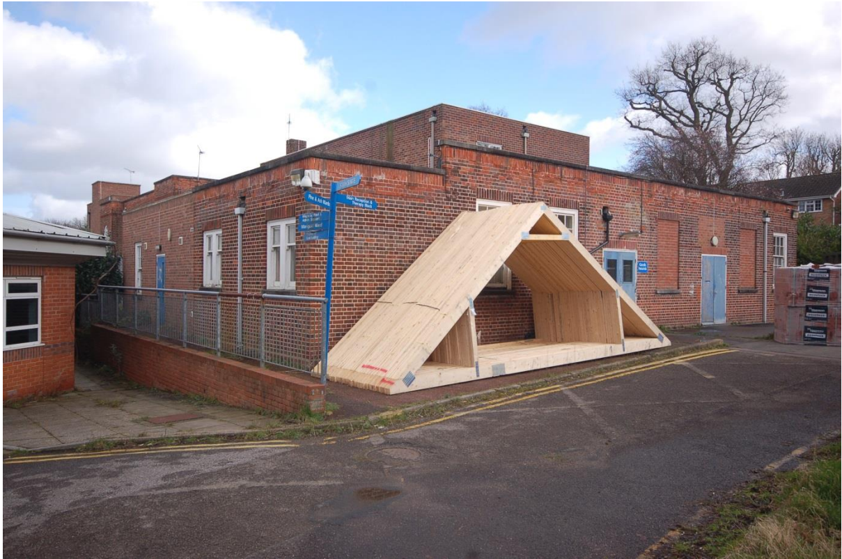
Plate 7: Building 1: viewed to northeast
