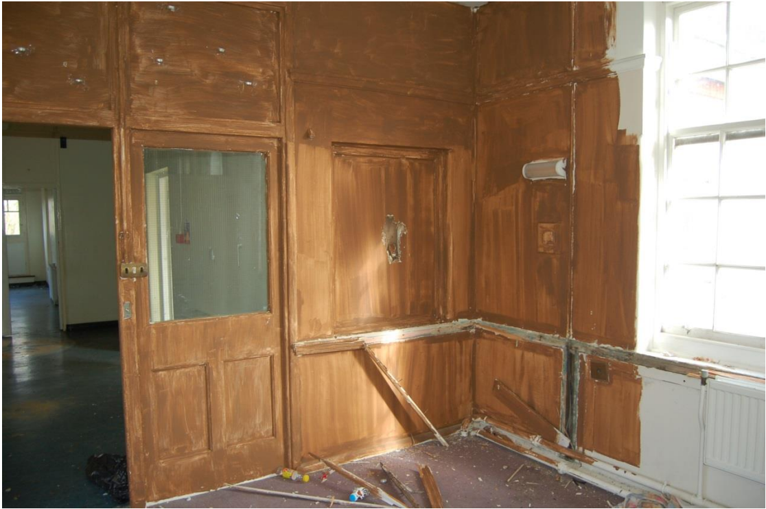
Plate 63, northeast corner of dormitory, including in-filled viewing window
