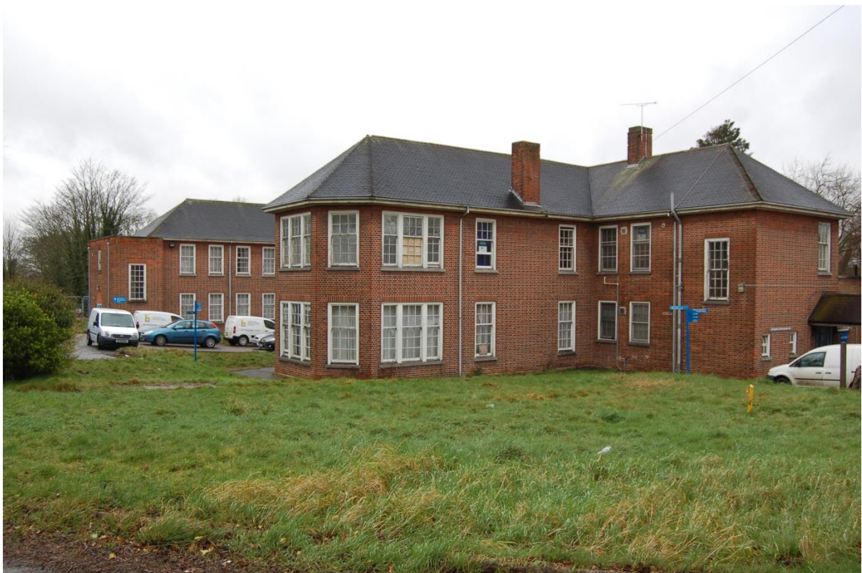
Plate 26: Building 2, viewed to northwest
