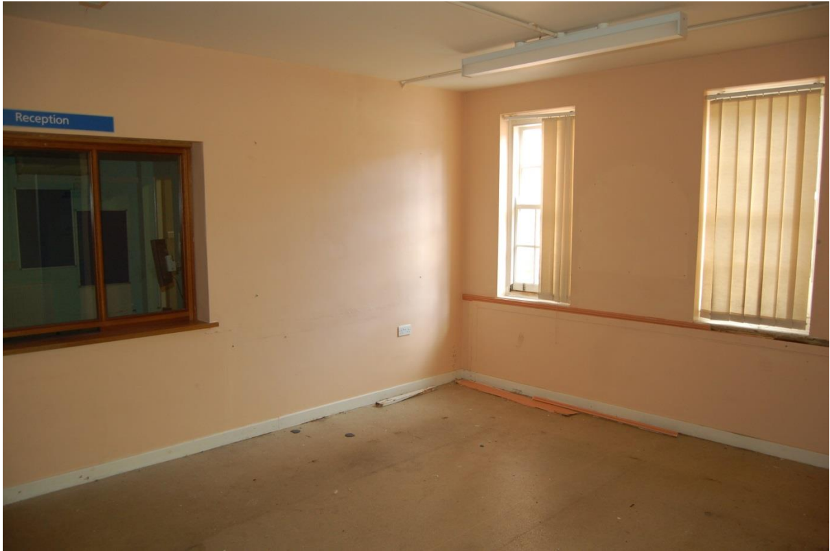
Plate 11: Room 2, with built-in radiator left
