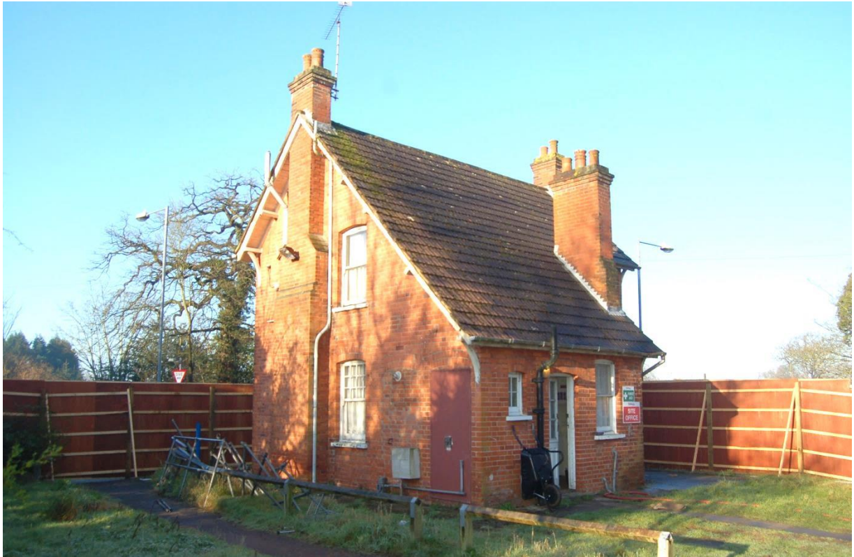
Plate 106: Building 6, viewed to southwest
