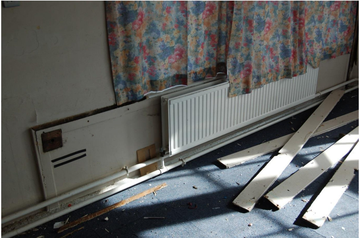
Plate 43: Room 14, radiator detail
