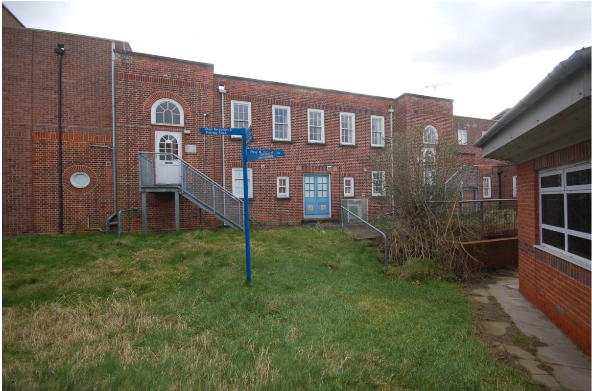
Plate 5: Building 1, rear of main block, viewed to southeast
